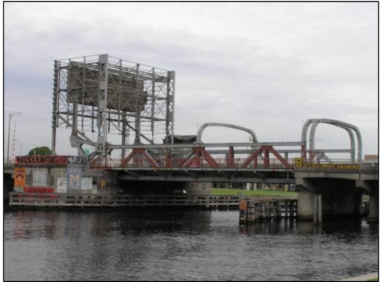
Photo 5-81. Laurel Street Bridge, Hillsborough County (No. 105503)
