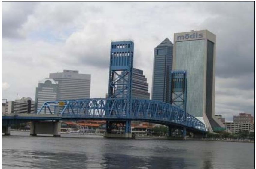
Photo 5-53. Main Street Vertical Lift Bridge, Duval County (No. 720022)
