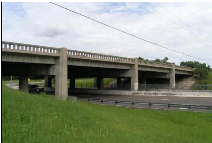
Photo 5-28. SR-109/University Avenue over SR-10A, Duval County (No. 720075)
