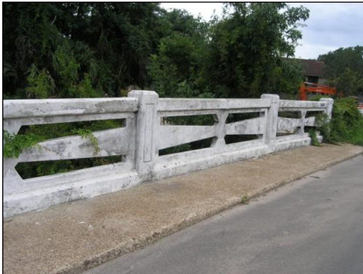
Photo 5-27. Myrtle Avenue Bridge, Duval County (No. 724258)
