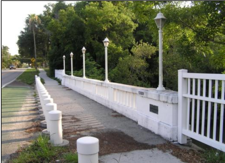
Photo 5-18. Philippe Parkway Bridge, Pinellas County (No. 150009)
