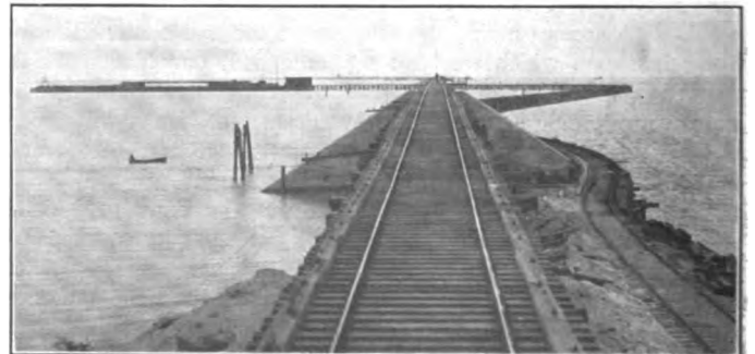
Temporary Dock and Approach at Knight's Key.
