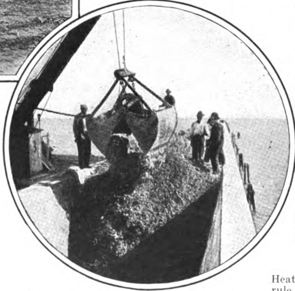
Filling in the concrete arches with sand
