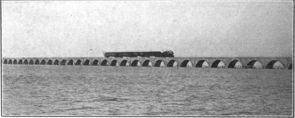
LONG KEY VIADUCT OF CONCRETE—2.7 MILES LONG
