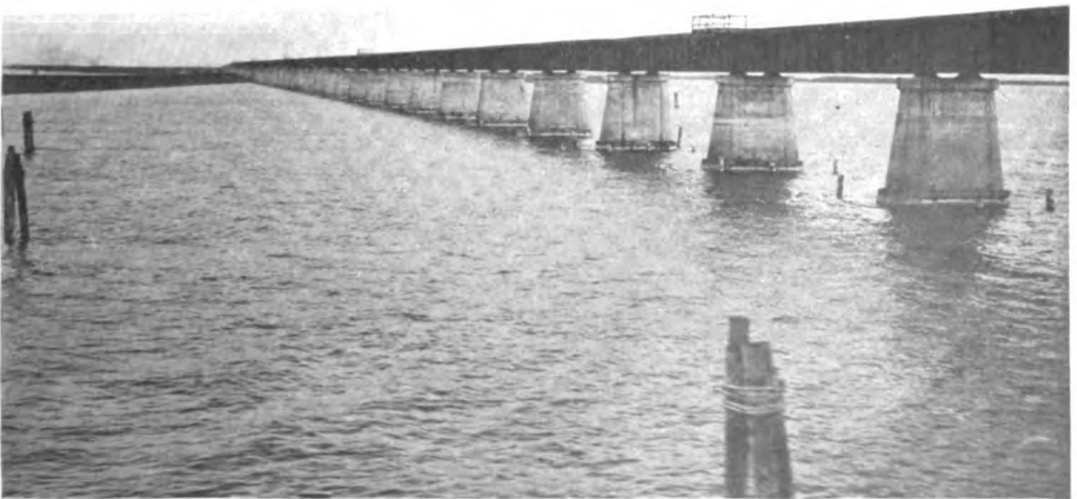
KNIGHTS KEY VIADUCT—THE SEA-GOING RAILROAD
