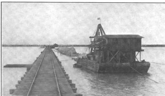
Gasolene Excavator Removing Washed Out Embankment, Preparatory to Building Concrete Arches.
