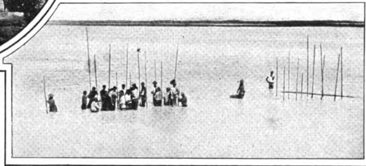
Drillers preparing submerged key for blasting
