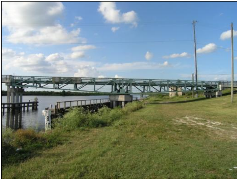
Photo 5-58. Belle Glade Swing Bridge, Palm Beach County (No. 930072)
