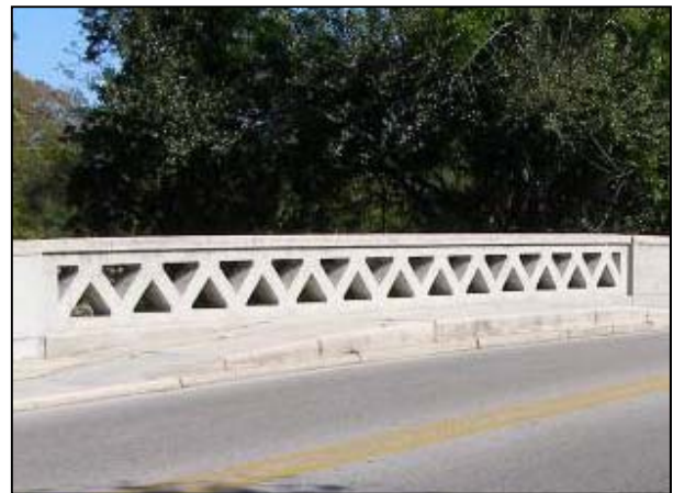
Photo 6-18. Zigzag Railing Detail on the Ninth Avenue Bridge.
