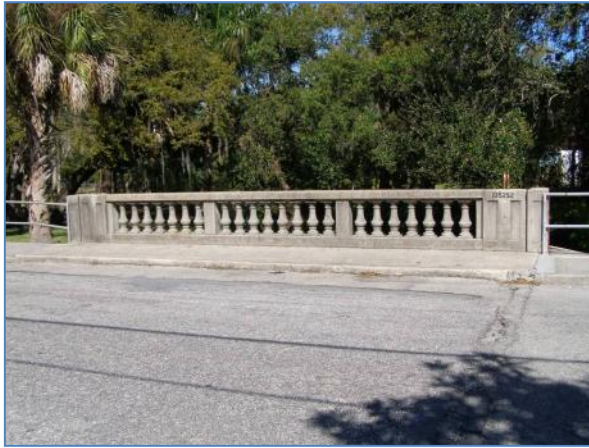
Photo 6-15. North Guardrail and Deck of the Twelfth Avenue Bridge (No. 135252)
