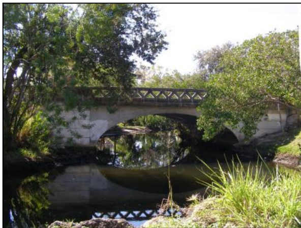
Photo 6-17. The Ninth Avenue Bridge (No. 135251), Looking Southwest.
