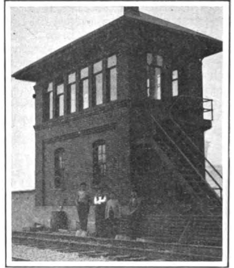
OPERATING TOWER AT THE BRIDGE
