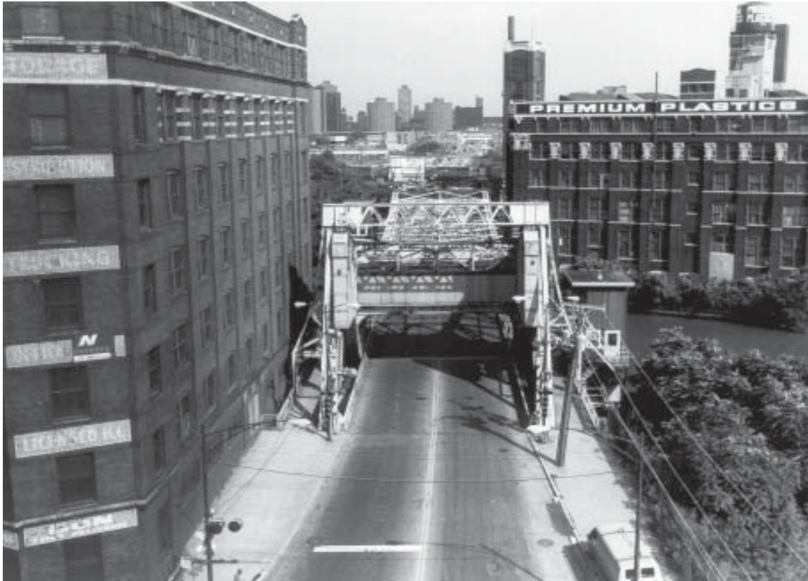
The Cermak Road Bridge District is the city's finest intact ensemble of riverfront industrial buildings grouped around the city's sole-surviving double leaf Scherzer Rolling Lift bridge. Above: A view of the Thomson & Taylor Spice Co. Building at 500 W. Cermak Rd. (left), the Cermak Road Bridge (center), and the Hoyt Building at 465 W. Cermak Rd. (right).
