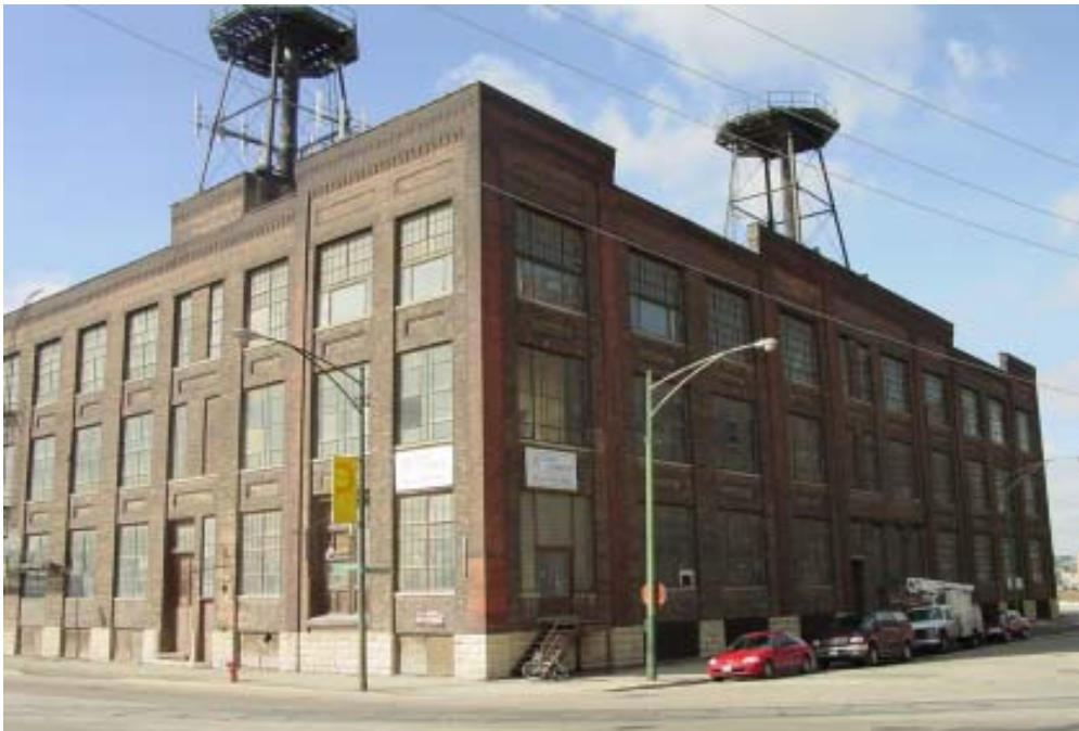
Bottom: The southeast portion of the Wendnagel Warehouse (left) was constructed in 1901. In 1906, the warehouse was expanded with six bays to the north.
