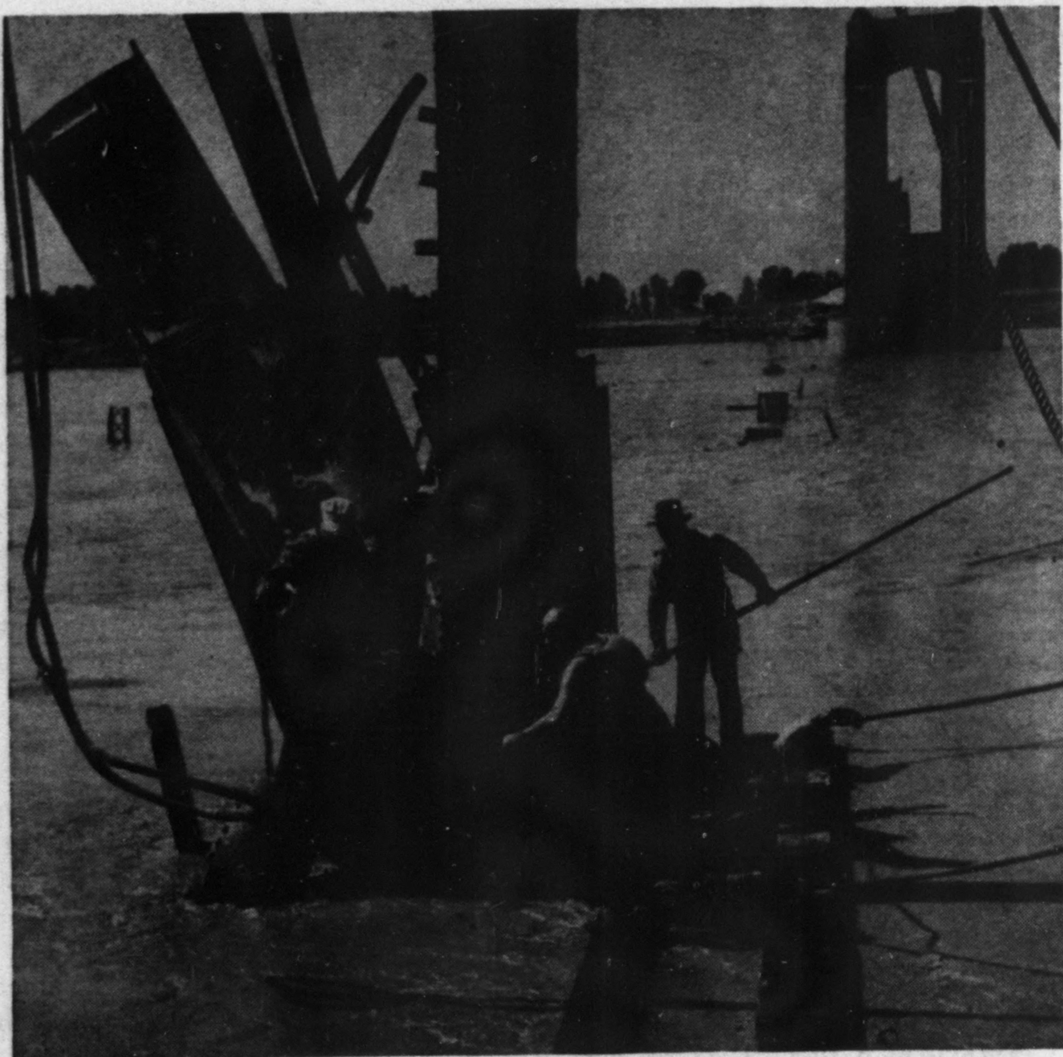
Some idea of the hazards of the work is shown in this action picture of workmen attaching slings preparatory to burning sections for removal.
