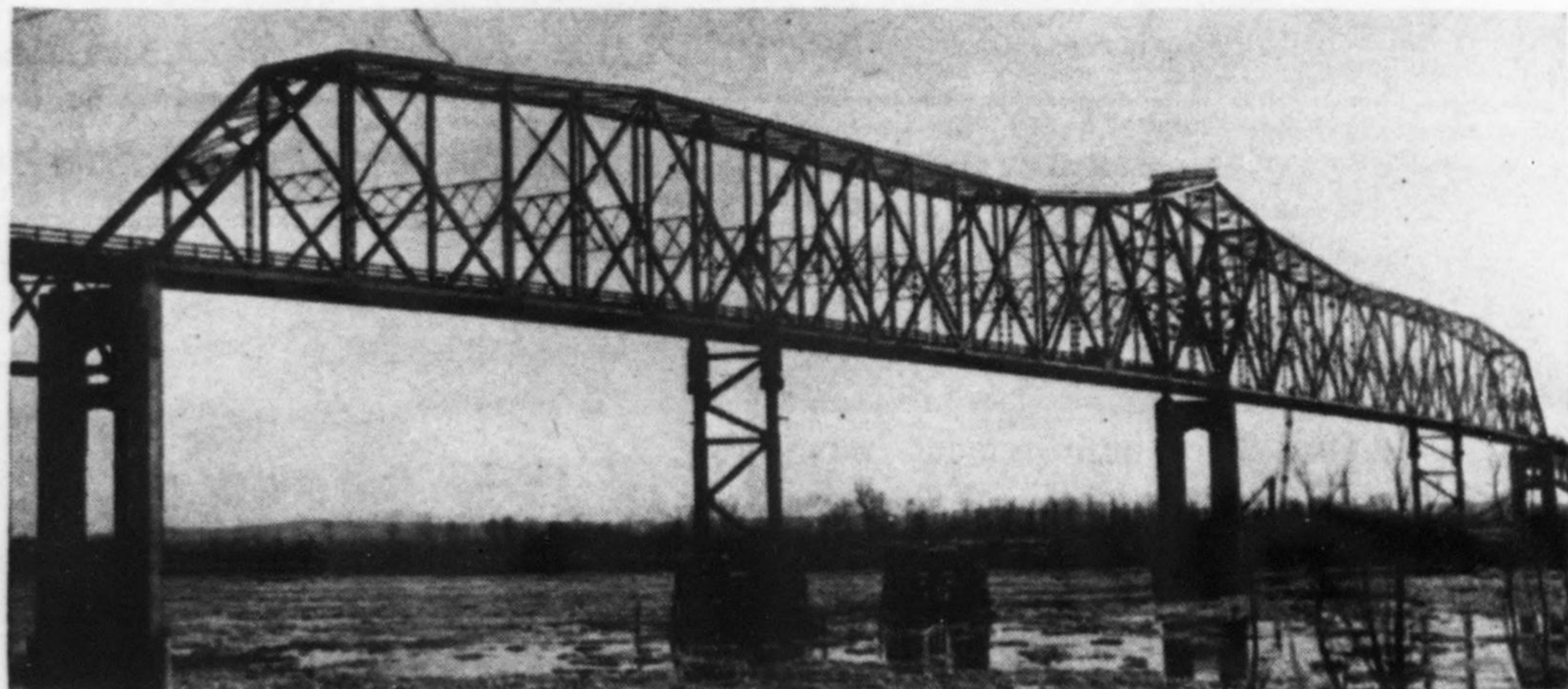
Two 670-ft. main spans fully erected. One falsework bent in each span is holding camber until riveting can be completed.
