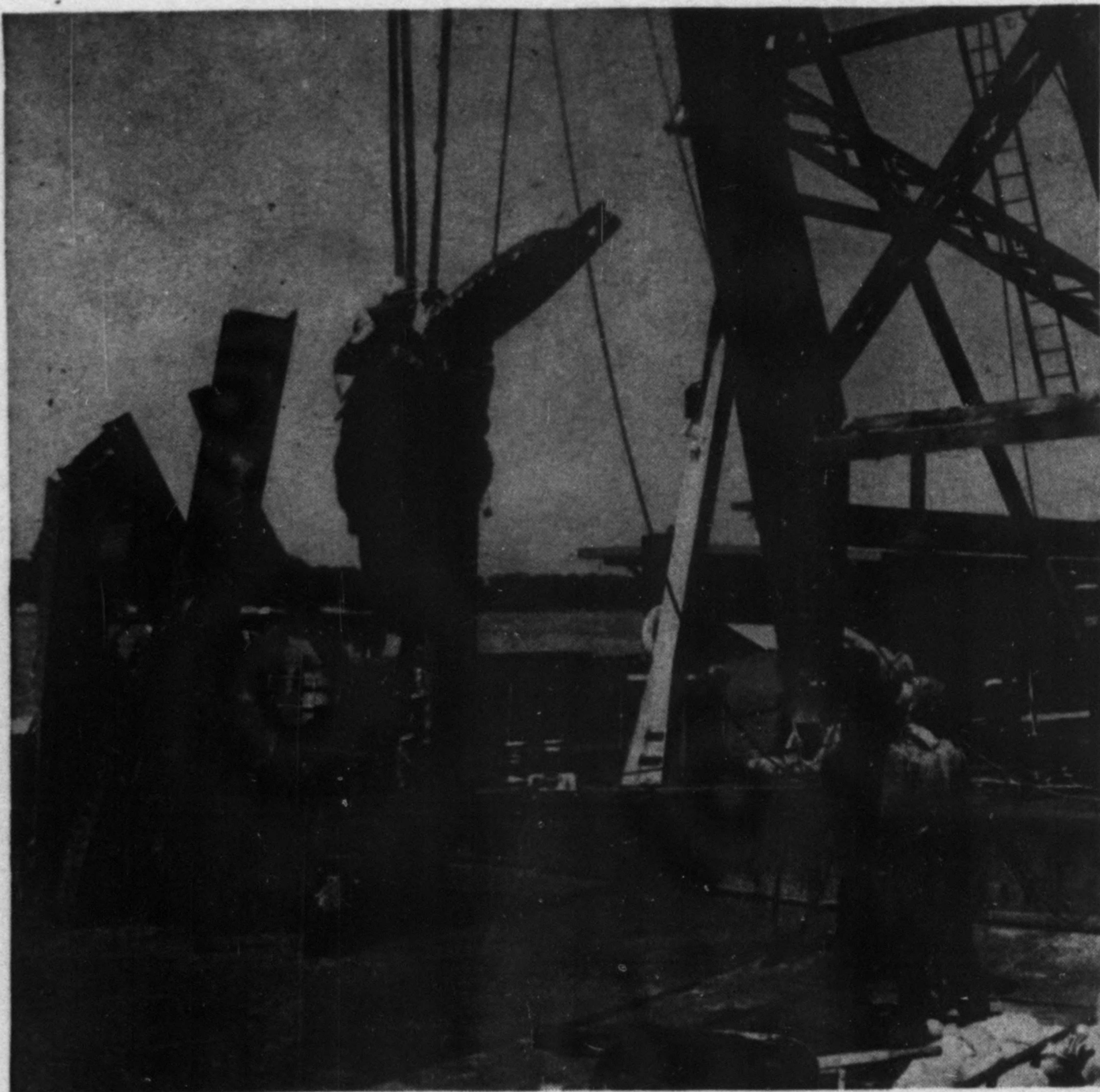
After a twisted mass of dynamited steel was raised above the river, members were burned into convenient lengths for loading onto barges.
