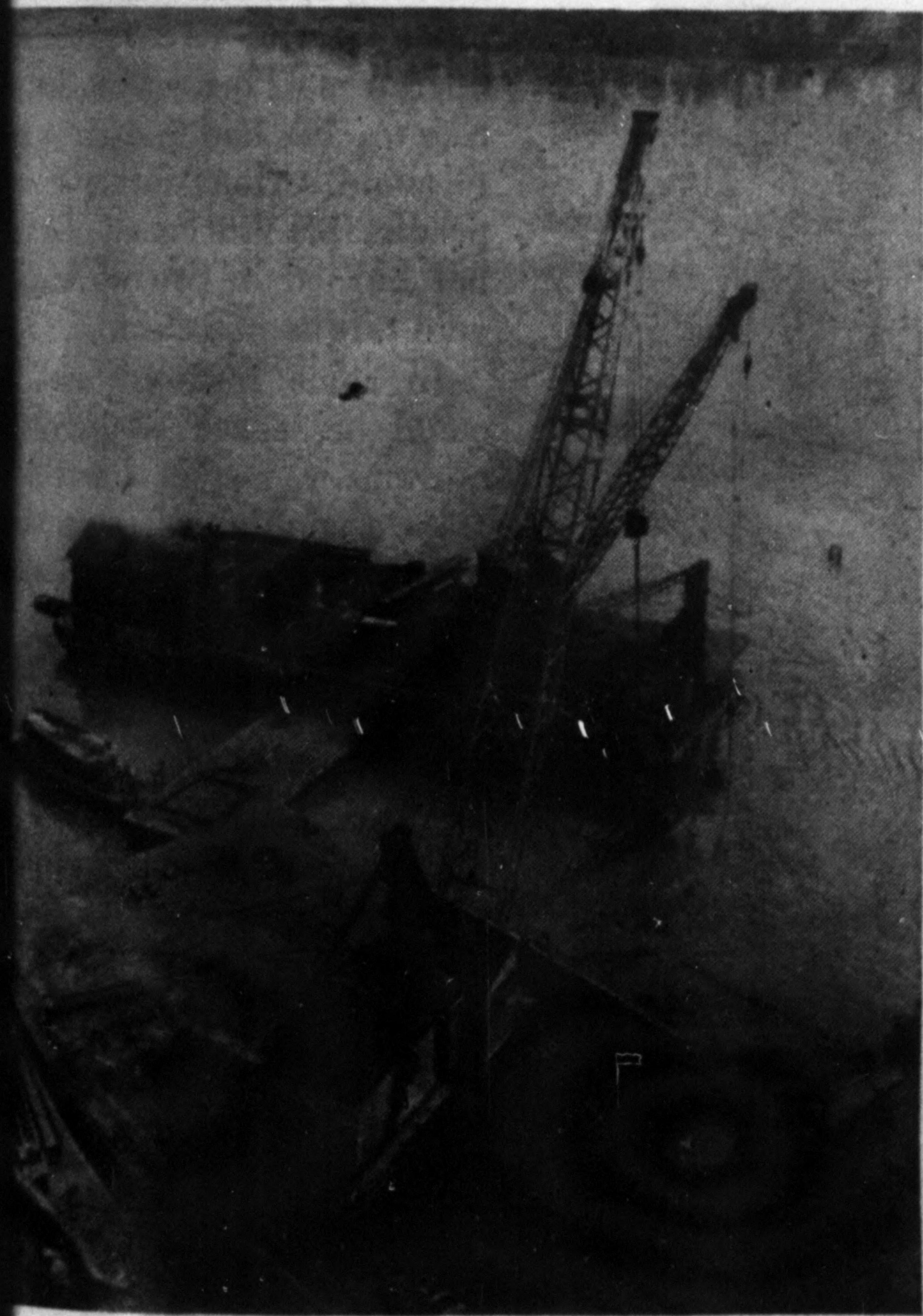
Salvaged steel was loaded on barges by a revolving crane and a crawler crane (left) while the U. S. Army Engineer derrick (right) moved out over the bottom truss chords to do the heavy lifting.
