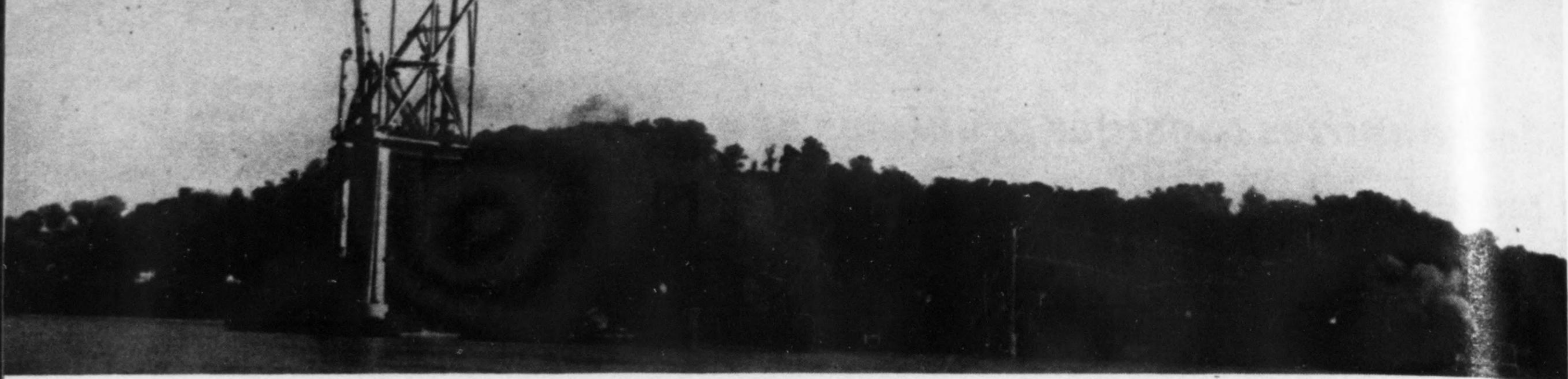
Erection of two main spans by two derricks operating in opposite directions from mid-river pier.
