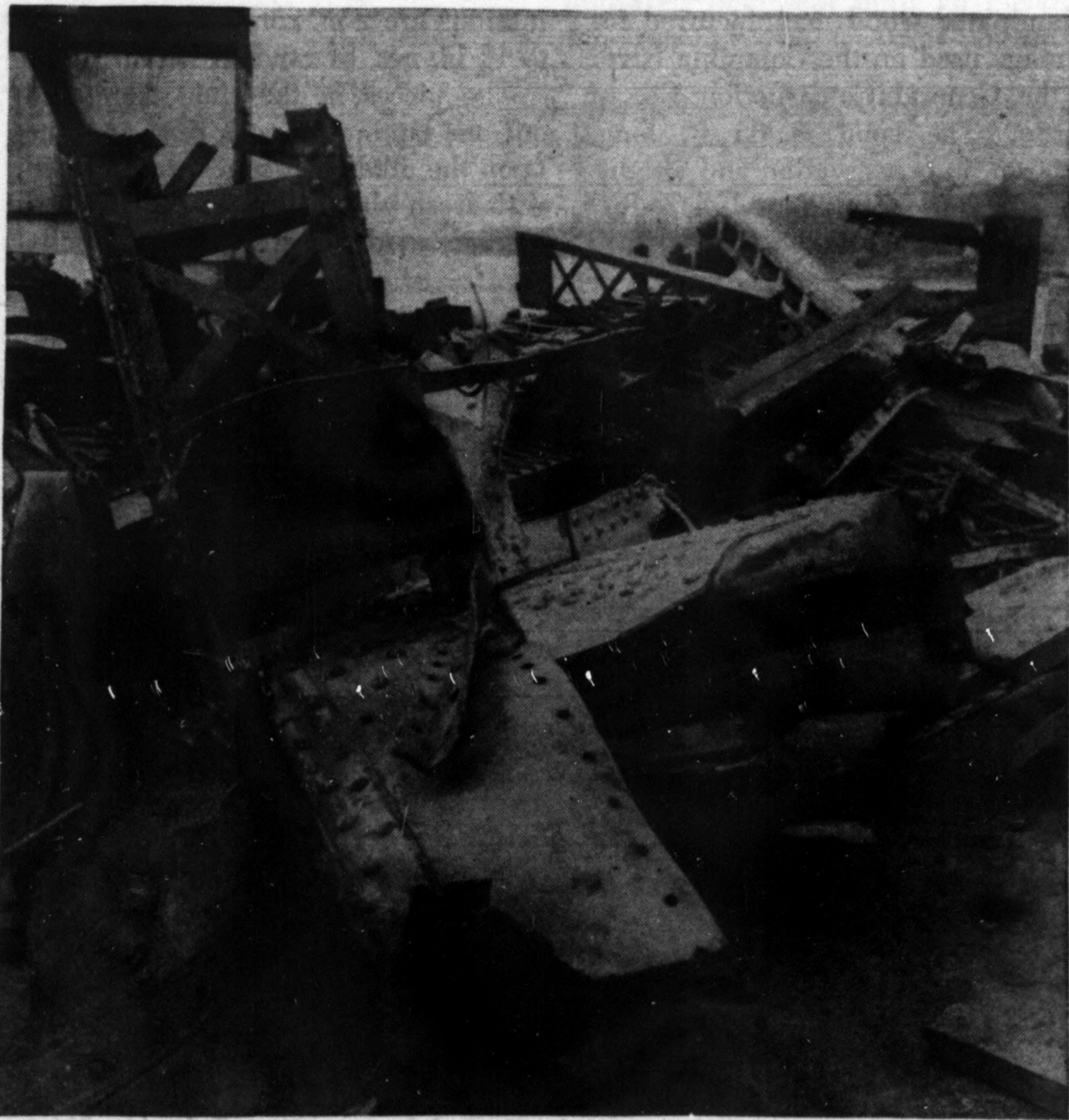
A close-up of a truss joint shows the effect of marine dynamiting.
