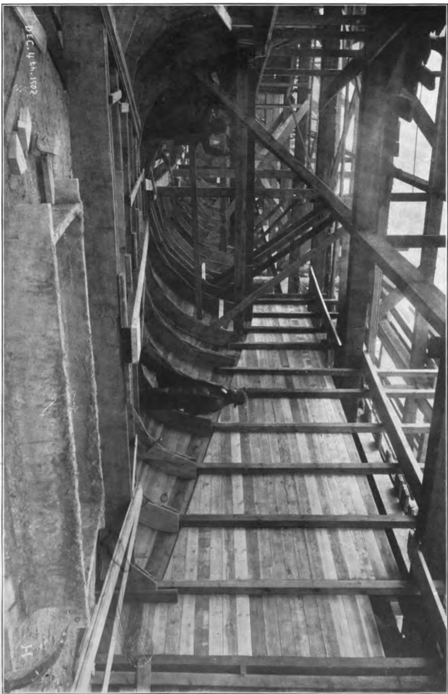
NO. 5. FORM FOR BOTTOM AND WALL, ONE OF MAIN CHANNELS, THIRTY-NINTH STREET PUMPING STATION — DECEMBER 4, 1903.
