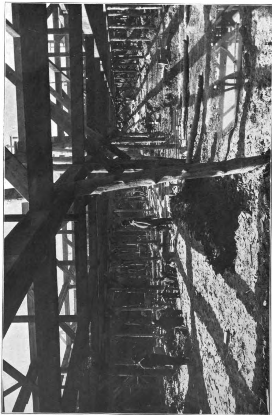
NO. 3. EXCAVATING IN COFFER-DAM, THIRTY-NINTH STREET PUMPING STATION, BELOW DREDGED LINE — SEPTEMBER 26, 1903.
