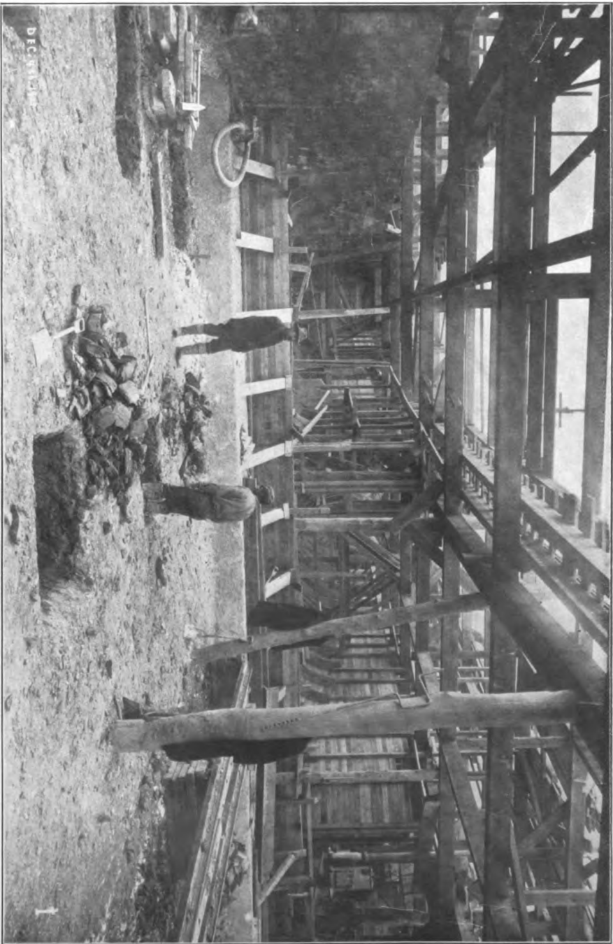
NO. 4. CONCRETE FLOOR AND WALL IN COFFER-DAM, THIRTY-NINTH STREET PUMPING STATION, AND FORMS FOR CONTINUATION — DECEMBER 4, 1903.
