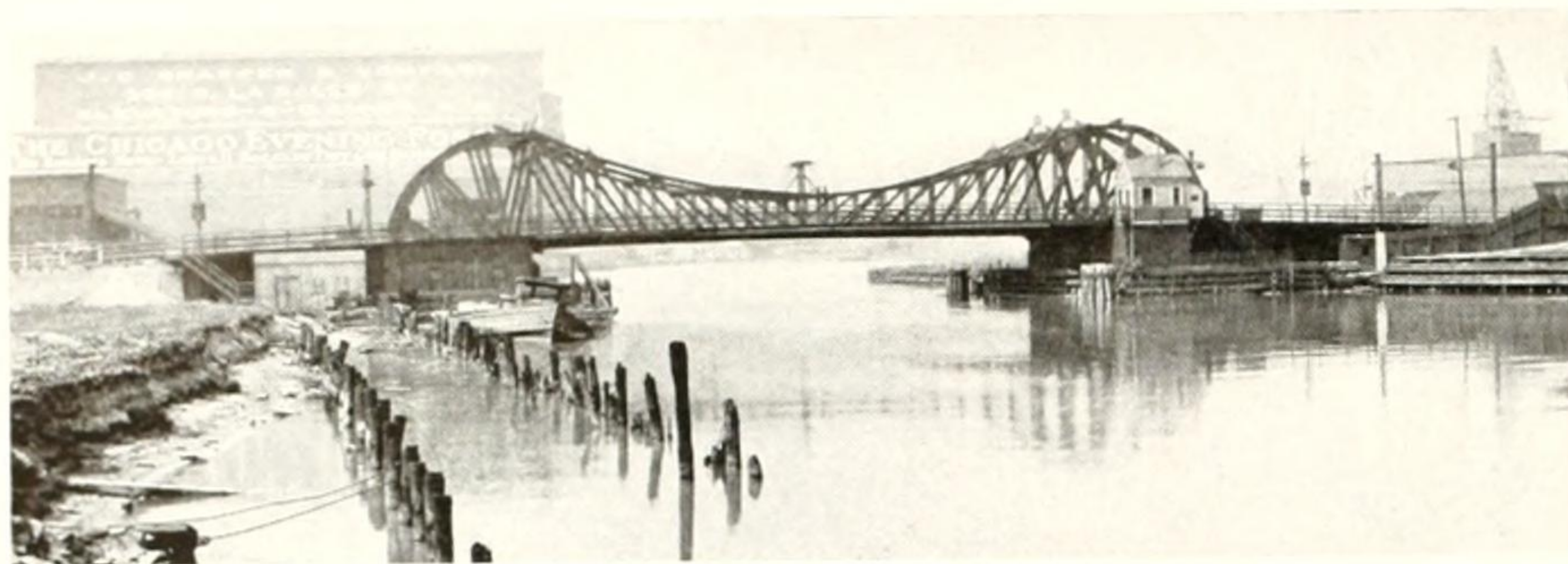
Ninety-Fifth Street Bridge: 1905. 3-Truss, External-Rack Trunnion Bascule.
