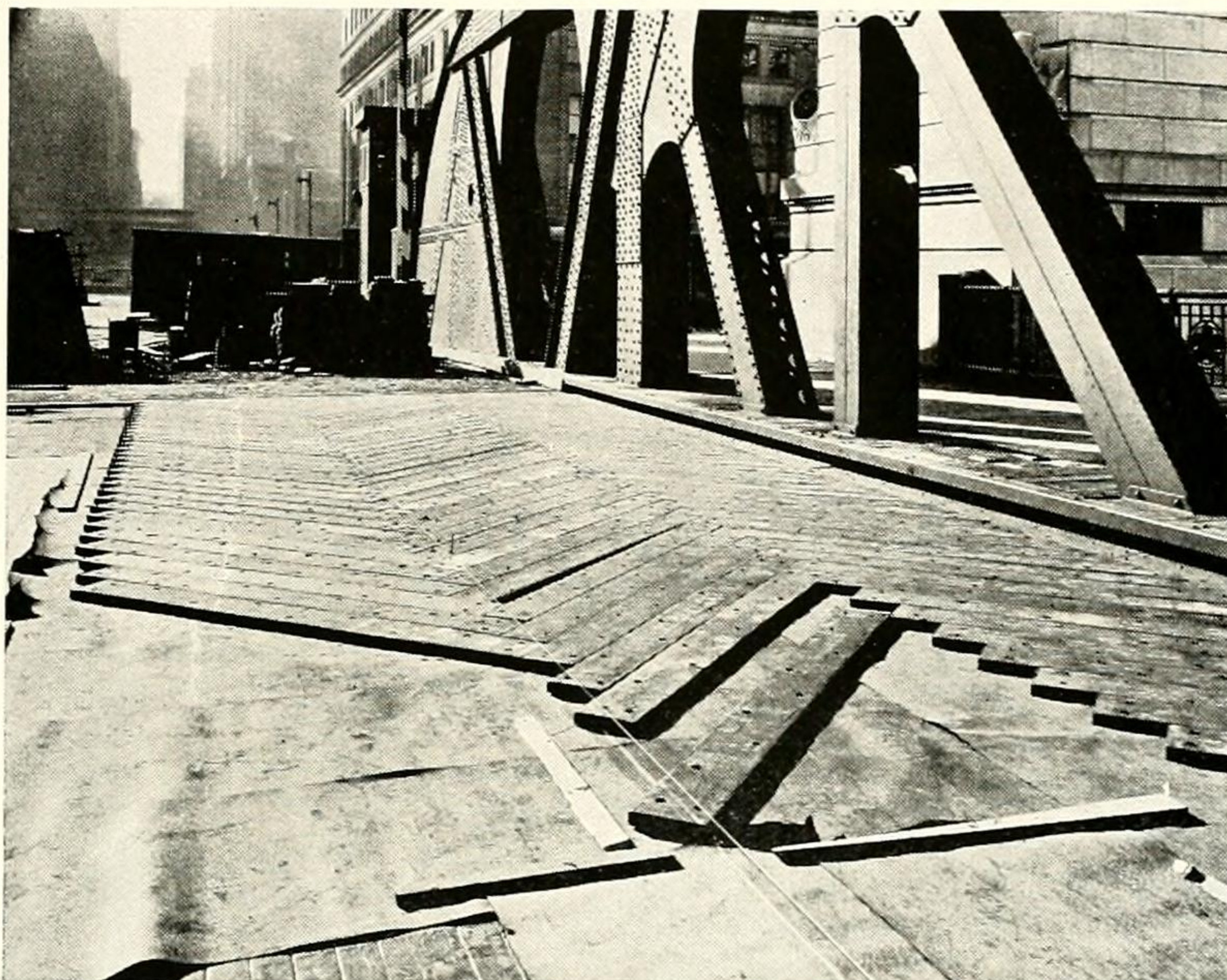
New types of bridge covering have been developed since the advent of heavy automobile traffic. This particular kind is made up of asphalt planks laid diagonally.
