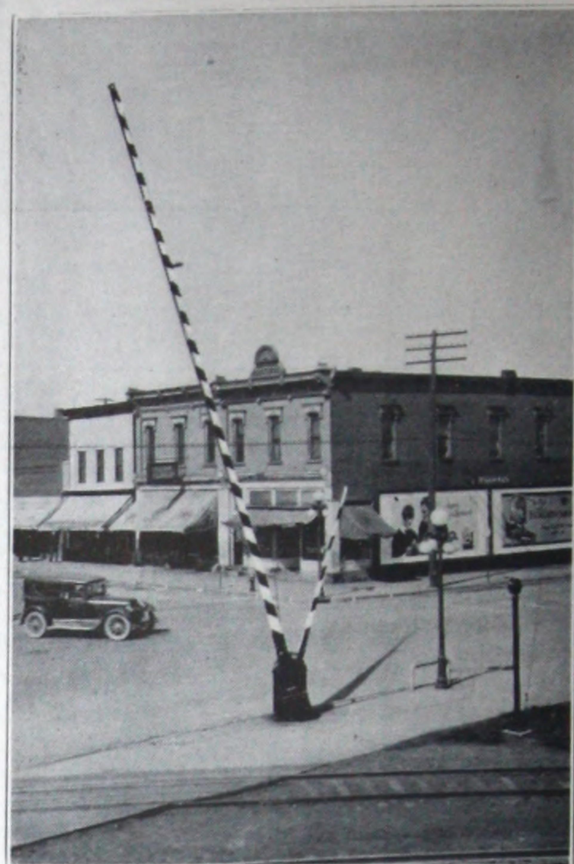
MODEL N-N-13 INSTALLATION 48-FT. ARM, 75^\circ TRAVEL
