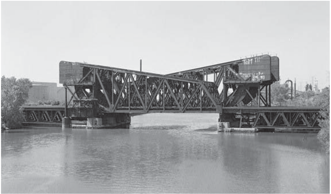
The Pennsylvania Railroad “Eight-Track” Bridge is significant for being the last Scherzer Rolling-Lift Bridge erected in Chicago for railroad use. The bridge encompasses four side-by-side bridges (bottom right). The counterweights are situated on alternating ends of each span (bottom left).
