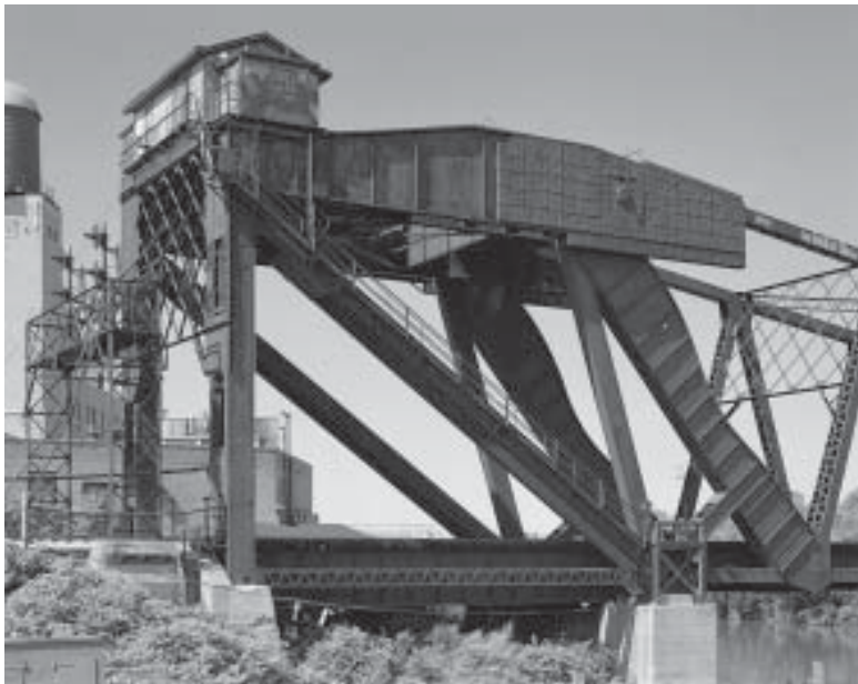
The Chicago & Alton Railway Bridge is an example of the Page trunnion bascule-type bridge. The single-leaf structure spans the South Branch of the Chicago River.
