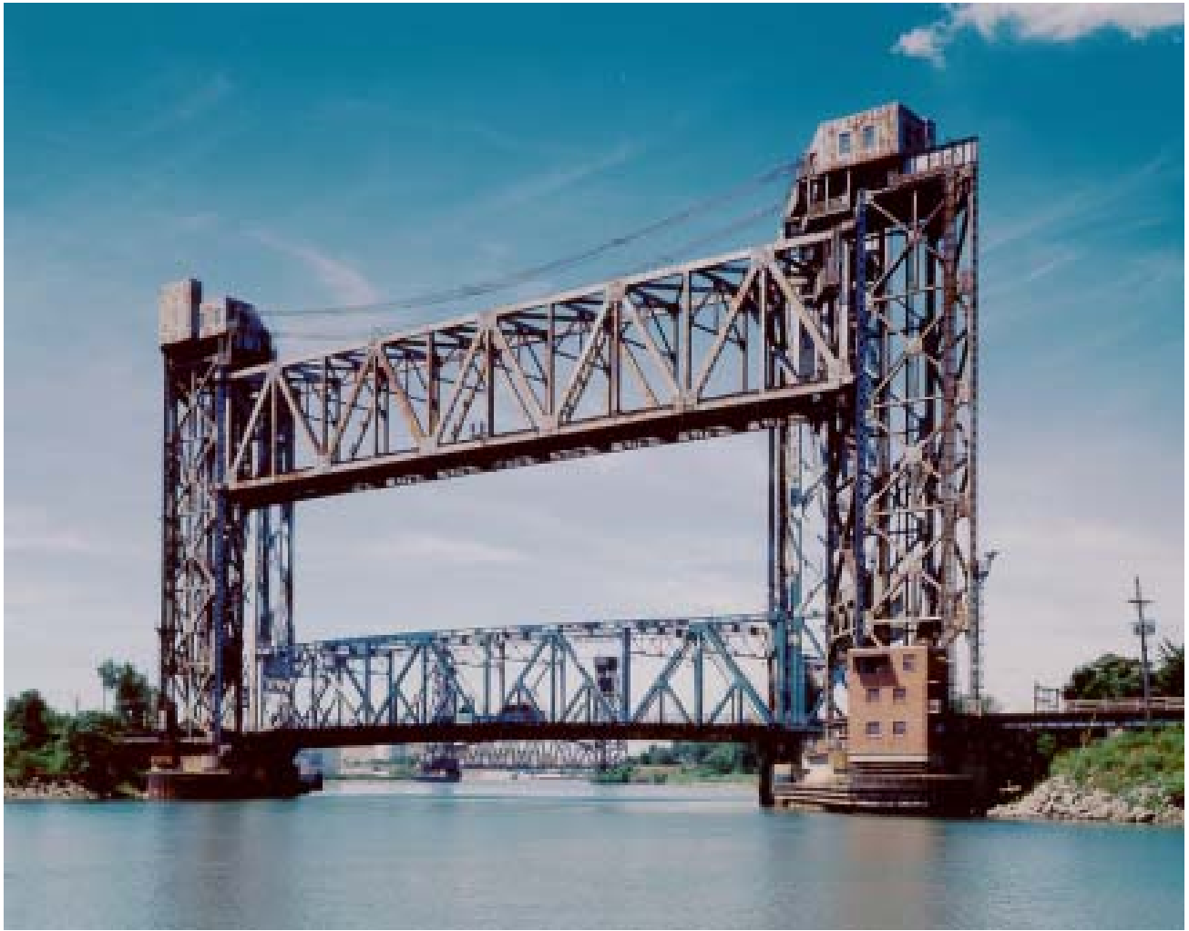
Top: The Chicago & Western Indiana Railroad Bridge is an outstanding example of a “tower-driven” vertical-lift bridge. Left: The span was designed to be raised and lowered by a system of giant pulleys and cables.
