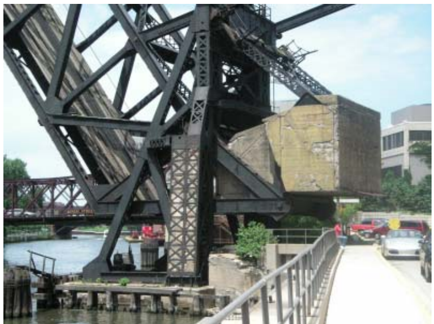
Left: The Chicago & Northwestern Railway Bridge on the North Branch of the Chicago River is an excellent early example of an overhead-counterweight bascule bridge based on the patents of prominent Chicago bridge designer Joseph Strauss. Bottom: The bridge's massive concrete counterweight weights over 1,200 tons.
