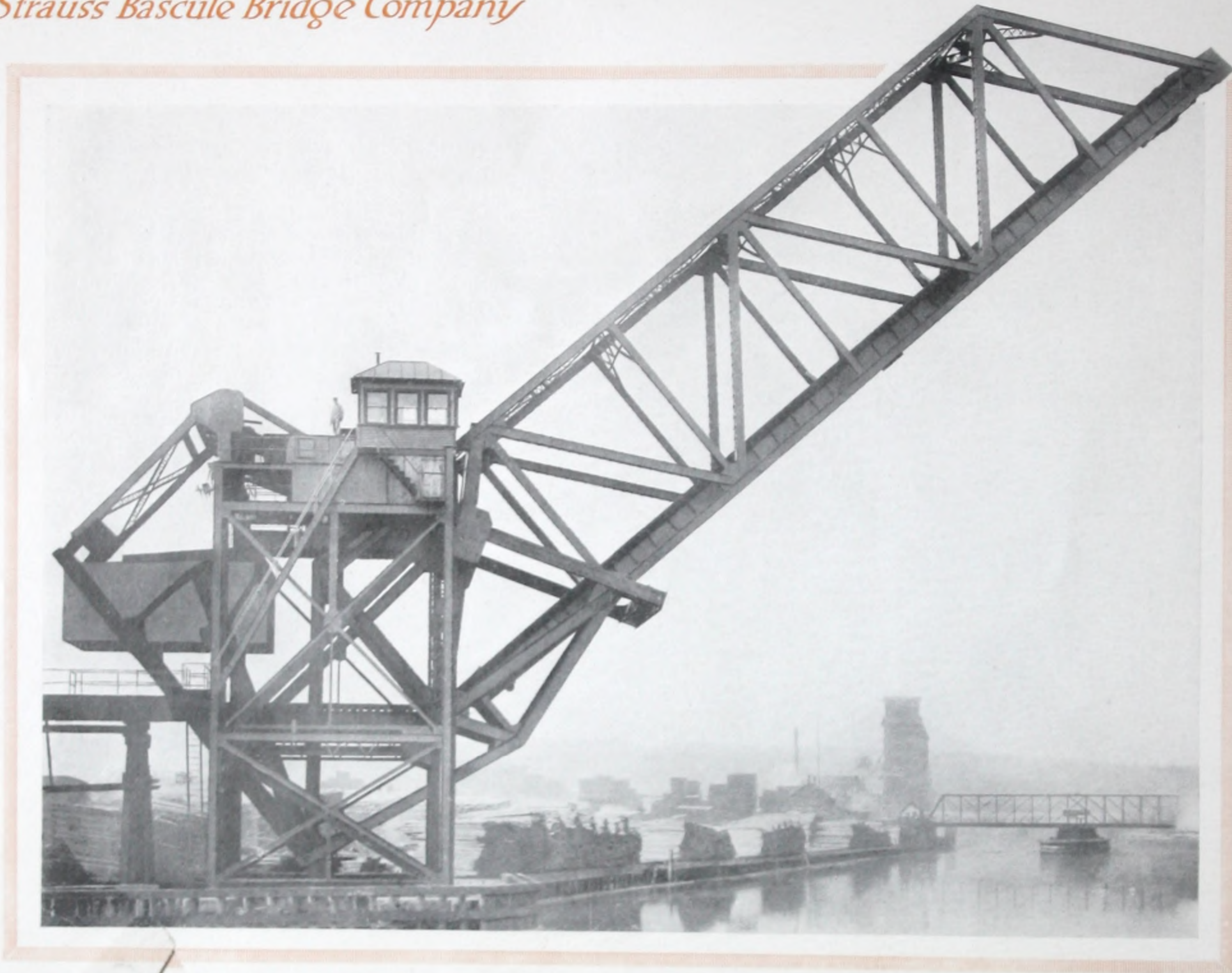
FIGURE 1. WHEELING & LAKE ERIE R. R. SINGLE TRACK BRIDGE OVER CUYAHOGA RIVER, CLEVELAND, OHIO Length of span 150 feet. Completed, 1905. First Strauss Bascule Built
