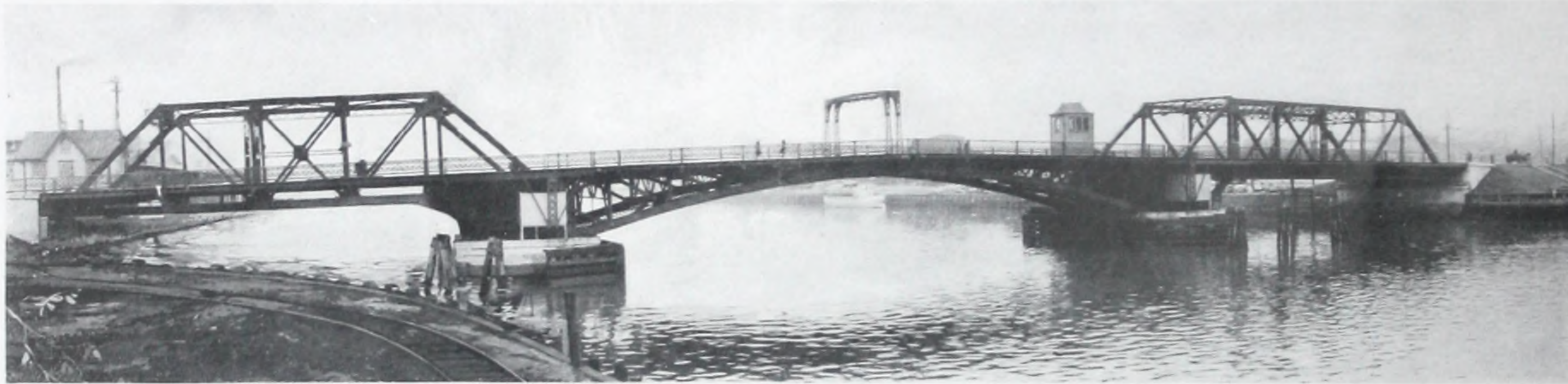
FIGURE 15. DOUBLE LEAF UNDERNEATH COUNTERWEIGHT HIGHWAY BRIDGE, THIRD STREET OVER CHRISTIANA RIVER, WILMINGTON, DELAWARE
