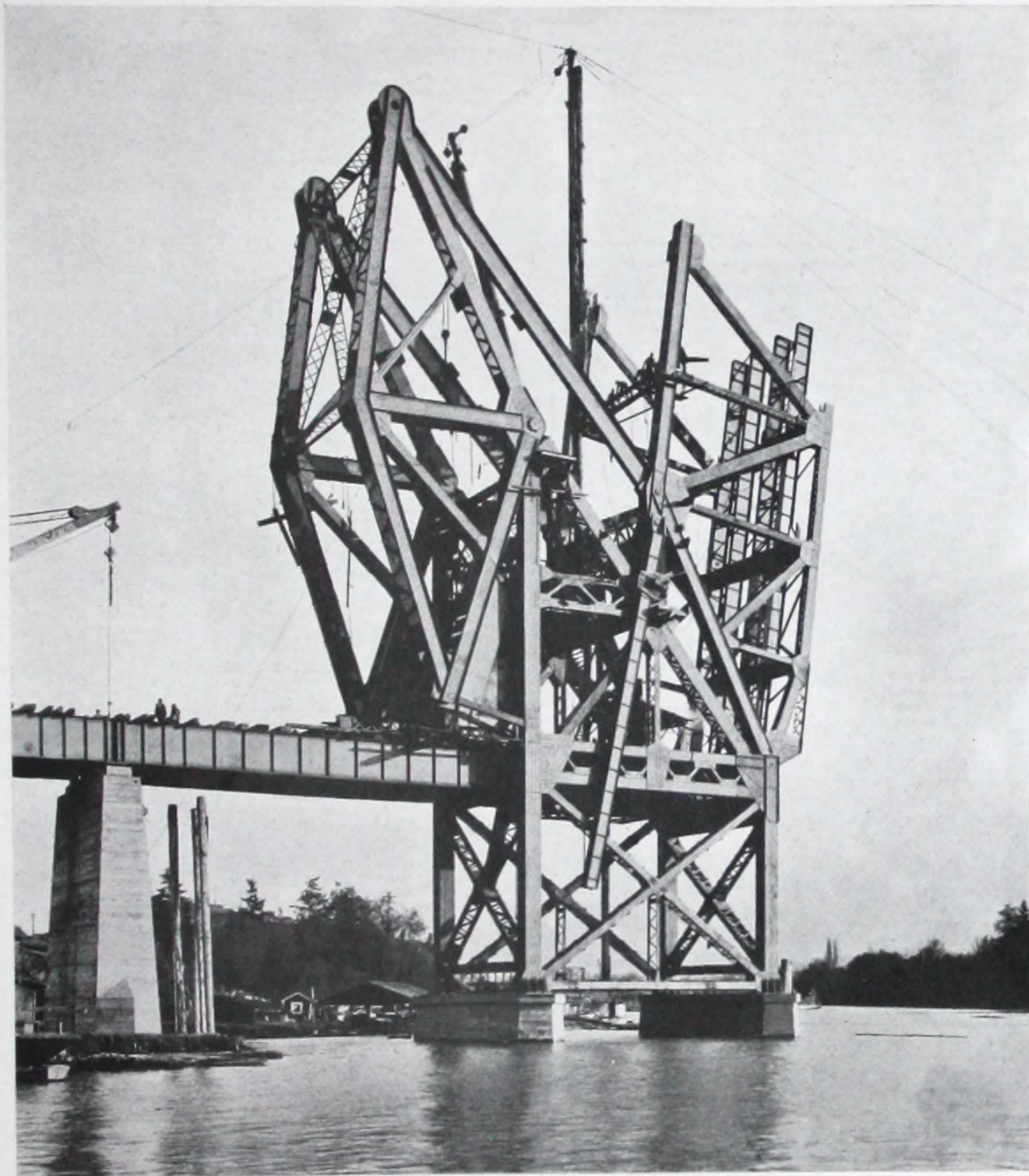
FIGURE 25. ERECTION VIEW GREAT NORTHERN RAILWAY BRIDGE OVER ENTRANCE TO LAKE WASHINGTON CANAL, SEATTLE, WASHINGTON
