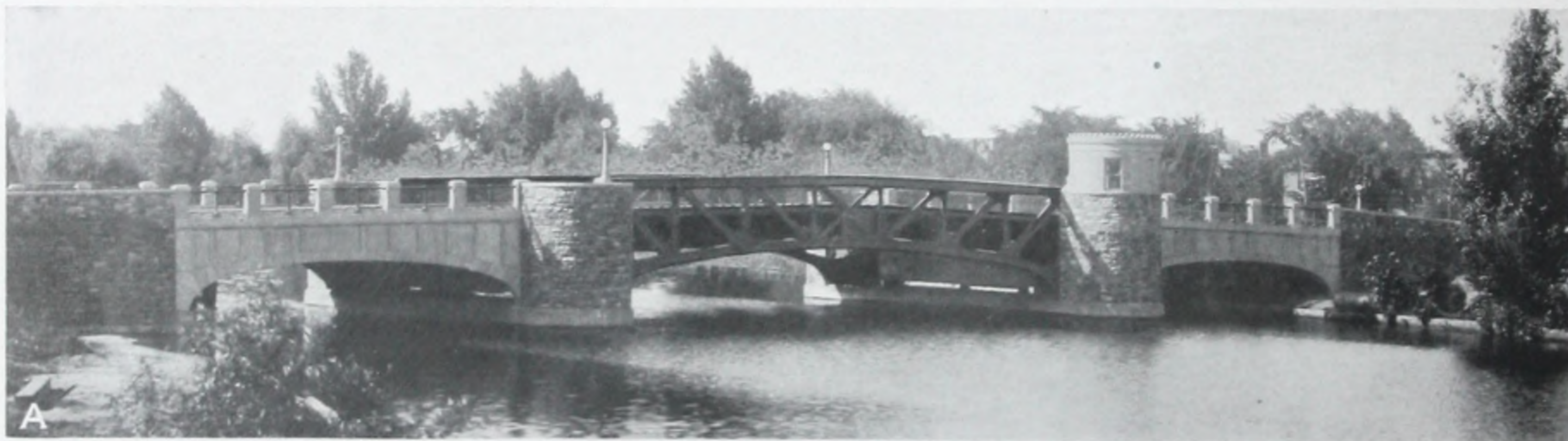
FIGURE 18. DIRECT LIFT HIGHWAY BRIDGE. COUNTERWEIGHTS BENEATH ROADWAY OVER RIDEAU CANAL AT PRETORIA AVENUE, OTTAWA, CANADA
