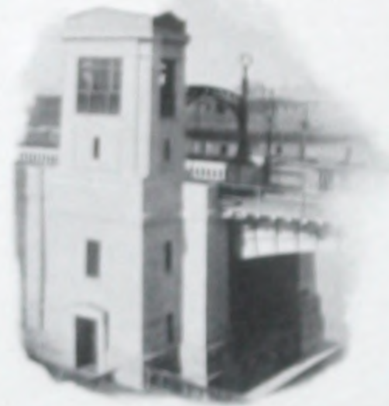
OPERATORS' HOUSE, CHARLES RIVER BRIDGE, BOSTON ELEVATED RY.
