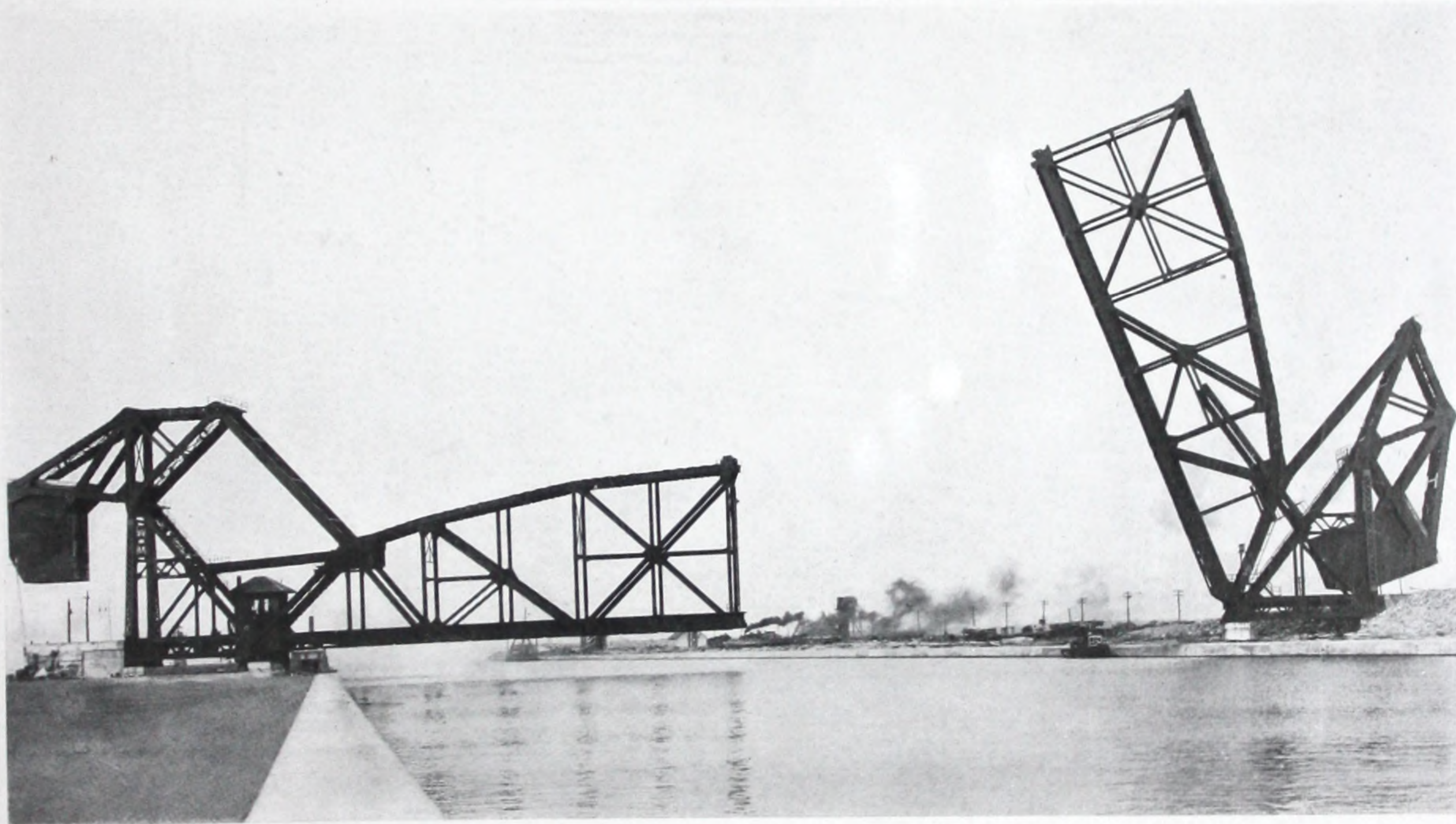
FIGURE 24. DOUBLE LEAF HEEL TRUNNION BRIDGE, CANADIAN PACIFIC RAILWAY (SINGLE SPAN DESIGN) OVER NEW U. S. SHIP CANAL, SAULT STE. MARIE, MICHIGAN
