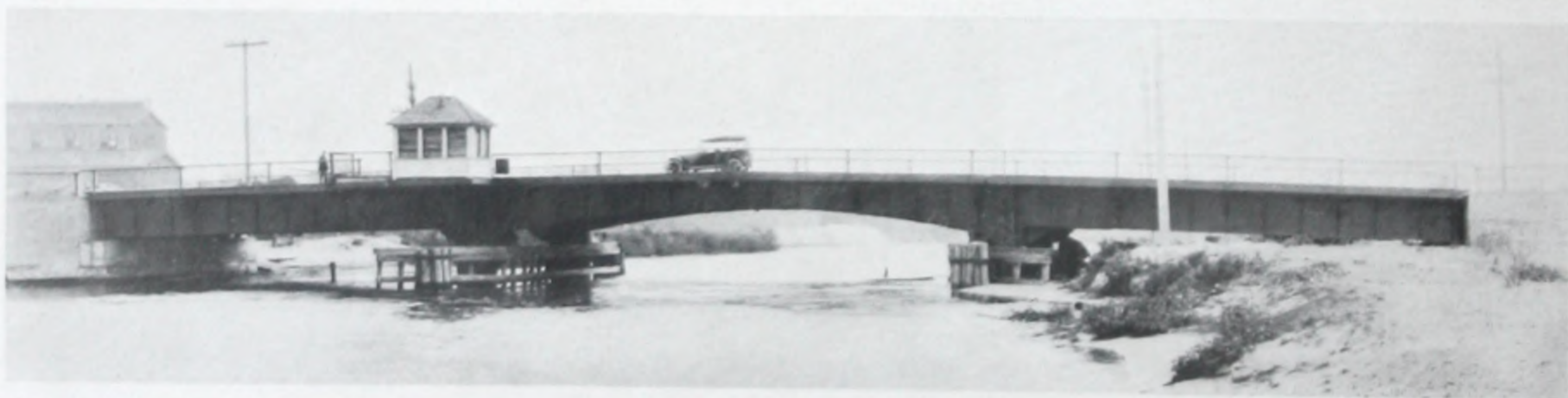
FIGURE 12. (A) AND (B) SHORT SPAN DOUBLE LEAF UNDERNEATH COUNTERWEIGHT, HIGHWAY BRIDGE OVER CALCASIEU RIVER, NEAR LAKE CHARLES, LA.
