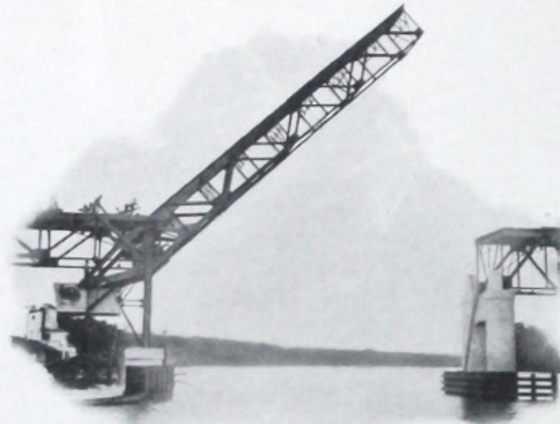
OZAMA RIVER BRIDGE, SANTO DOMINGO
