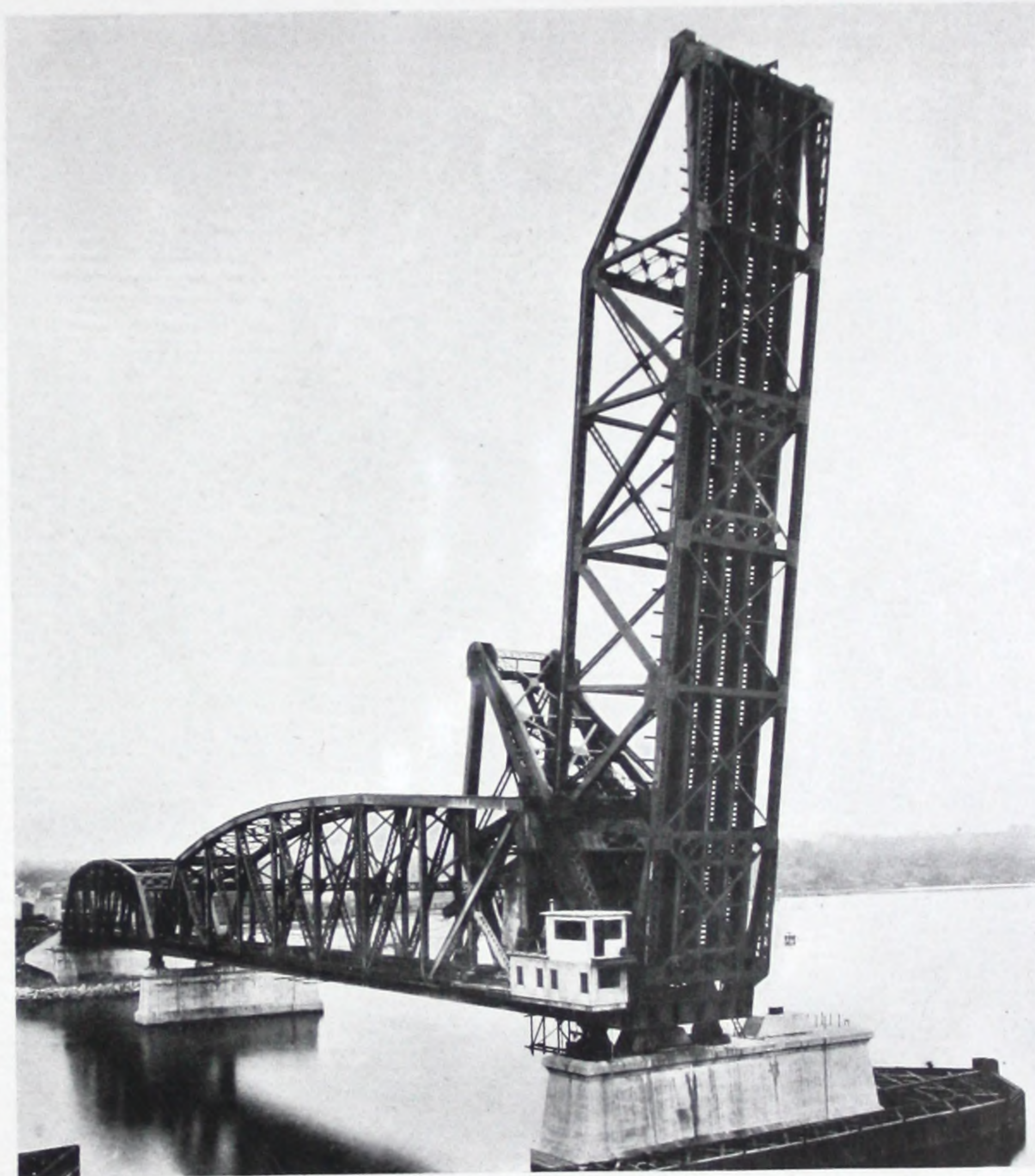
FIGURE 22. SINGLE LEAF HEEL TRUNNION BRIDGE, NEW YORK, NEW HAVEN & HARTFORD RAILROAD OVER THAMES RIVER, NEW LONDON, CONNECTICUT
