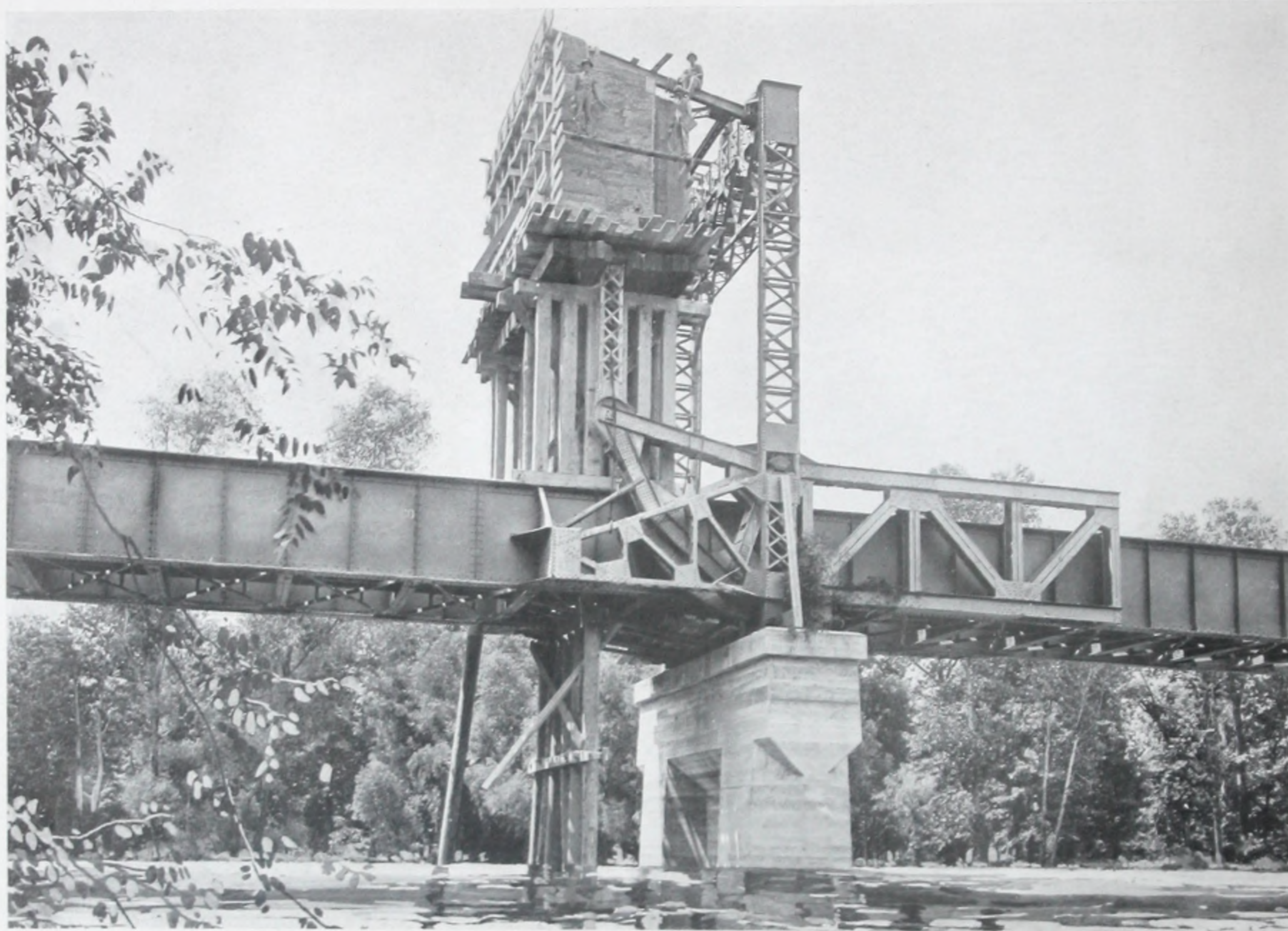
FIGURE 4. SINGLE LEAF OVERHEAD COUNTERWEIGHT BRIDGE, ILLINOIS CENTRAL RAILROAD. "LIFTING TRUSS DESIGN" OVER BIG BLACK RIVER, ALLEN, MISSISSIPPI
