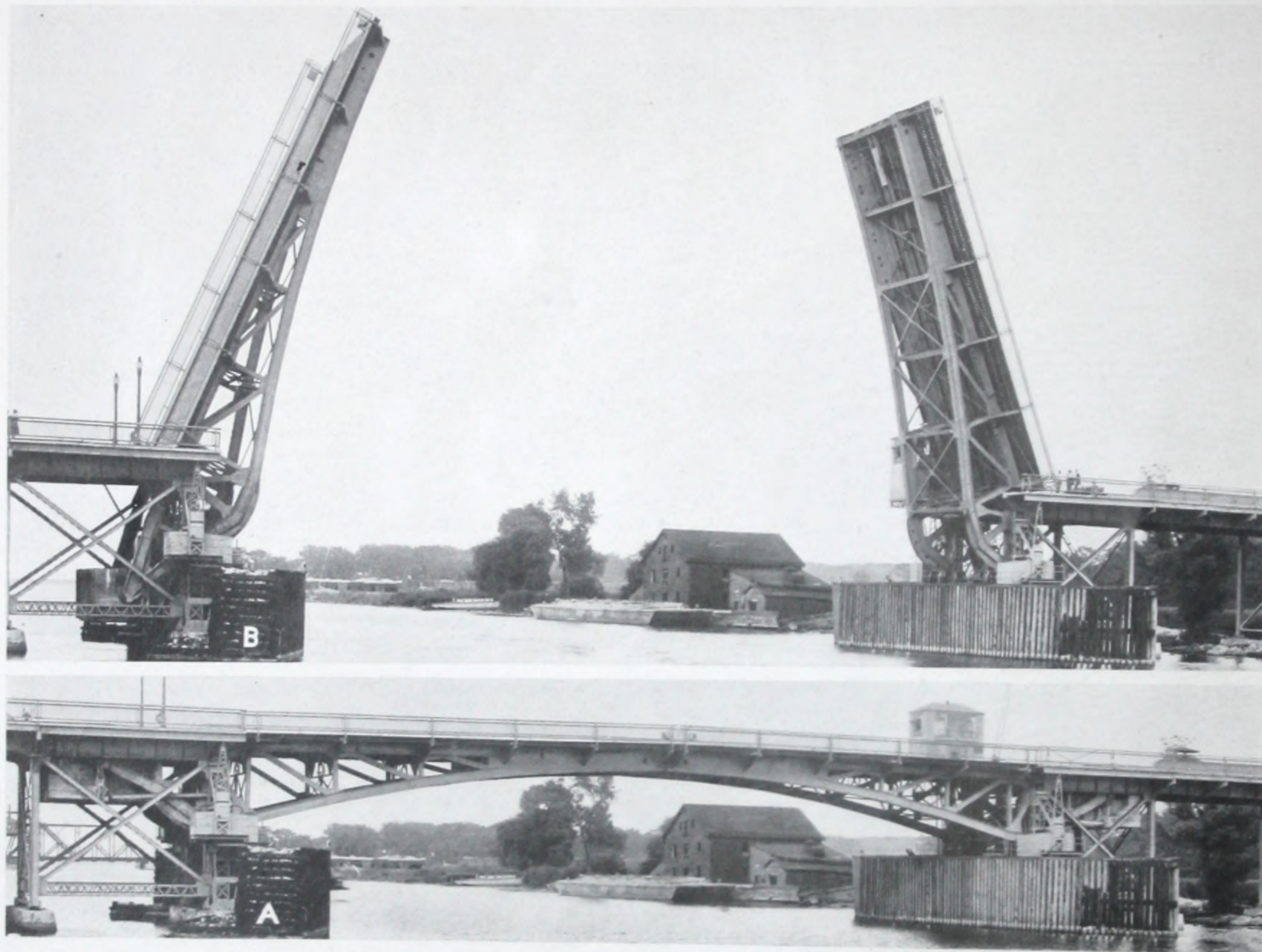
FIGURE 7. (A) AND (B) DOUBLE LEAF UNDERNEATH COUNTERWEIGHT HIGHWAY BRIDGE. STUTSON STREET OVER GENESEE RIVER, CHARLOTTE, NEAR ROCHESTER, NEW YORK
