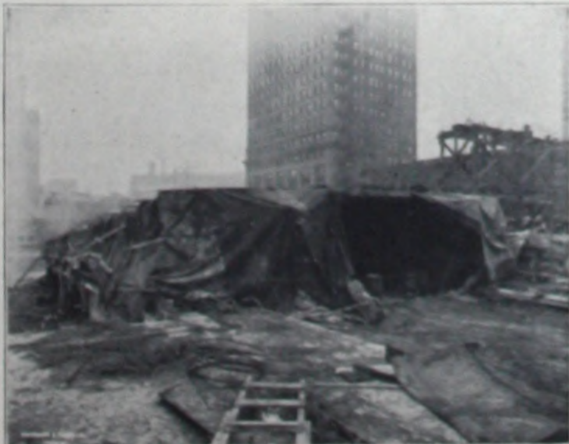
Tents Protecting Concrete in Winter Time.
