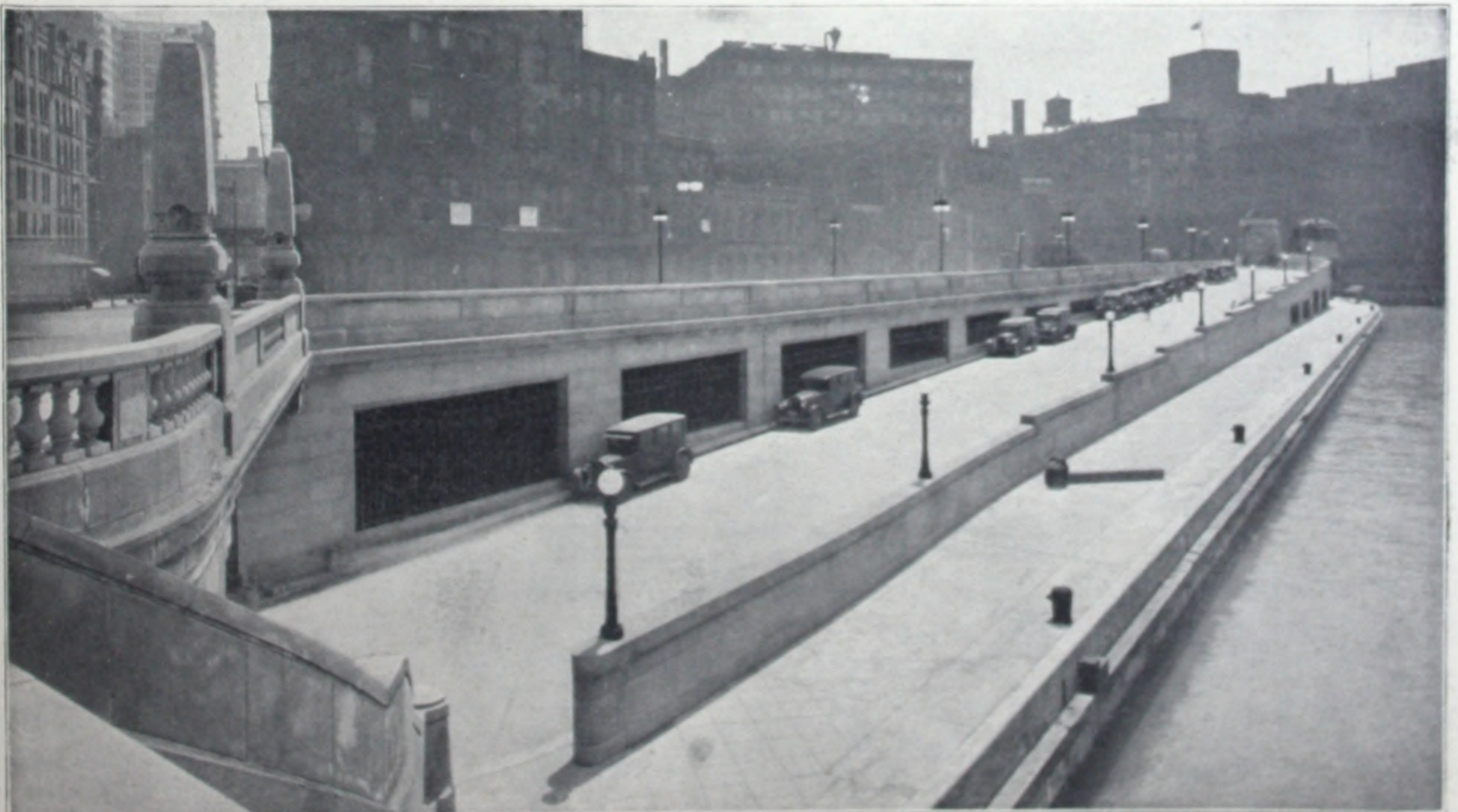
View from Wells Street, Showing Ramp from Upper to Lower Level.
