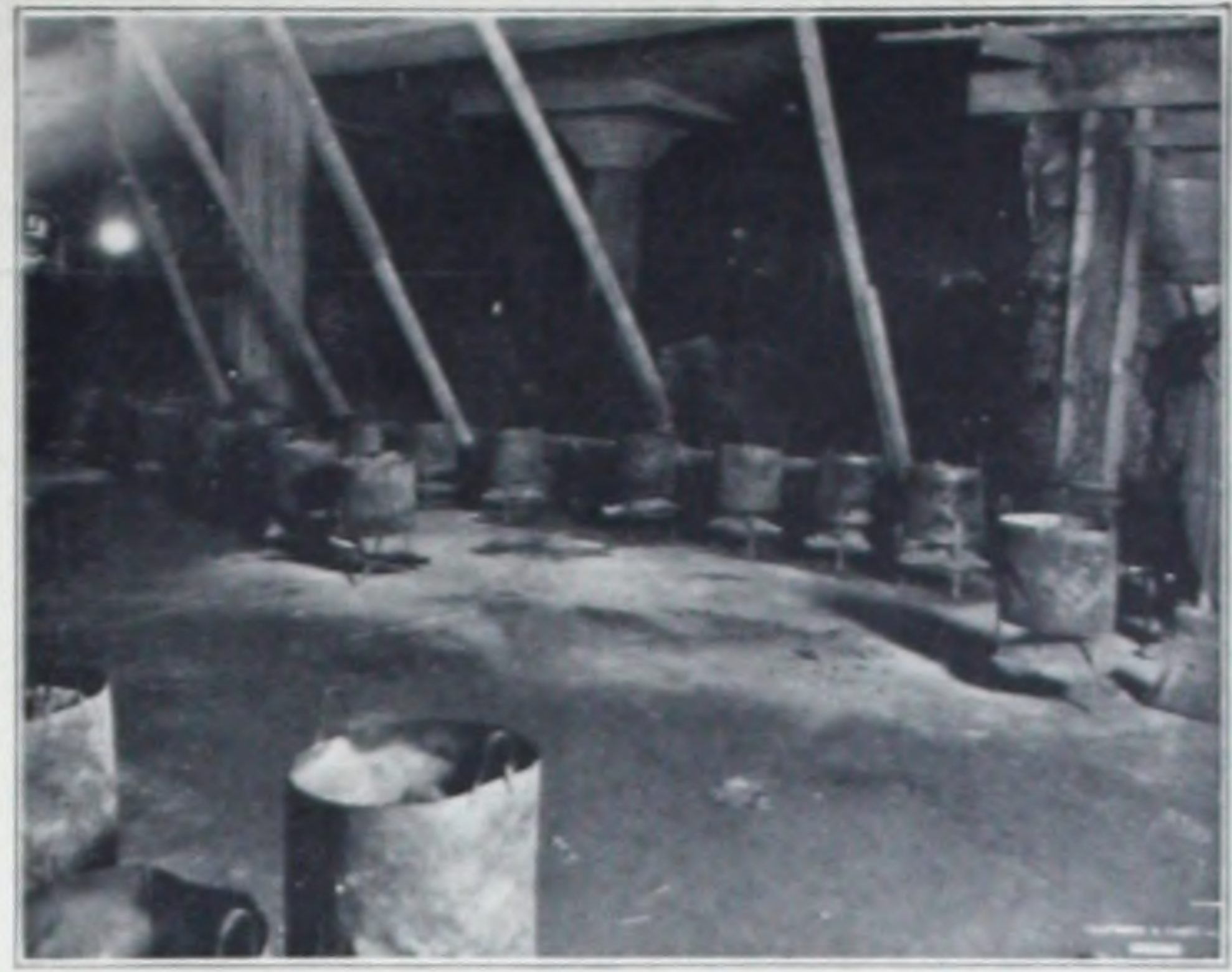
The Salamanders That Kept the Temperature Inside the Tarpaulin 70°.
