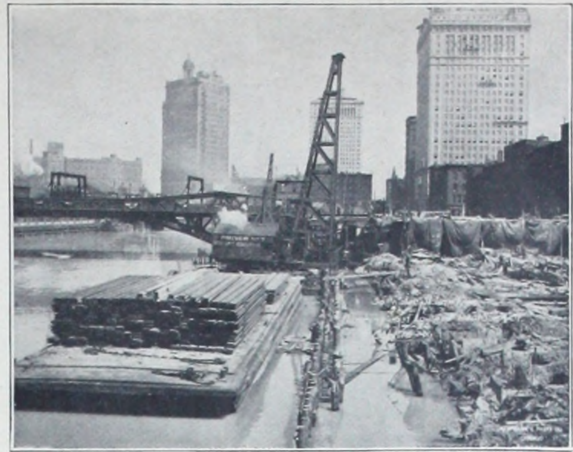
Driving Piles for New Docking.
