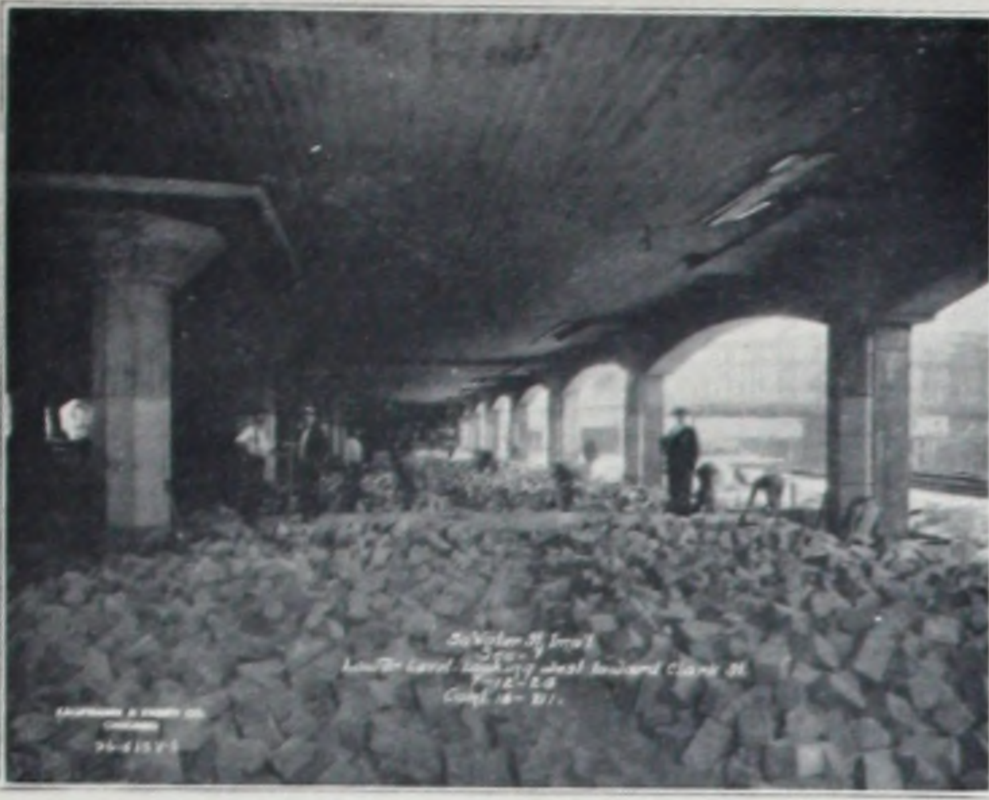
Granite Block Piled Up, Ready to Be Laid
