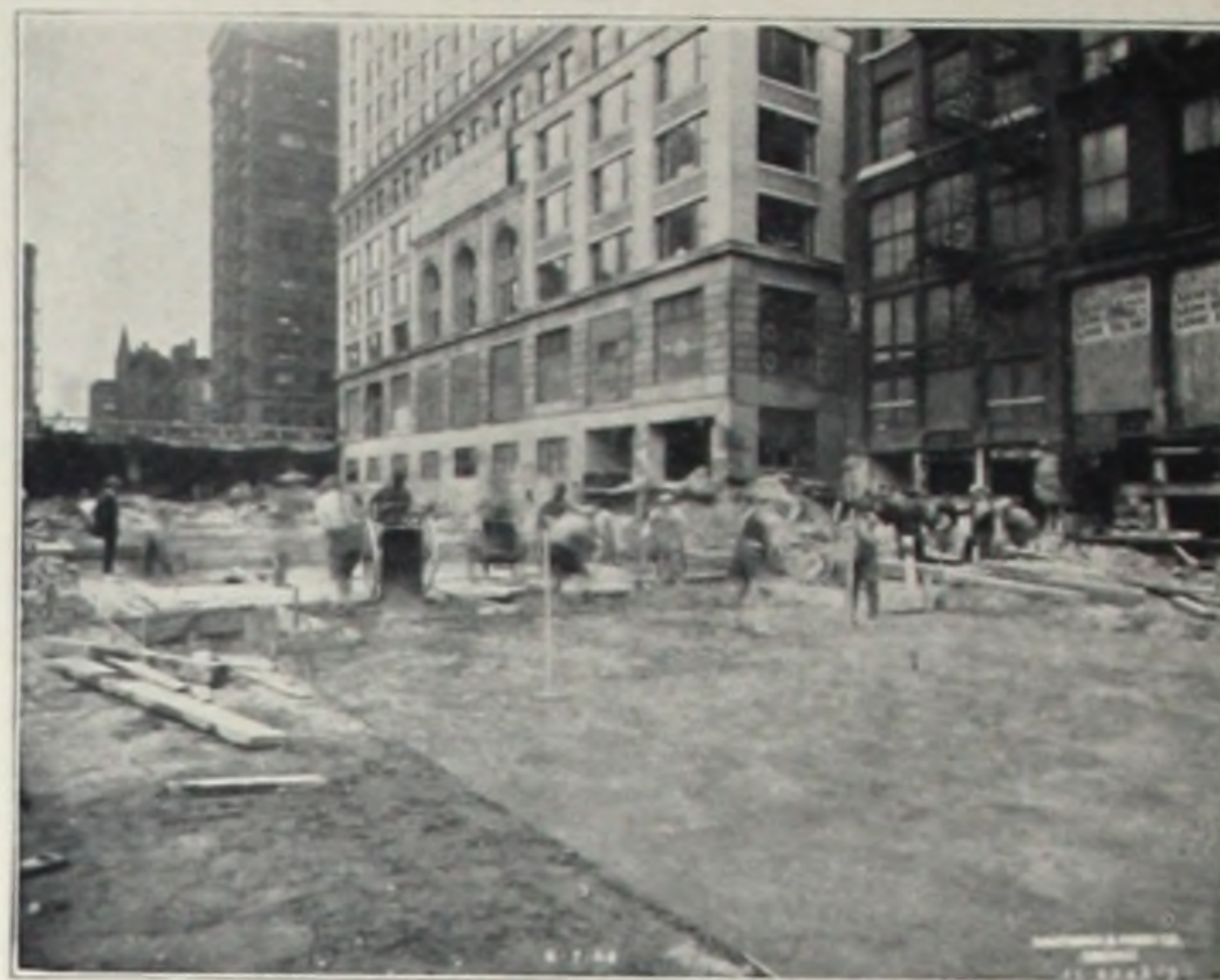
Pouring Concrete in Deck Slab. Buggymen Walked Sixteen Miles Per Eight-Hour Day.
