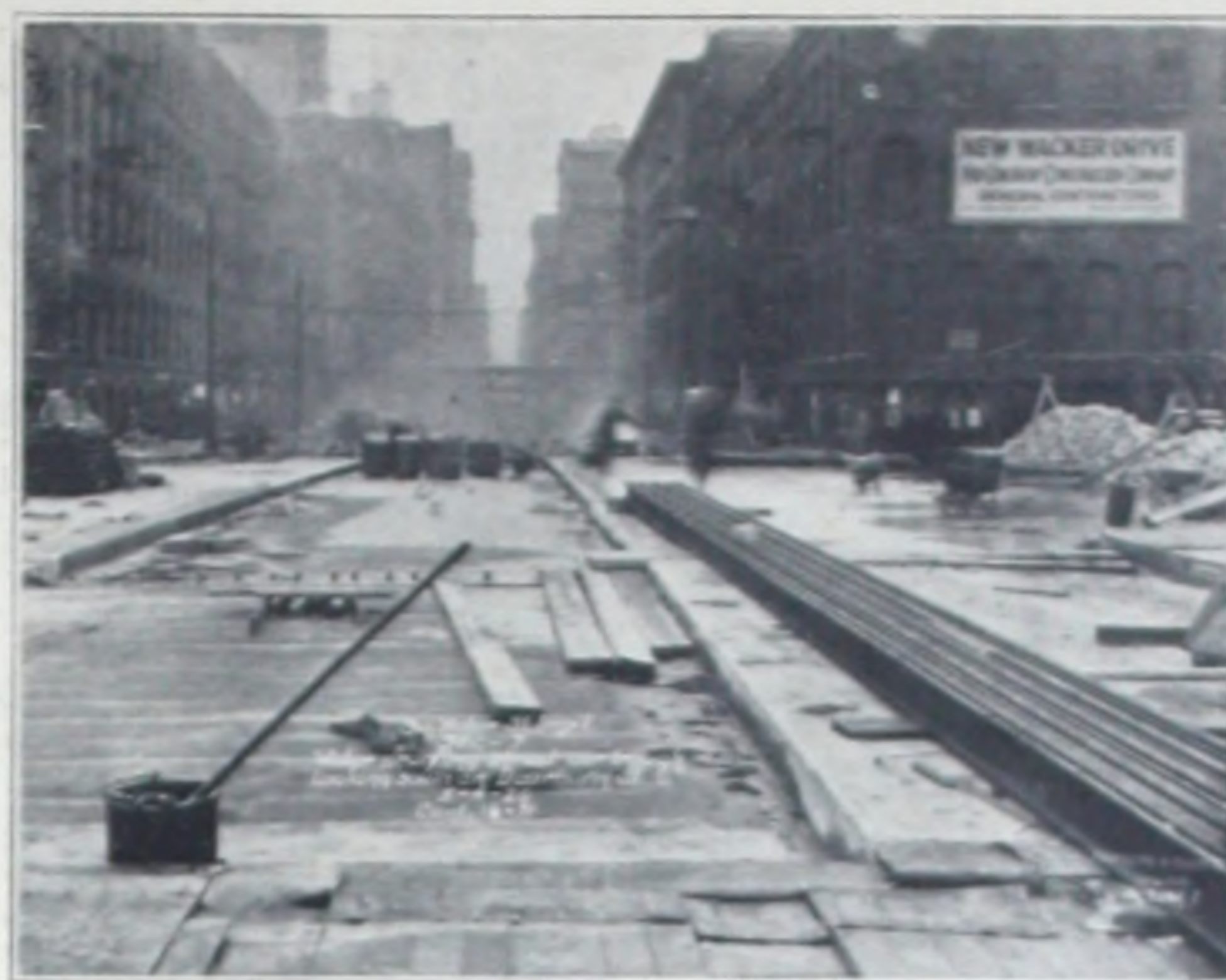
Waterproofing Slab Before Application of Pavement.
