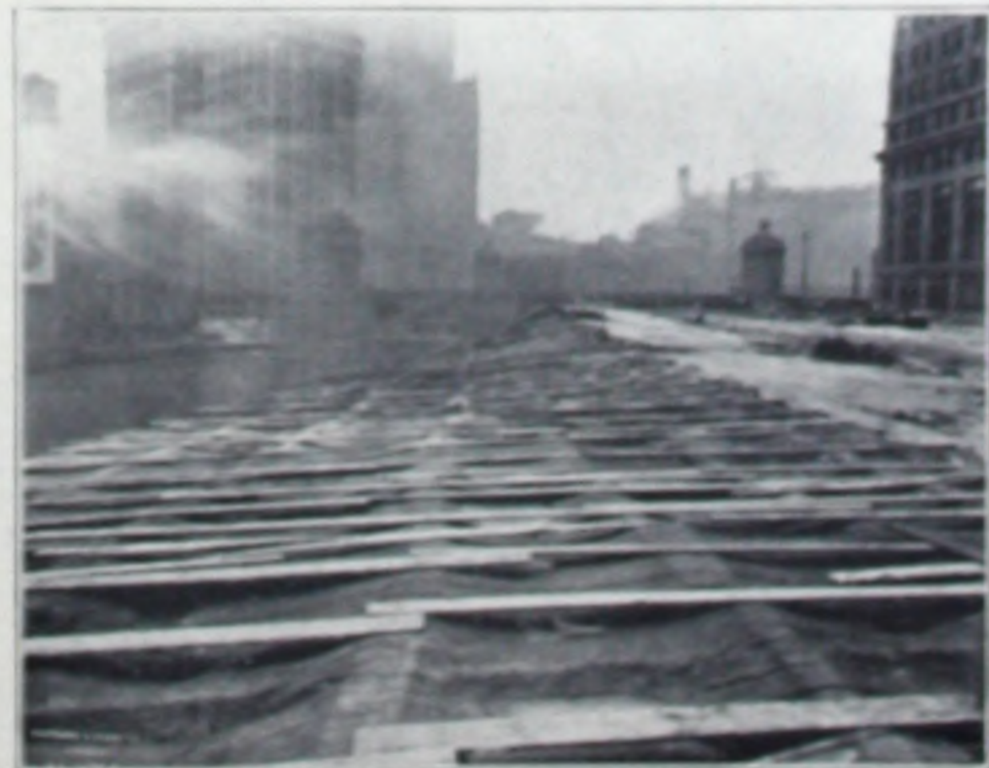
How They Covered the Work in Zero Weather. Acres Covered with Tarpaulins
