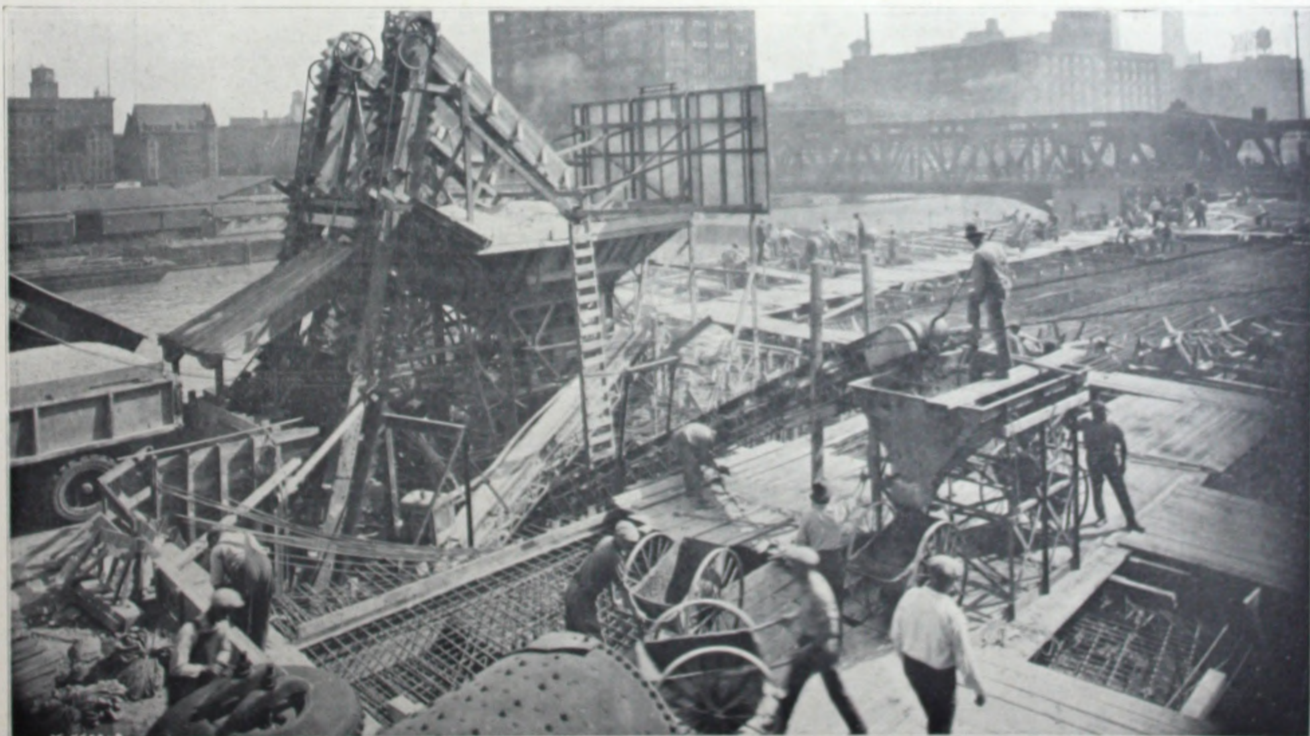
Giant Mid-Continent Concrete Mixer Turning Out Thirty Cubic Yards of Concrete Per Hour. Three of These Were Used.
