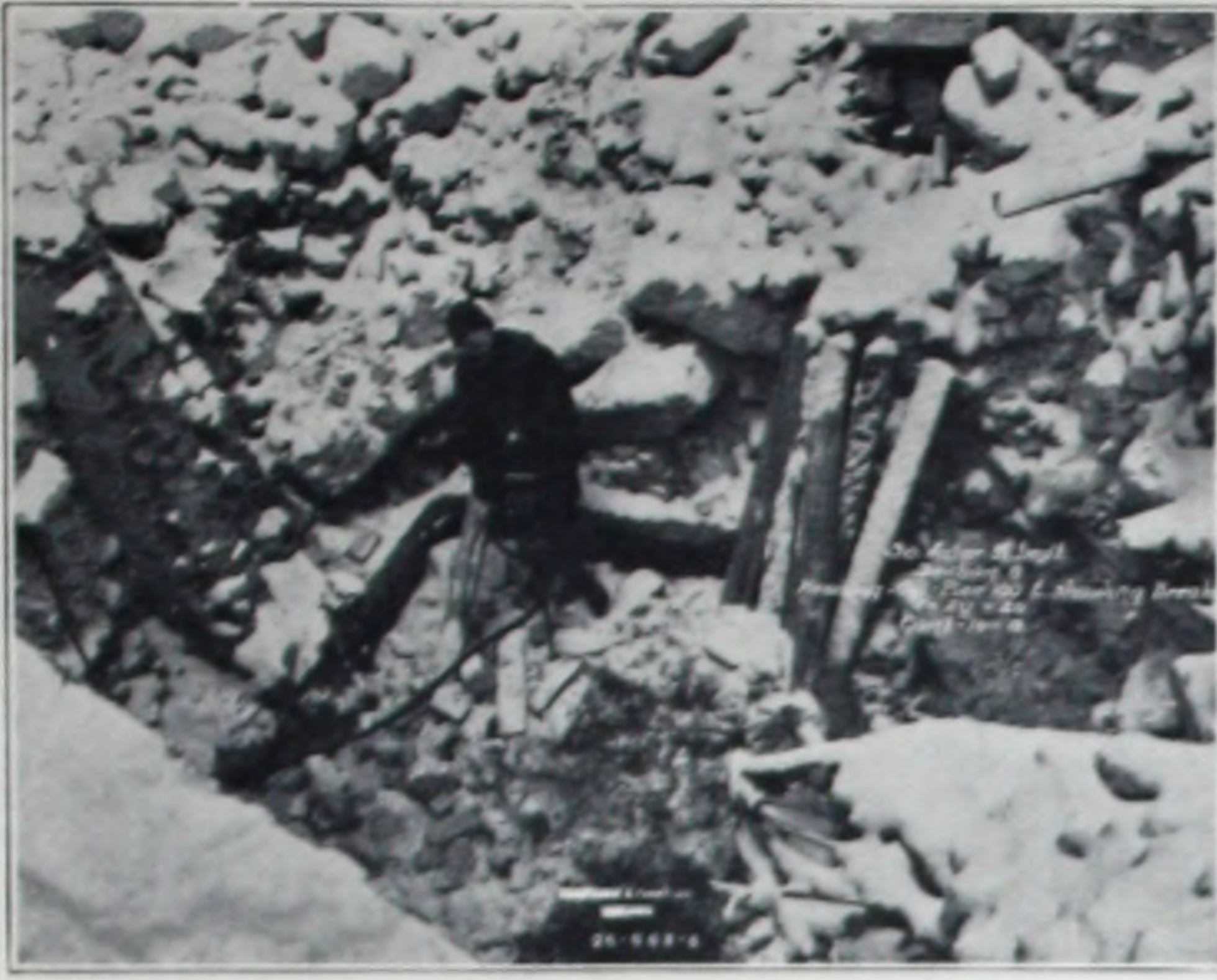
Granite Boulders Being Broken with Concrete Breakers In Winter.
