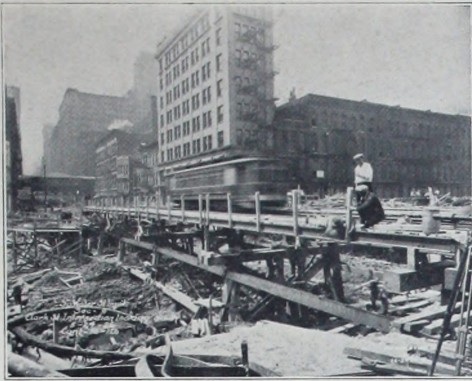
The Constructors Carried the City Traffic on the Back of Their Neck While Building the Job.
