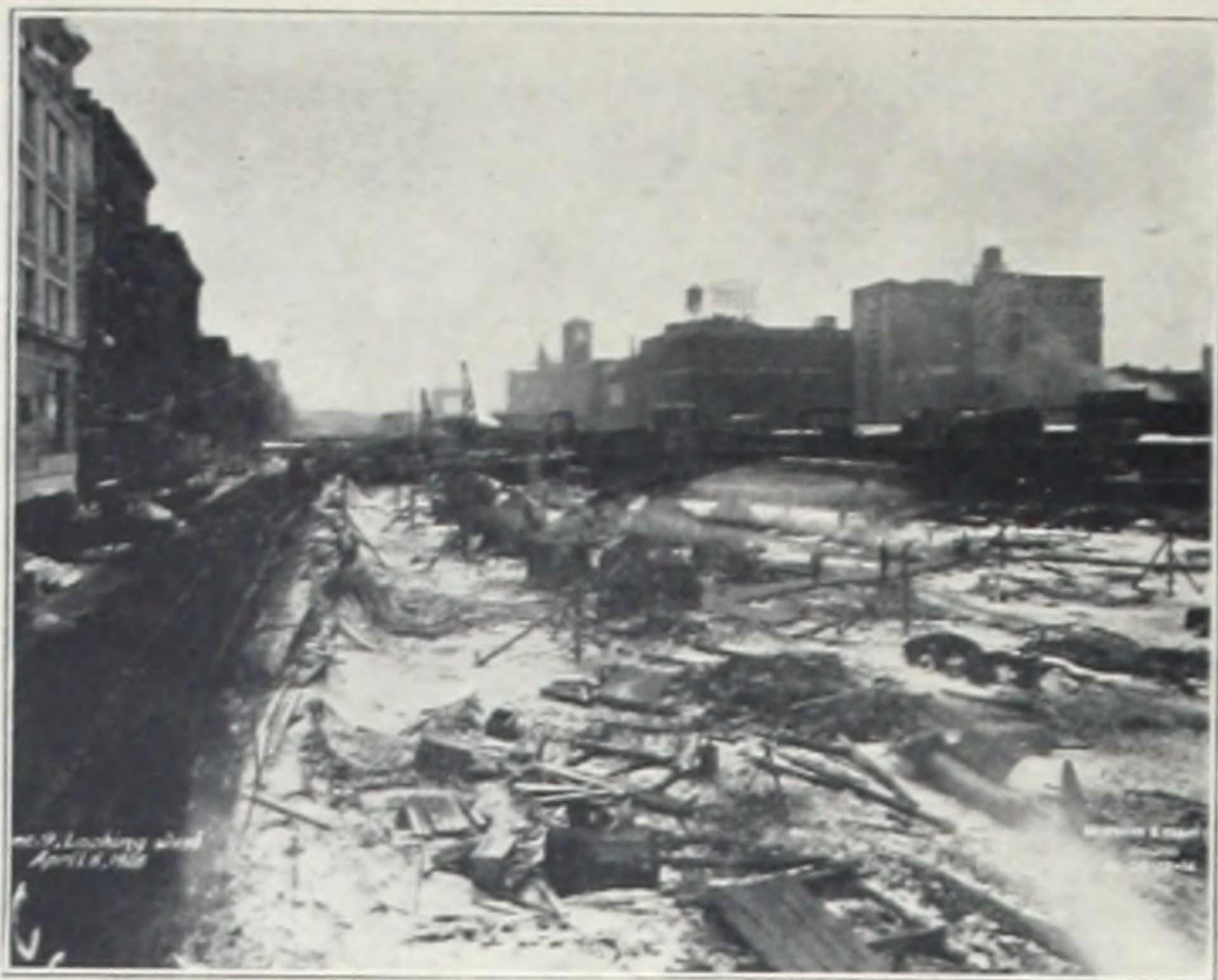
Zero Weather on Top—Building Going on Underneath.
