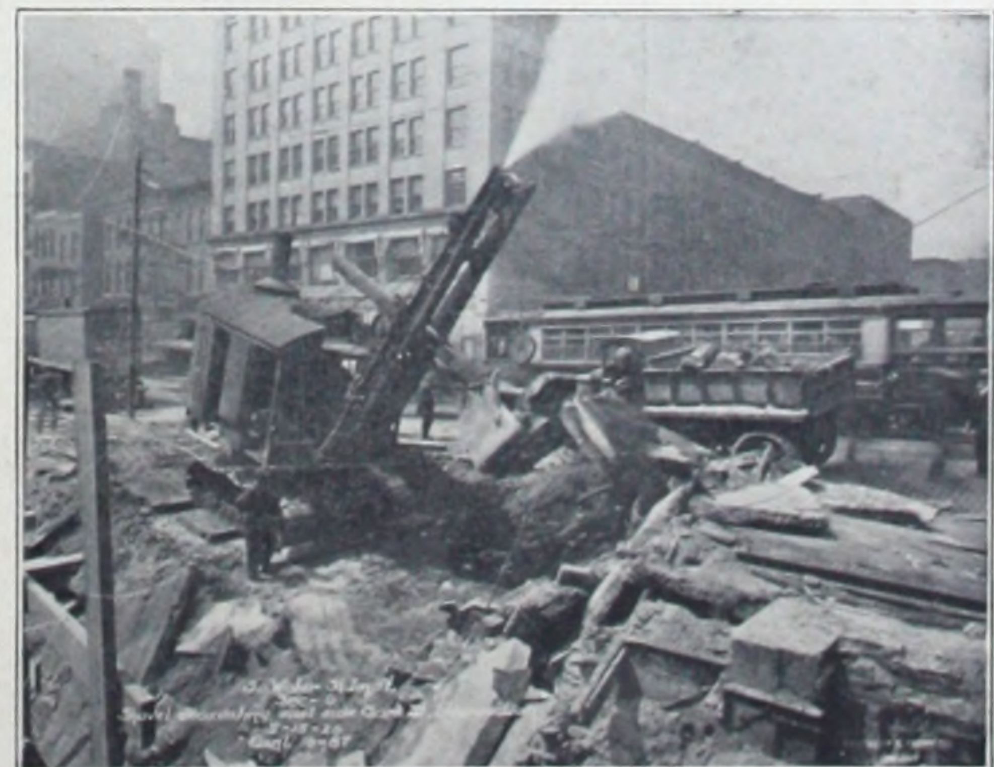
Making the Dirt Fly. Mid-Continent Steam-Shovel Excavating at Clark Street.
