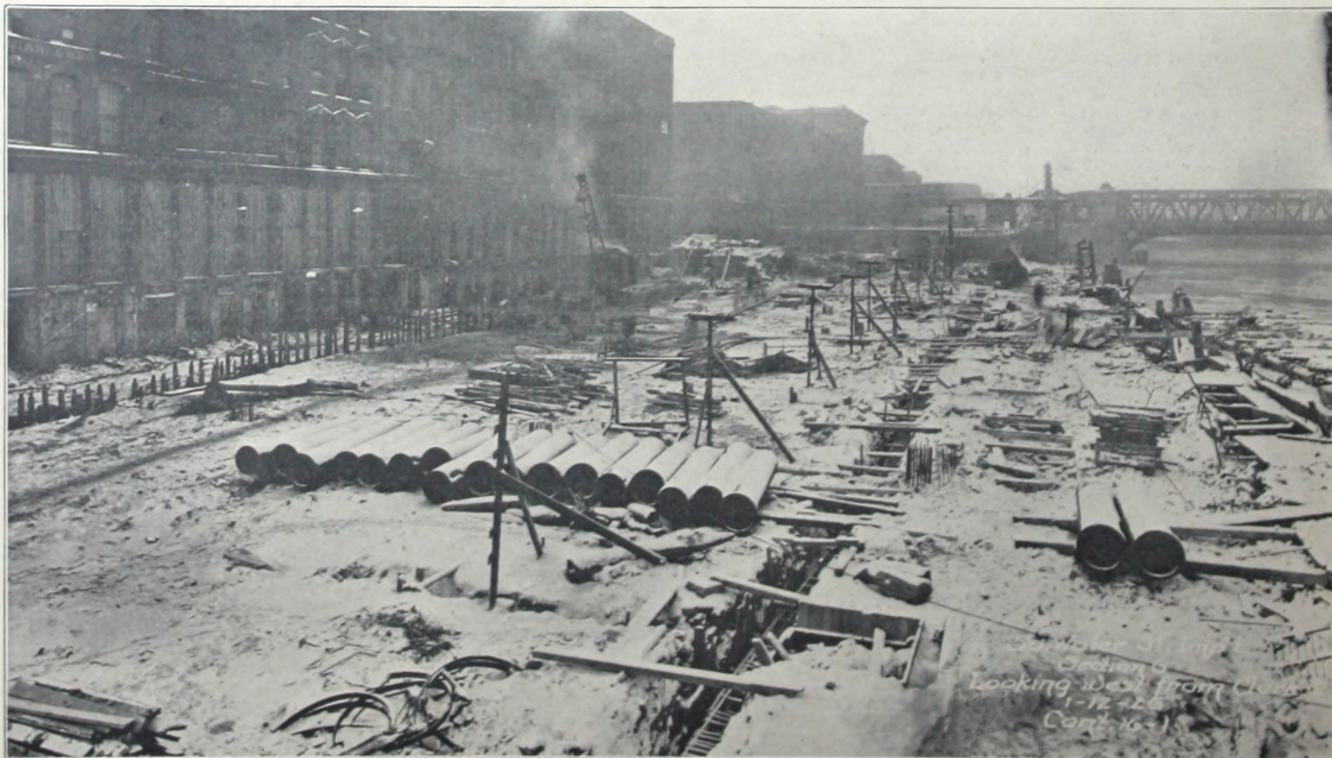
The Depth of Winter, and the Work Going Forward. Trenching for Pipe Lines.
