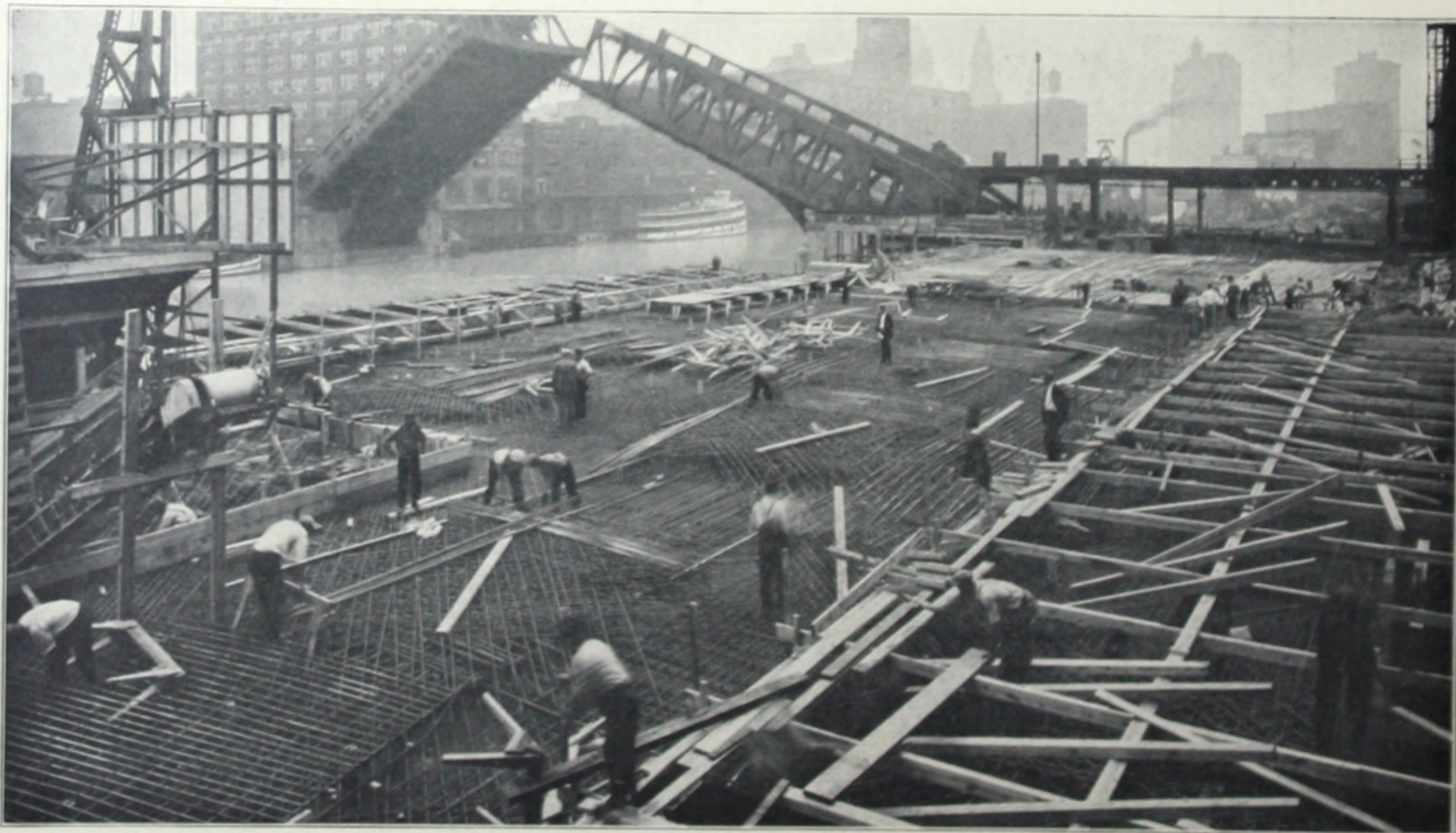
A Network of Steel. Reinforcement for the Concrete of the Driveway.
