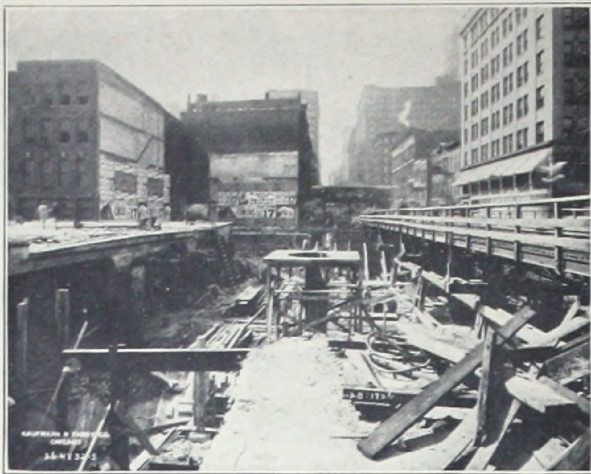
Temporary Trestle Carrying Street Cars While Building Goes on Underneath.
