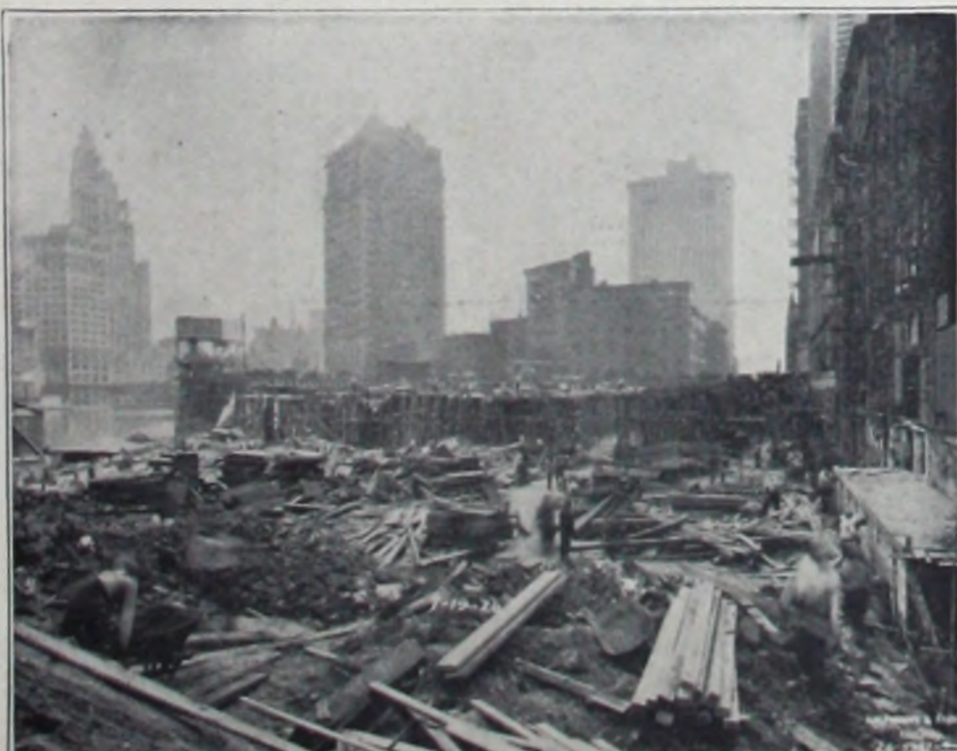
Cleaning Up the Debris.
