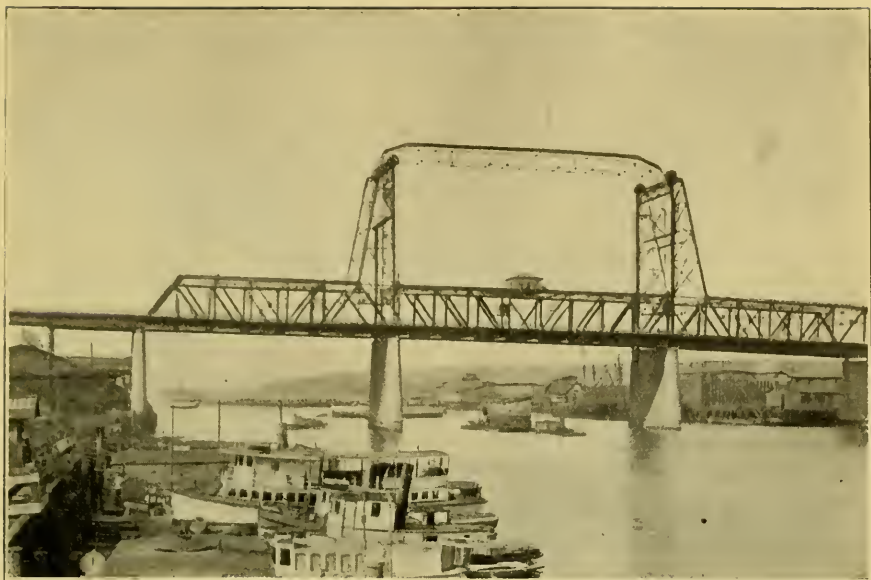
FIG. 31n. Bridge over the City Waterway at Tacoma, Wash.—Lifting Span Down.
