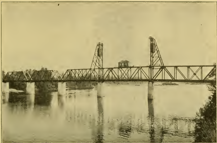
FIG. 31x. Salem, Falls City, and Western Railway Bridge over the Willamette River at Salem, Oregon.—Lifting Span Down.
