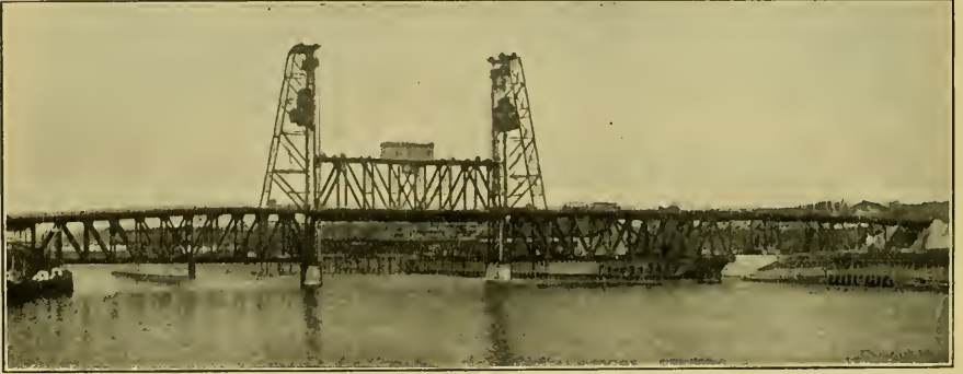
FIG. 31k. O.-W. R. R. and N. Co.'s Bridge over the Willamette River at Portland, Ore.—Lifting Deck Up.
