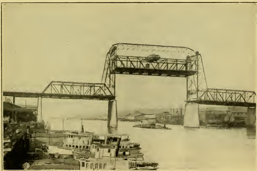
FIG. 31o. Bridge over the City Waterway at Tacoma, Wash.—Lifting Span Up.
