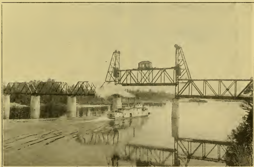
FIG. 31y. Salem, Falls City, and Western Railway Bridge over the Willamette River at Salem, Oregon.—Lifting Span Up.
