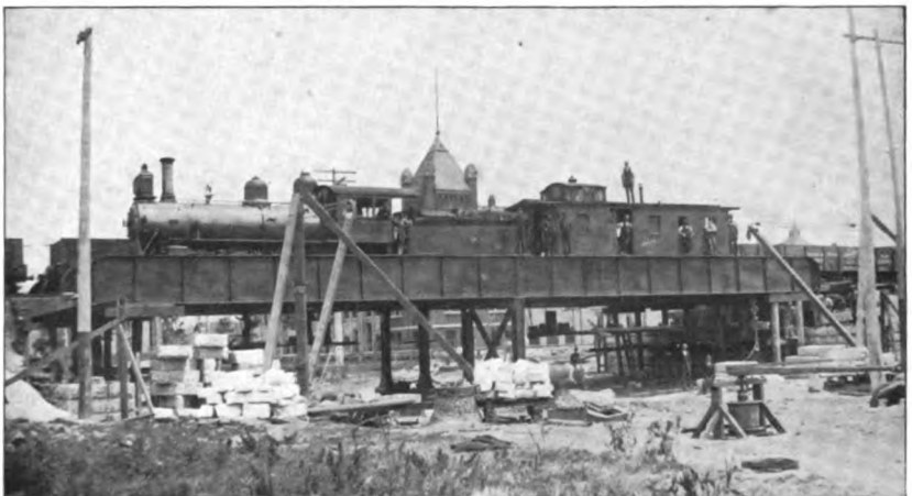
FIG. 458. IRVING PARK BOULEVARD 100 FT. CLEAR SPAN WITH CENTER POSTS. Shows also the building of stone abutments in progress.
