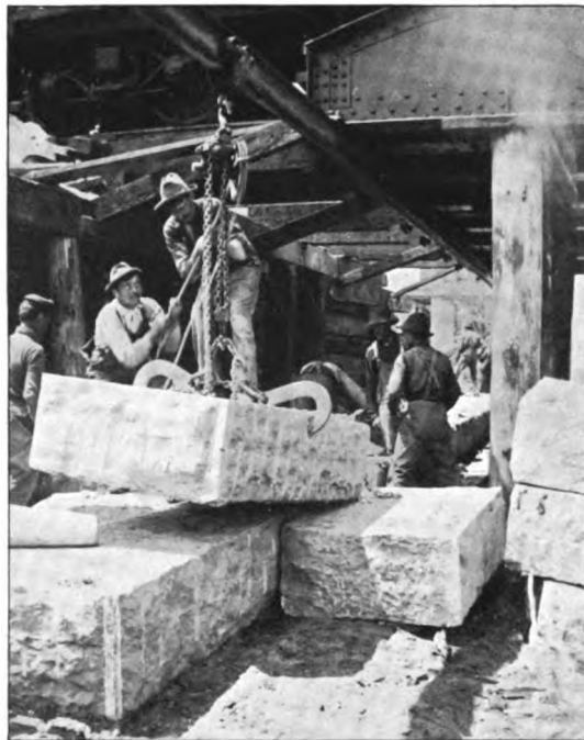
FIG. 472. EIGHT-INCH I BEAM, TROLLEY AND TWO-TON HOISTING BLOCK USED IN LAYING DIMENSION STONE IN ABUTMENTS.
