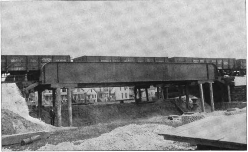
FIG. 453. METHOD OF TEMPORARILY SUPPORTING BRIDGES ON PILING, MILWAUKEE DIVISION.
