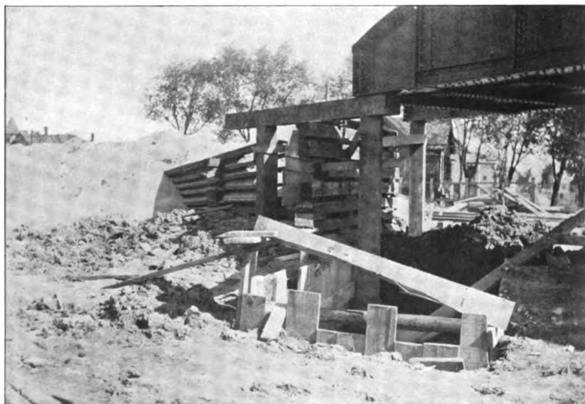
FIG. 469. TEMPORARY END SUPPORT AND BACK WALL.
