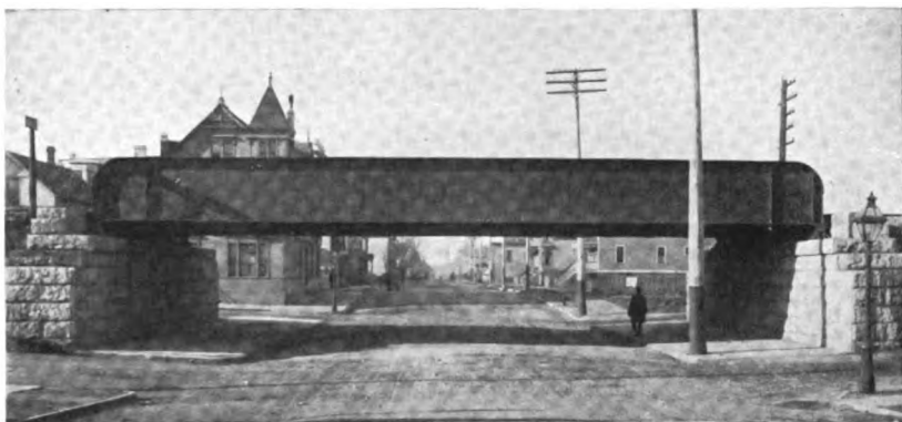
FIG. 450. BRIDGE AT ROSCOE STREET, 66 FT. BETWEEN ABUTMENTS.
