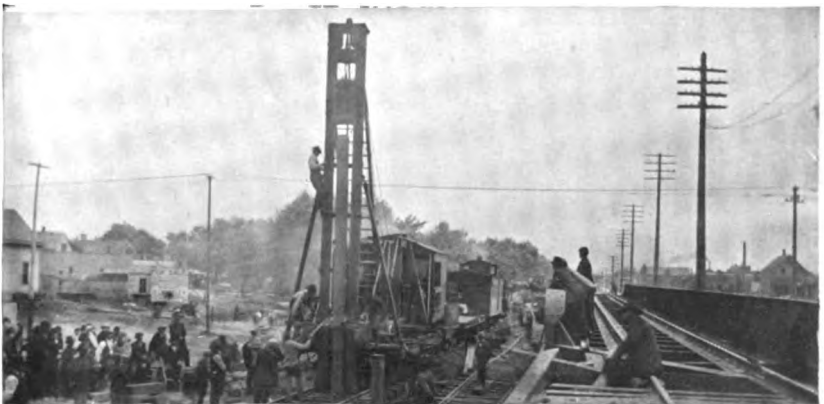
FIG 456. DRIVING PILES FOR TEMPORARY SUPPORT OF EAST TRACK SPAN JULY 9.
