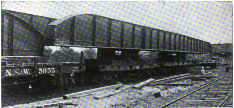
FIG. 466. COMPLETE SPAN LOADED ON CARS FOR DELIVERY ON WORK.
