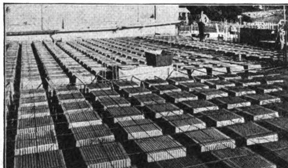
FLOREDOME Construction, Mt. Tabor School, Portland, Ore. Note straight and true lines of FLOREDOMES and accurate spacing of joists.
