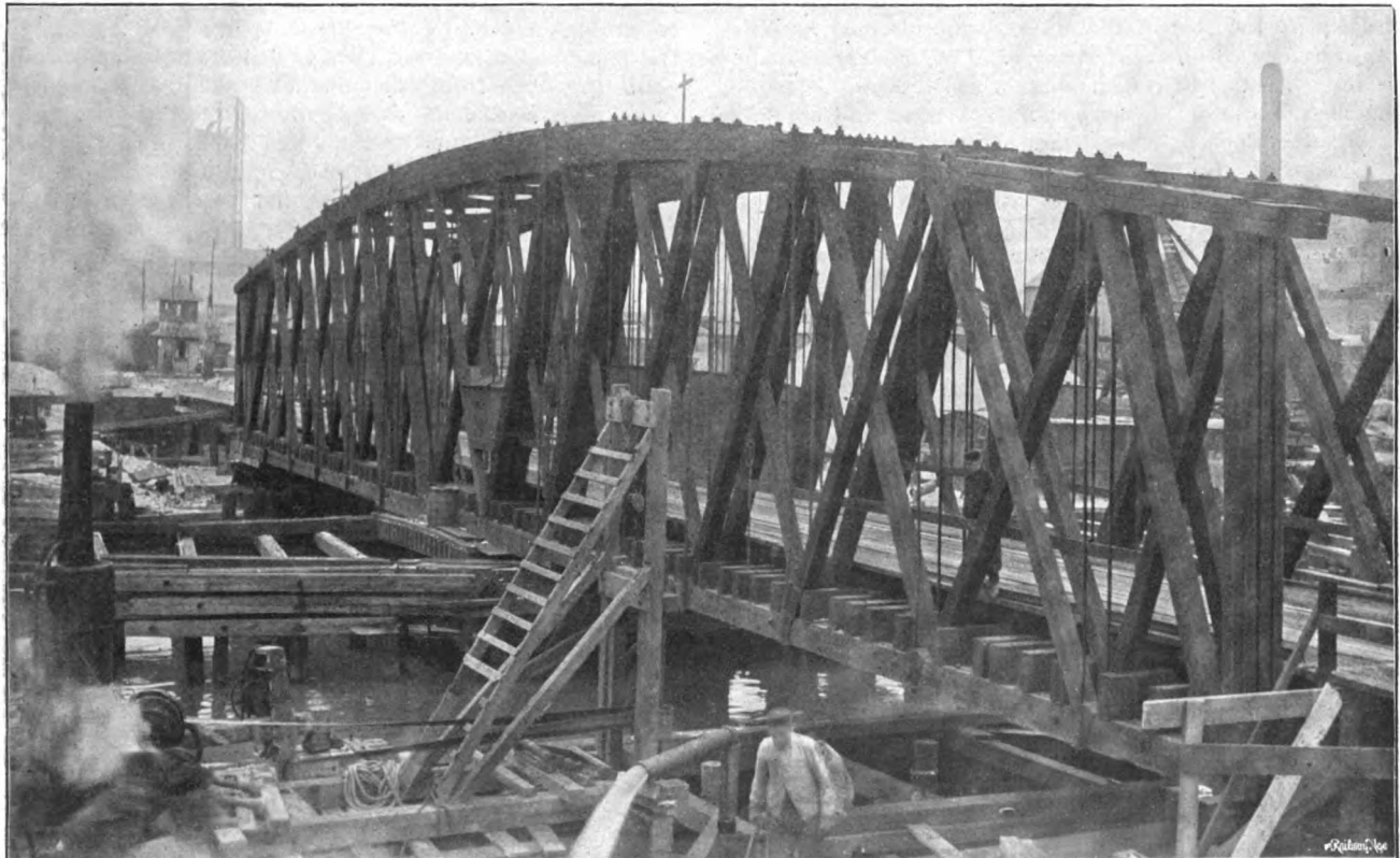
CHICAGO MILWAUKEE & ST. PAUL BRIDGE—OLD STRUCTURE TO BE REPLACED.
