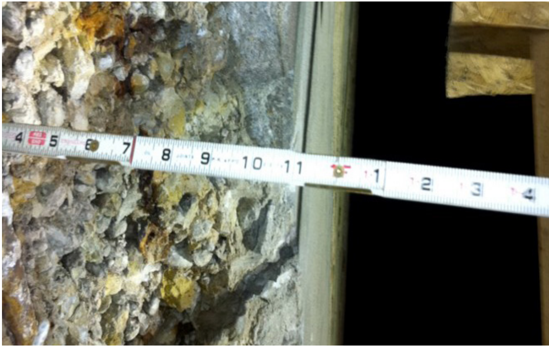
Figure 10 - The Depth of Concrete Repair was 10-12"
