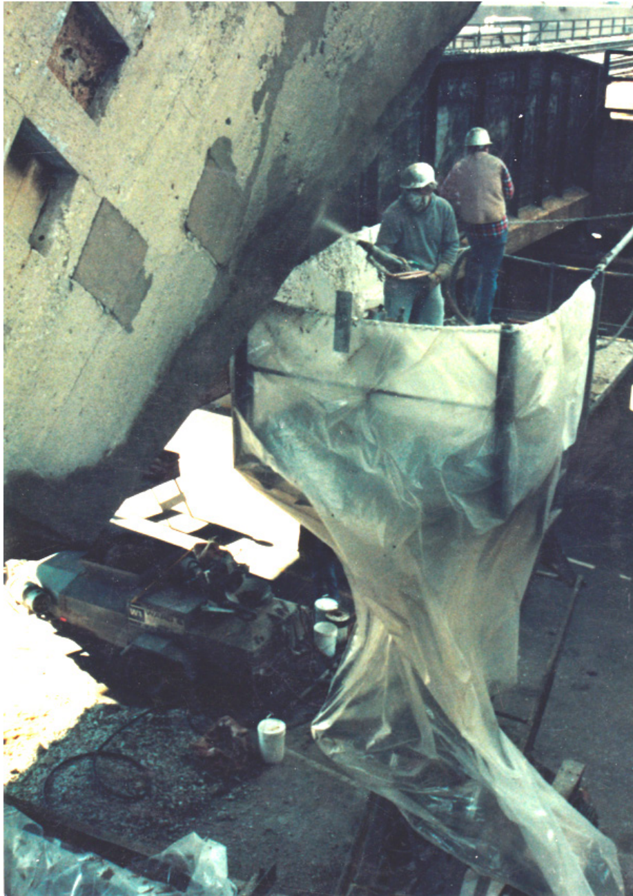
Figure 13 - Wet Mix Shotcrete was Selected for the Repairs
