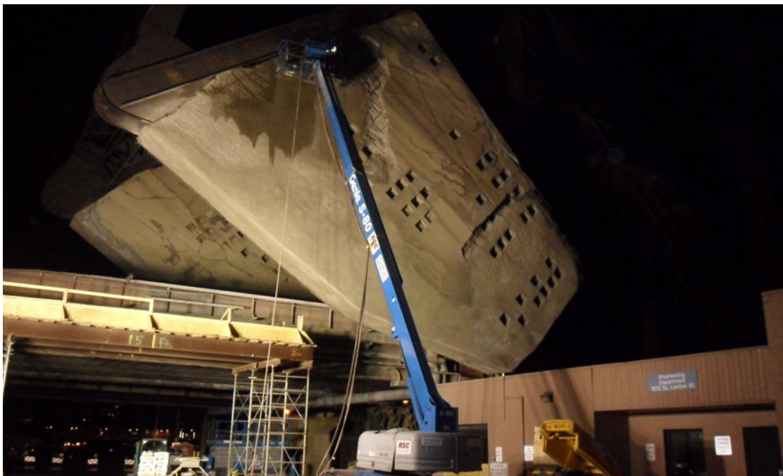
Figure 11 - The Bridge was Raised at Night to Allow Counterweight Access by Boon Lift
