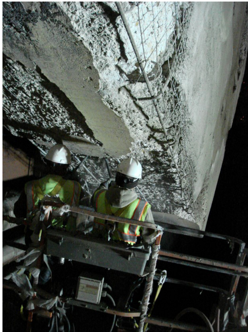
Figure 8 - The 21st Century Repair Plan Required Approx. 9,000 ft 2 of Surface Repairs
