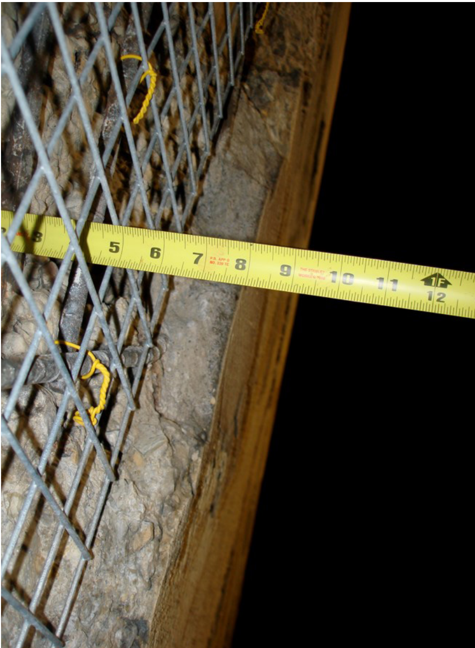
Figure 12 - Installation of 2"x2" Galvanized Welded-Wire Fabric
