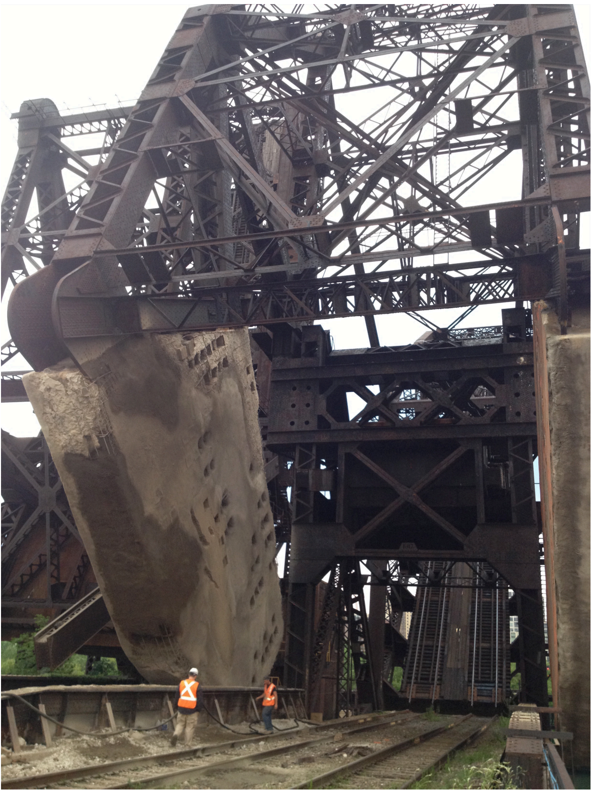
Figure 14 - 2014 Repairs in Progress
