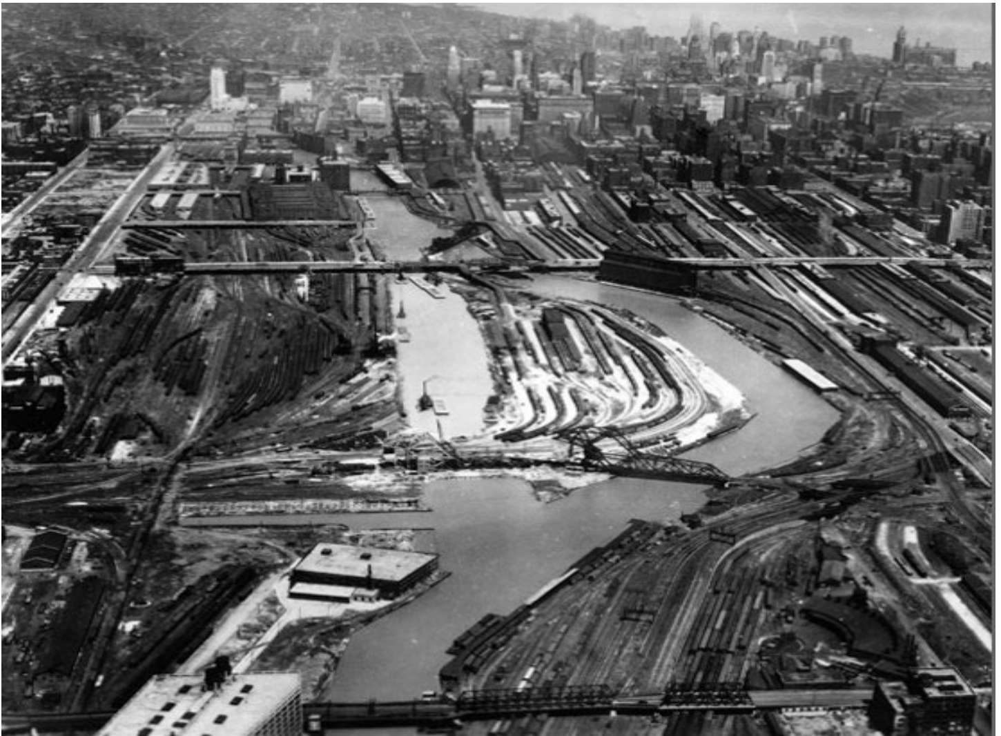
Figure 3 - The South Branch of the Chicago River was Straightened and the Bridge Relocated in 1930
