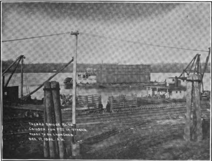
Caisson for Pier 3
