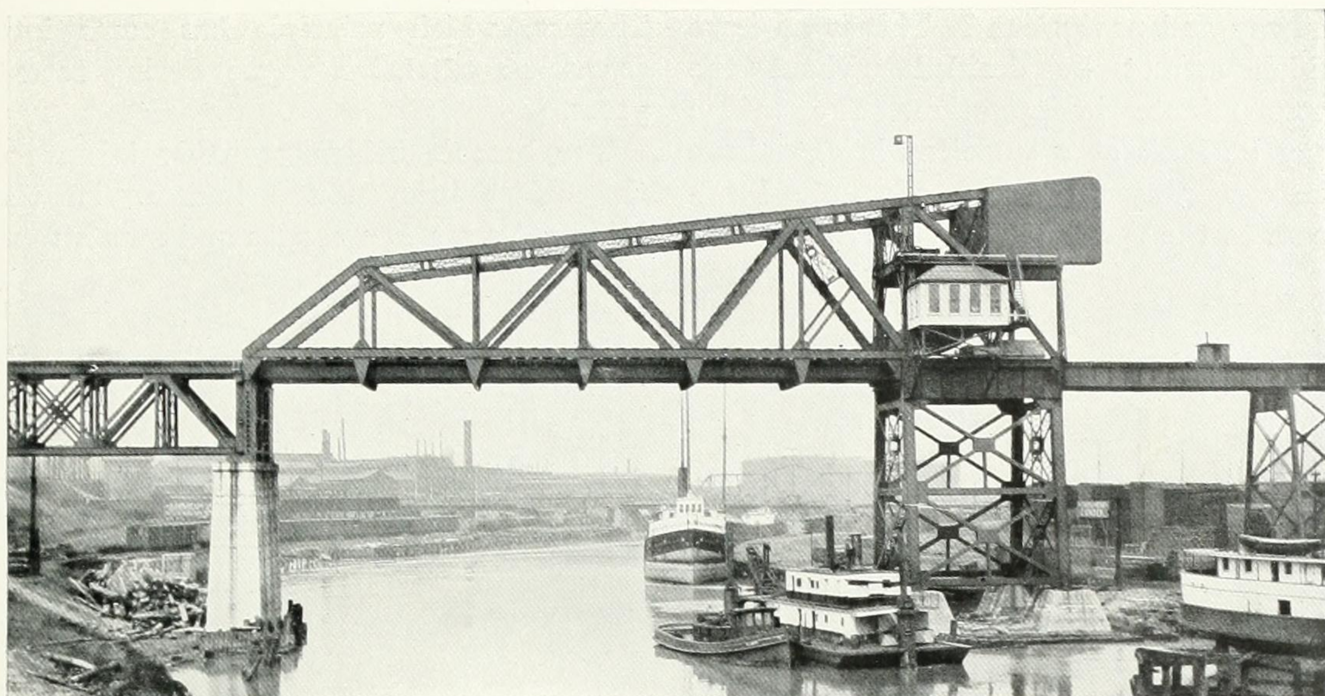
160-FOOT SINGLE-LEAF DOUBLE-TRACK SCHERZER ROLLING LIFT BRIDGE ACROSS THE CUYAHOGA RIVER AT CLEVELAND, OHIO, U.S.A., IN CLOSED POSITION.
