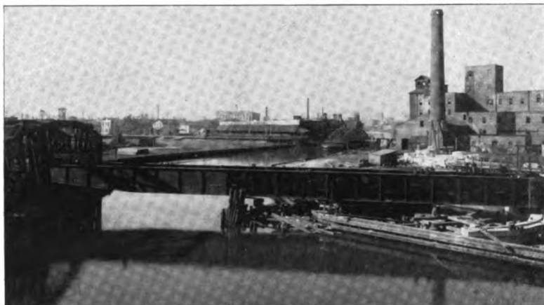
Fig. 11.--Bridge in Place.
