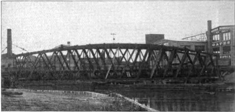
Fig. 7.—The Old Wooden Truss with Track Elevated Across it.
