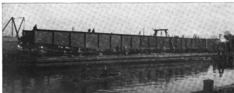
Fig. 12.--Shows Bridge After Reaching Full Height with Jacks Still Under it.
