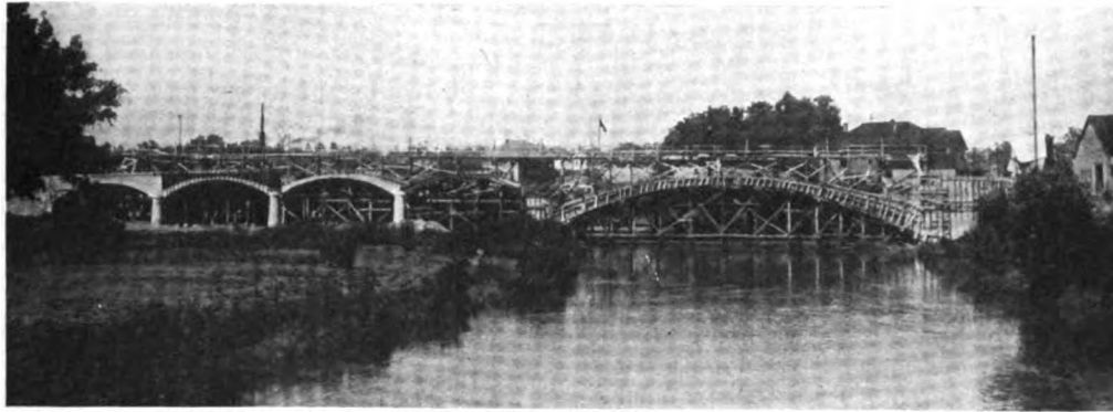
General View of the Bridge Under Construction.
