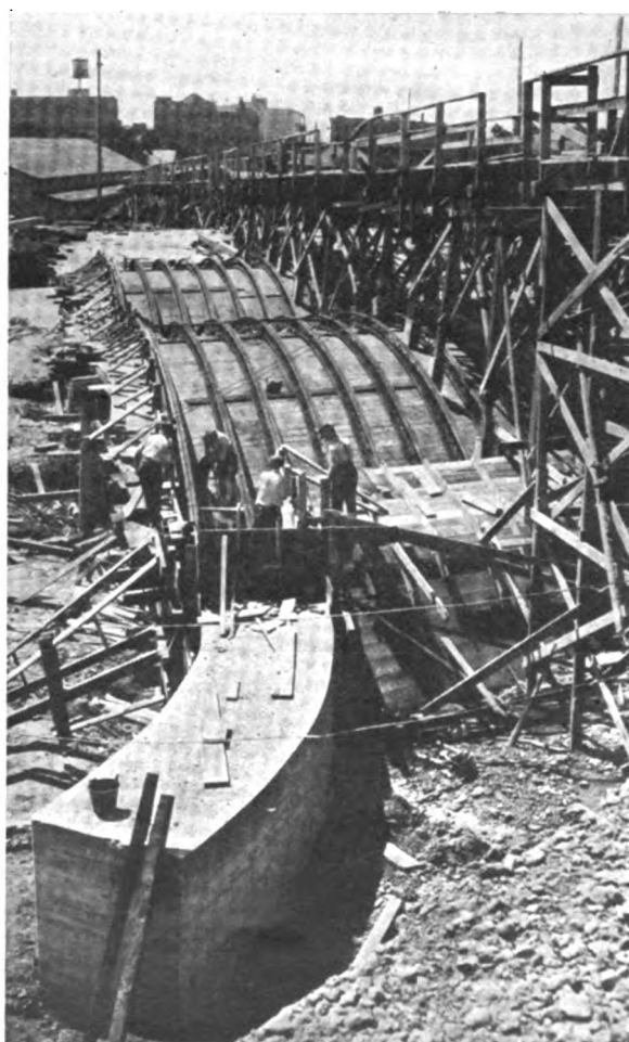
View Along Bridge, Showing Reinforcing Ribs and Trestle.
