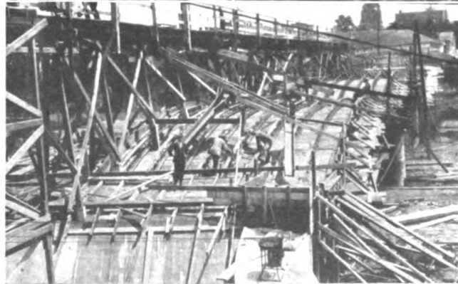
Above—Placing Lagging on Form for Large Arch. Left—Hoist Tower and Track for Foundation Concrete. Right—Guy Derrick, Aggregate Piles and Bins Over Mixer. Below—View Along Bridge, Showing Reinforcing and Trestle Construction.
