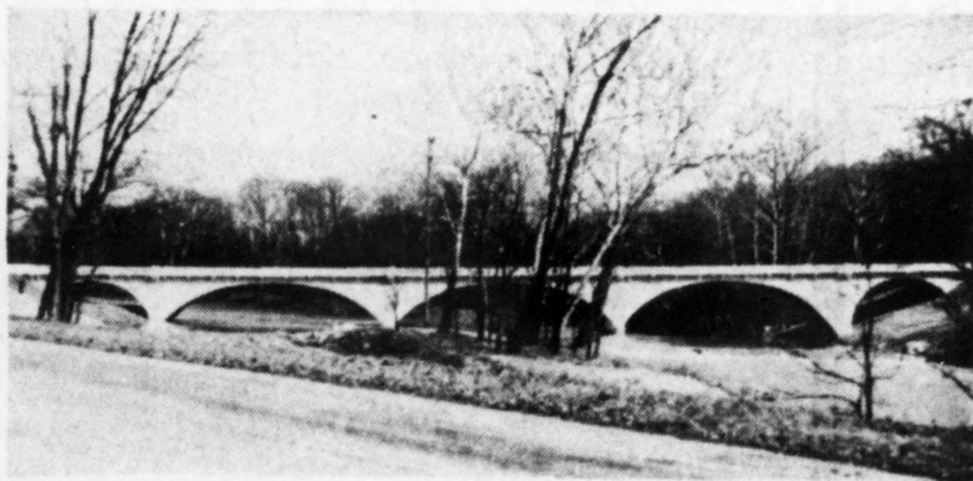
These bridges are designed to carry 90-ton caterpillar tread army trucks if moved slowly to avoid effect of impact.
