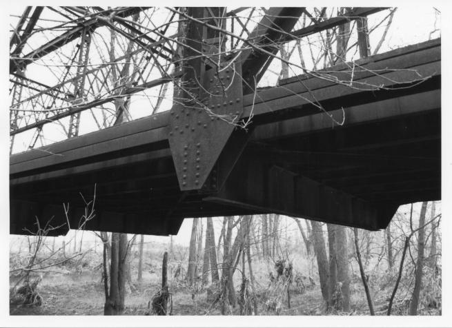
Photo 2 County Line Bridge Hancock Co. Indiana Guy Booth Dec. 3, 1993 Historic Landmarks Foundation of Indiana Detail of Gusset Plate, Bottom Chord and Floor beam From West
