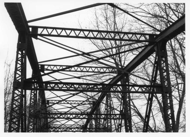
Photo 4 County Line Bridge Hancock Co. Indiana Gny Booth Dec. 3, 1993 Historic Landmorks Foundation of Indiana Detail of Panels connecting Top Chords Looking North From South Side of Bridge
