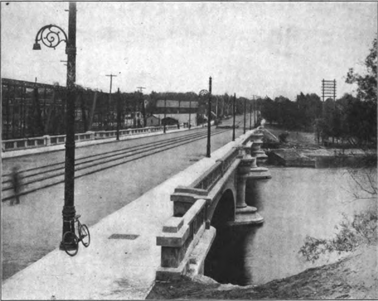
REINFORCED CONCRETE BRIDGE—JEFFERSON ST. SOUTH BEND, IND.
