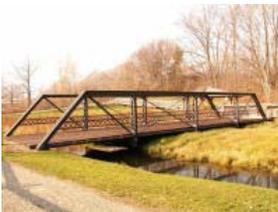
**Bridge Type:** Four panel half-hip Pratt pony truss with pinned connections.
