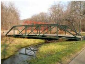
**Bridge Type:** Five panel full-slope Pratt pony truss with riveted connections.
