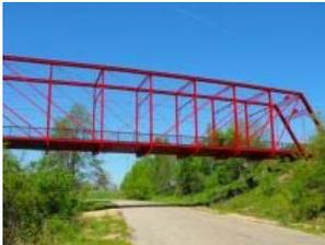
**Bridge Type:** Eleven panel Whipple through truss with pinned connections.
