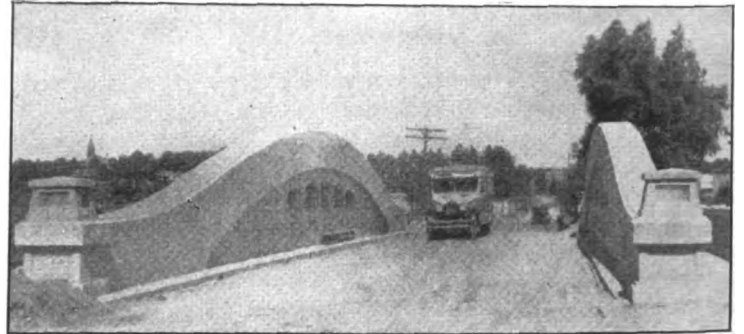
90-Foot Reinforced Concrete Girder, Whitehall, Muskegon County, Crossing White River
