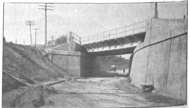
Leoni Grade Separation, Jackson County Traffic Under M. C. R. R.
