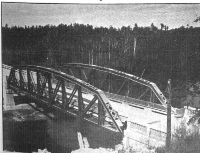
Steel Bridge on M-13 Near Manton, Wexford County, Crossing Manistee River; 18-foot Roadway, 5-foot Walk
