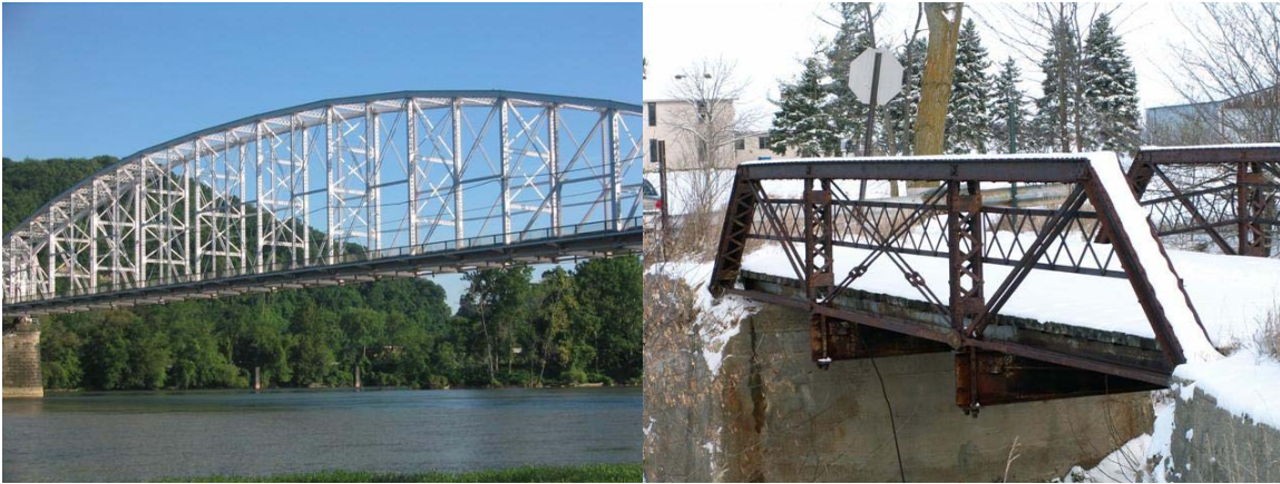
Above left: Hulton Road Bridge over Allegheny River, Allegheny County, Pennsylvania. Above right: Kimpton Road Bridge over Macon Creek South Branch, Monroe County, Michigan. Both of these are truss bridges; networks of triangles make up each bridge. (Nathan Holth)
