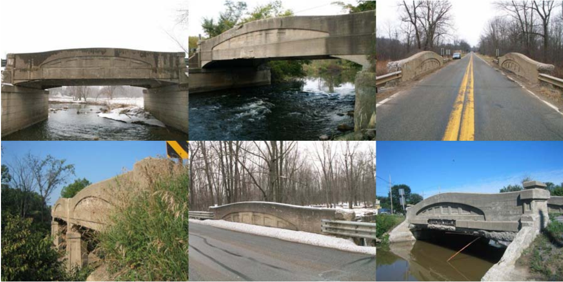
Michigan concrete camelback bridges without pierced openings. Top left: David Highway Bridge over Libhart Creek, Ionia County. Top middle: 23 Mile Road Bridge over Kalamazoo River, Calhoun County. Top right: Folks Road Bridge over Kalamazoo River, Jackson County. Bottom left: Genesee Road Bridge over CN Railroad, Lapeer County Michigan, now demolished. Bottom middle: Borden Road Bridge over Prairie Creek, Ionia County. Bottom right: Vernier Street over Swan Creek, St. Clair County. (Nathan Holth)
