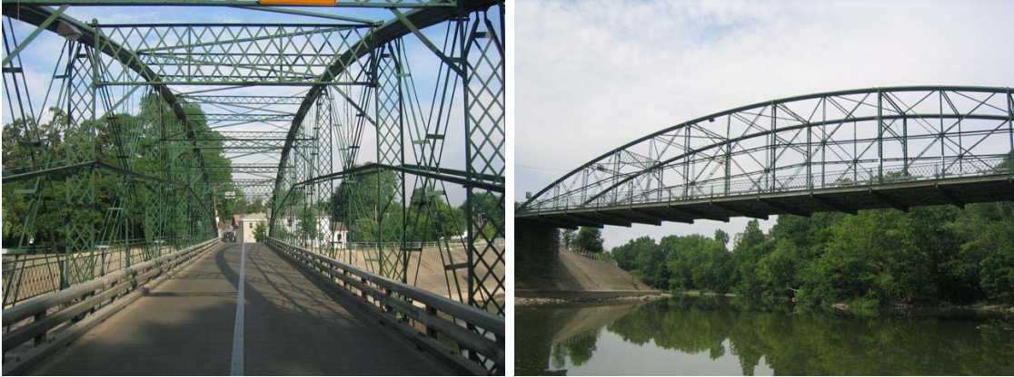
Above: Two views of an 1870s bowstring truss bridge. This is the Blackfriars Street Bridge over North Branch Thames River in London, Ontario. (Nathan Holth)
