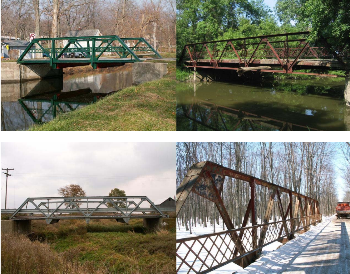
Warren pony truss bridges with riveted connections in Michigan. Top left: Van Buren Street Bridge over Augusta Canal, Kalamazoo County. Top right: Card Road Bridge over North Branch Clinton River, Macomb County. Bottom left: Lewis Road Bridge over Little Salt Creek, Midland County. Bottom right: Reed Road Bridge over North Branch Cass River, Tuscola County. Note that these are one-lane structures. (Nathan Holth)
