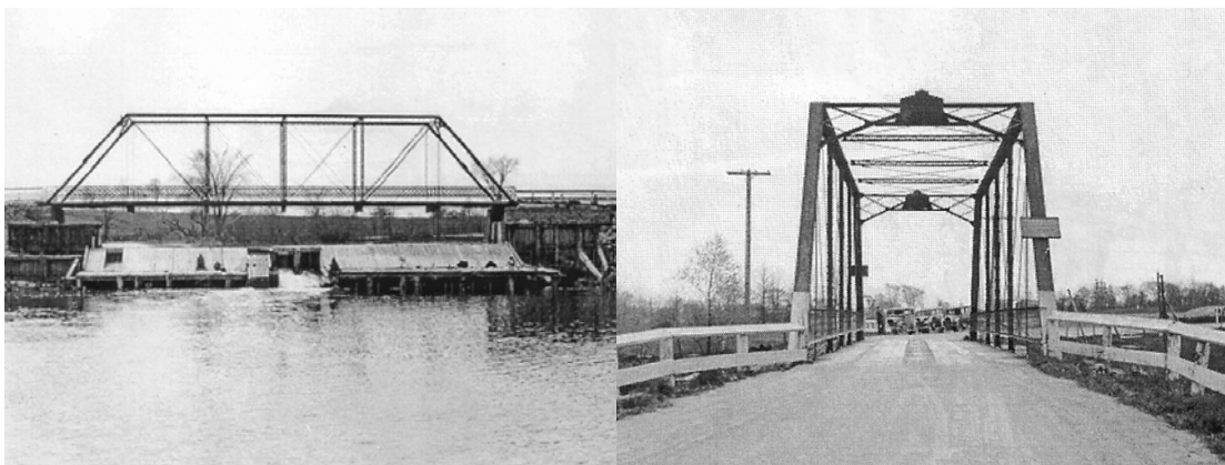
Above left: A side view of the bridge shows the Pratt configuration of the trusses. Also note the dam below the bridge. Above right: Portal view of bridge, showing the
