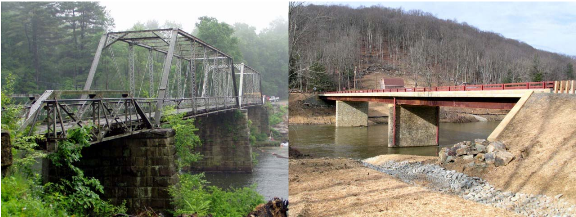
Above left: Shanley Road Bridge over Clarion River, Elk County Pennsylvania, June 2004 (Nathan Holth)
