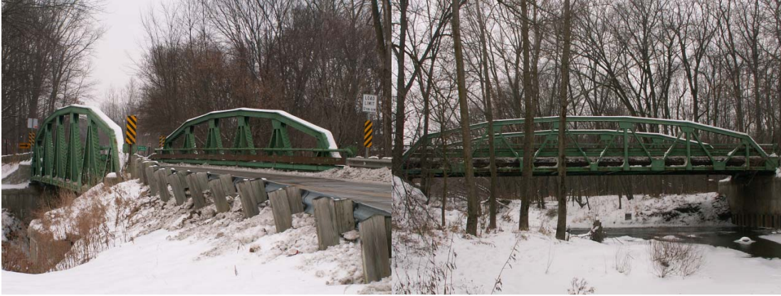
Above: Two views of the Indian Trail Road Bridge as it appears today. (Nathan Holth)
