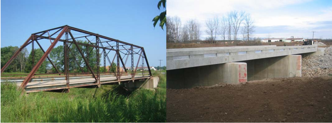
Above left: Church Road Bridge over Black River, Sanilac County Michigan, July 2004
