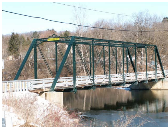
Above: The restored Maple Road Bridge over Huron River, in Washtenaw County, Michigan. (Nathan Holth)
