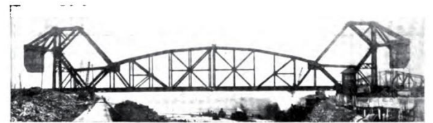
Strauss Heel Trunnion Bascule Bridge over the United States Ship Canal at Sault Ste. Marie. Movable Span, 336 feet. Single Track. The only double-leaf bascule acting as a simple span for live load. Designed by the Strauss Bascule Bridge Co. for the Canadian Pacific Ry. Co. P. B. Motley, Engineer of Bridges; C. C. Schneider, Consulting Engineer.
