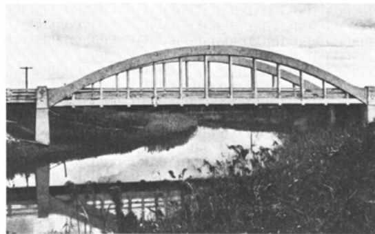
The State's first reinforced concrete bowstring arch bridge, built over Shark Creek on the Pacific Highway near South Grafton in 1935-36.
