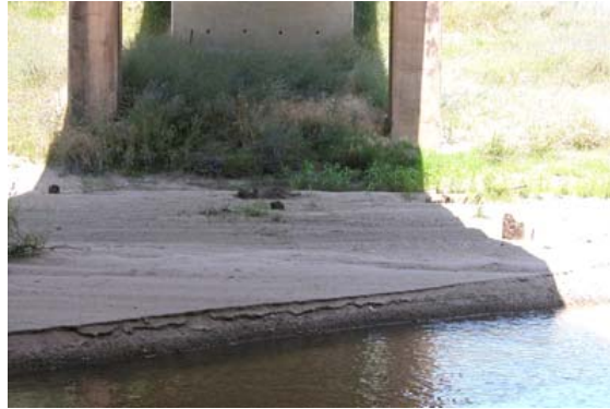
View south under main span showing heads of timber piles used to support falsework for construction
