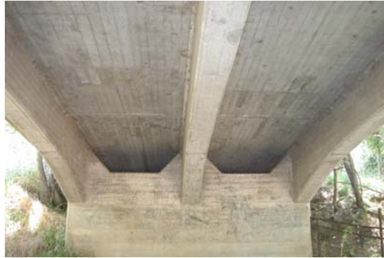
Centreline view under northern approach span with three girders, showing approach slab extending beyond abutment wall
