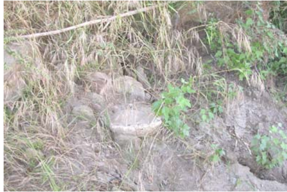
Concrete pad on northern side of creek originally used to support falsework
