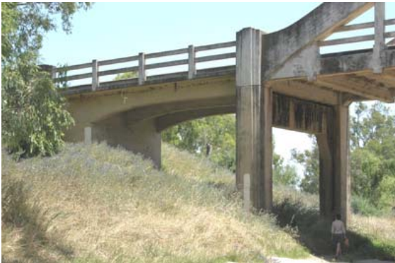
View of southern approach span showing curved soffit to abutment wall with cantilever approach slab behind. Note also the ribbed pier detail
