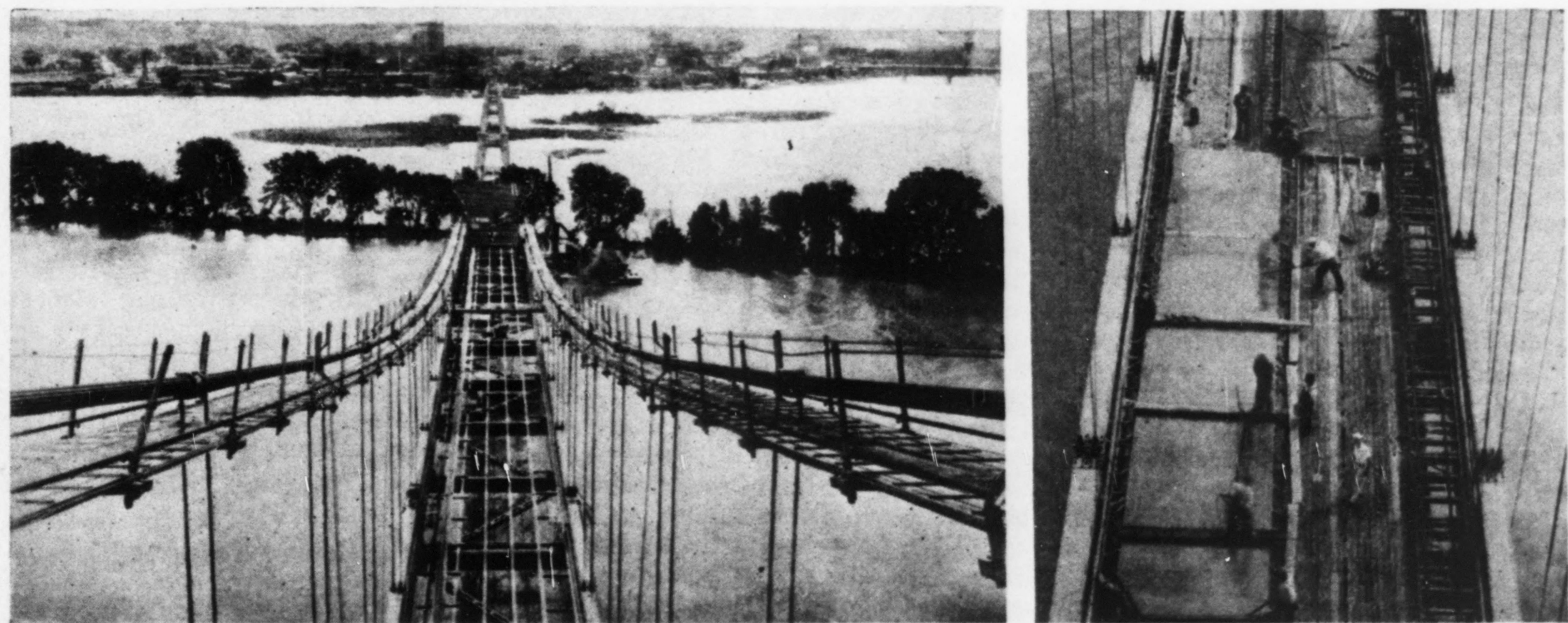
Installing floor steel in toll-collecting area over the island.
