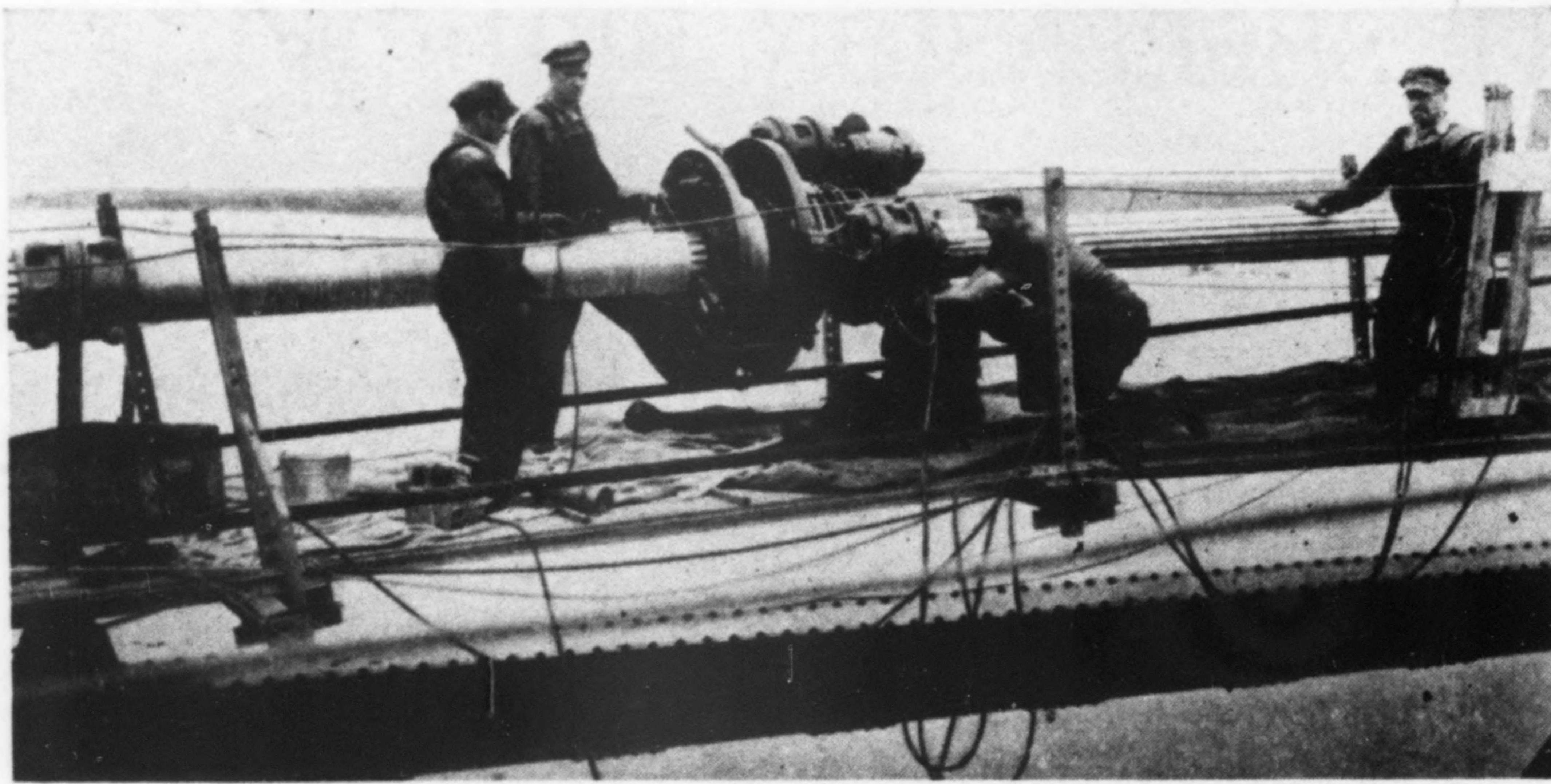
CABLE WRAPPING beginning at center of main span. Aluminum and zinc fillers bring cable to a circular section before wire wrapping is applied.
