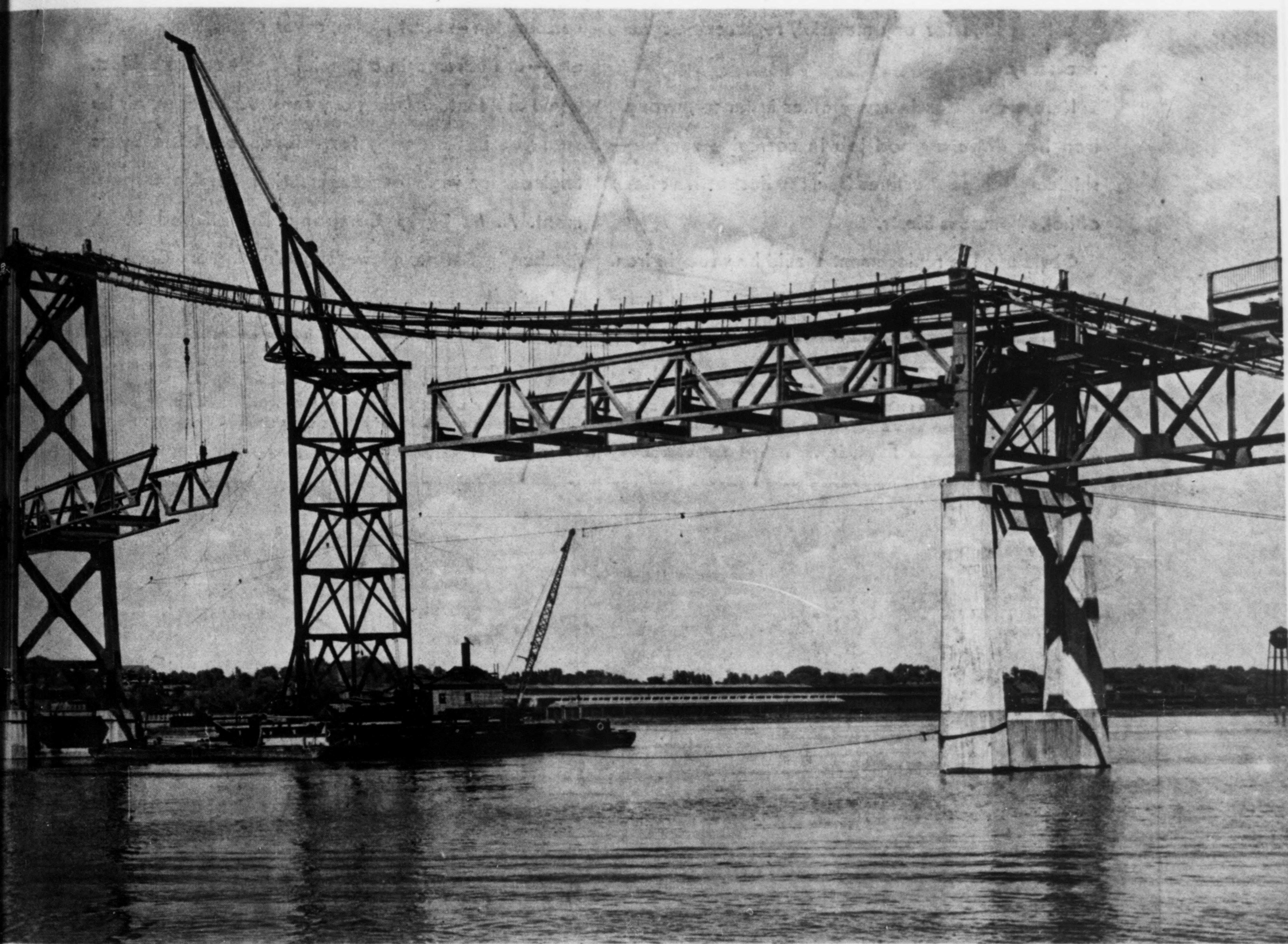
Stiffening truss erection by floating derrick on the Davenport Bridge over the Mississippi River
