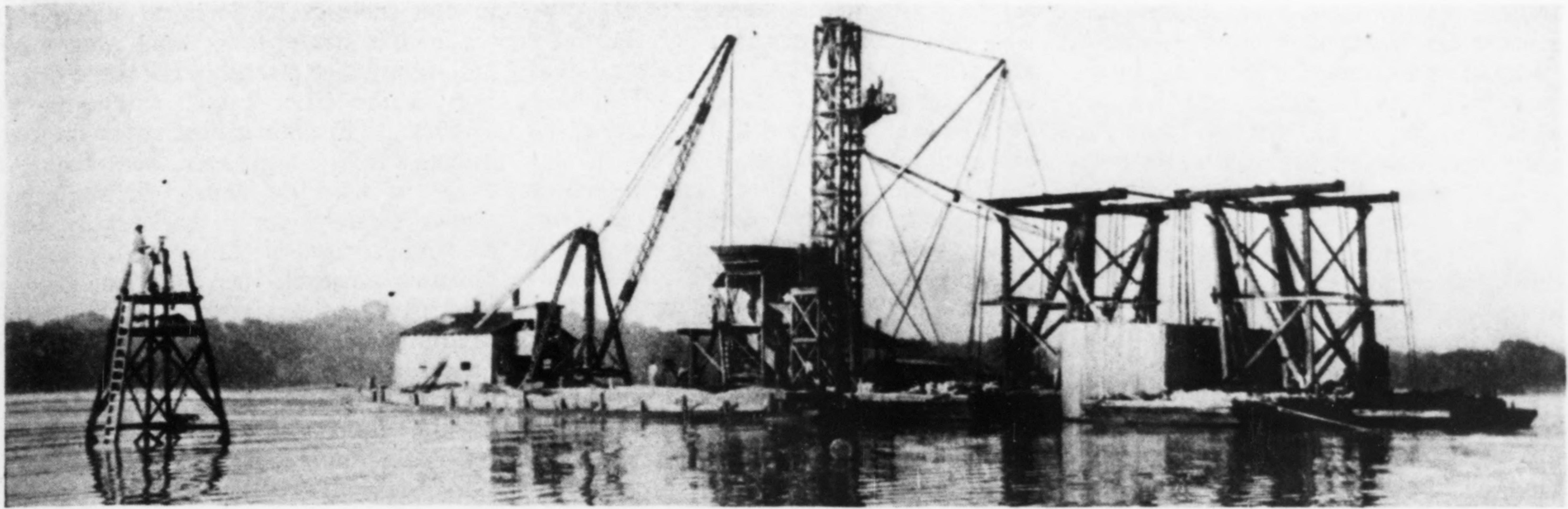
Lowering a caisson with the special headframe device.
