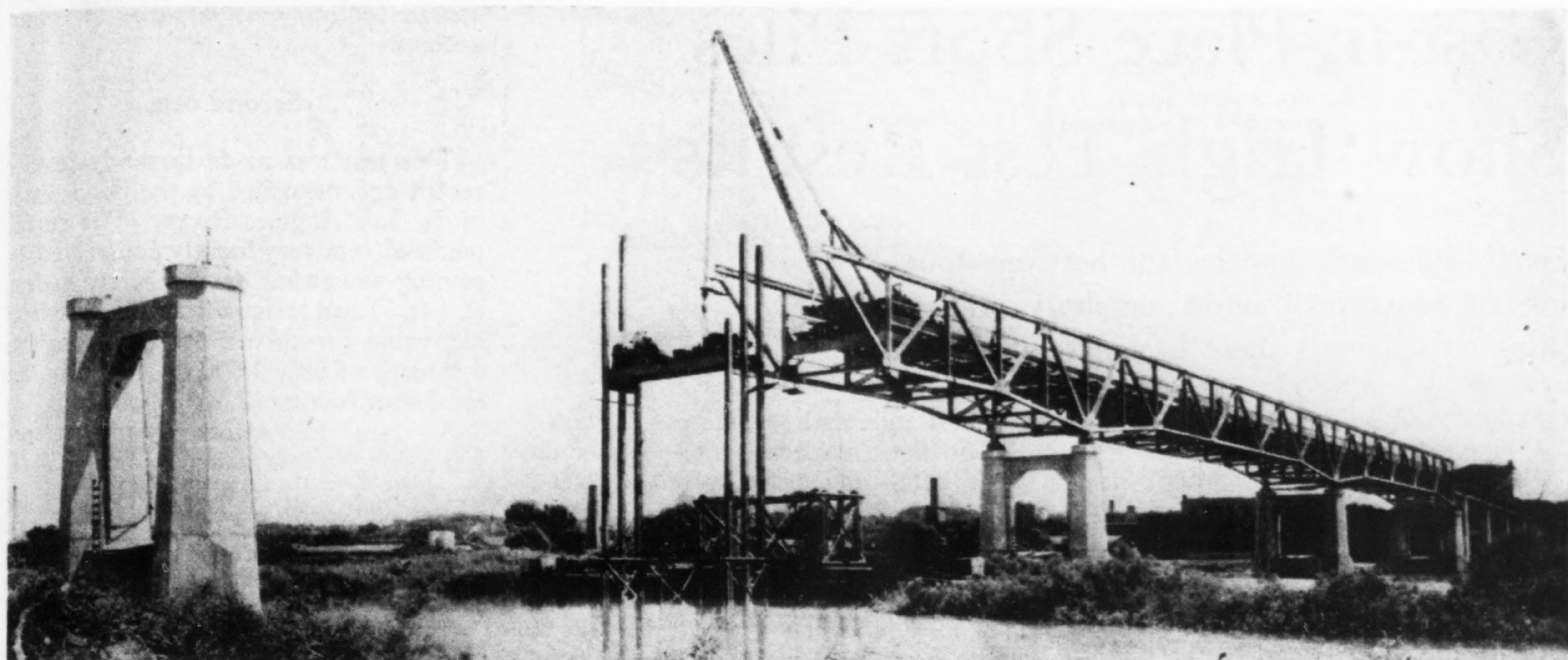
CANTILEVER ERECTION of continuous-truss spans using a falsework bent of six steel H-piles equipped with jacks to lift the span for landing on pier ahead.
