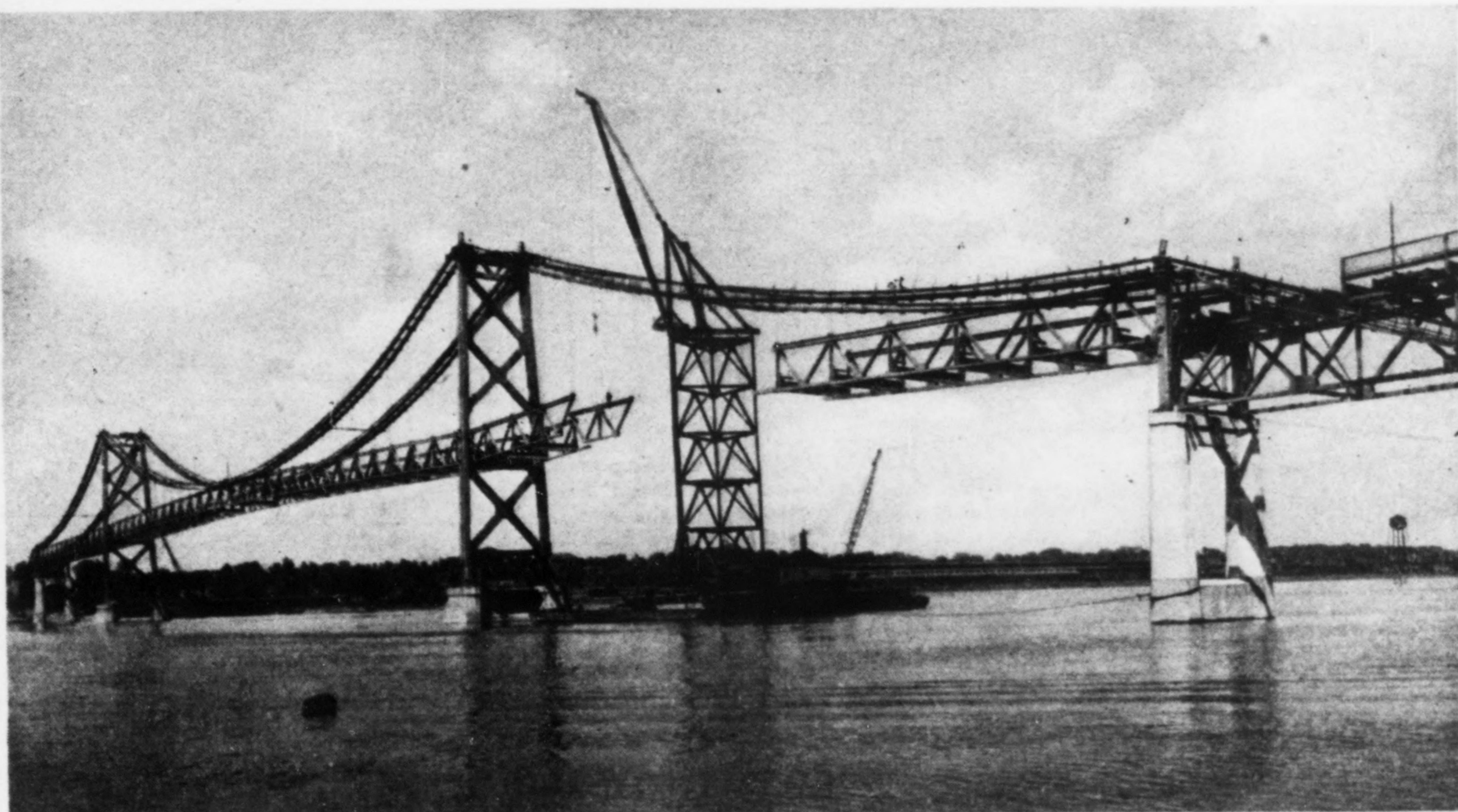
FLOATING TOWER DERRICK hanging stiffening trusses and floor steel on the Davenport Bridge.
