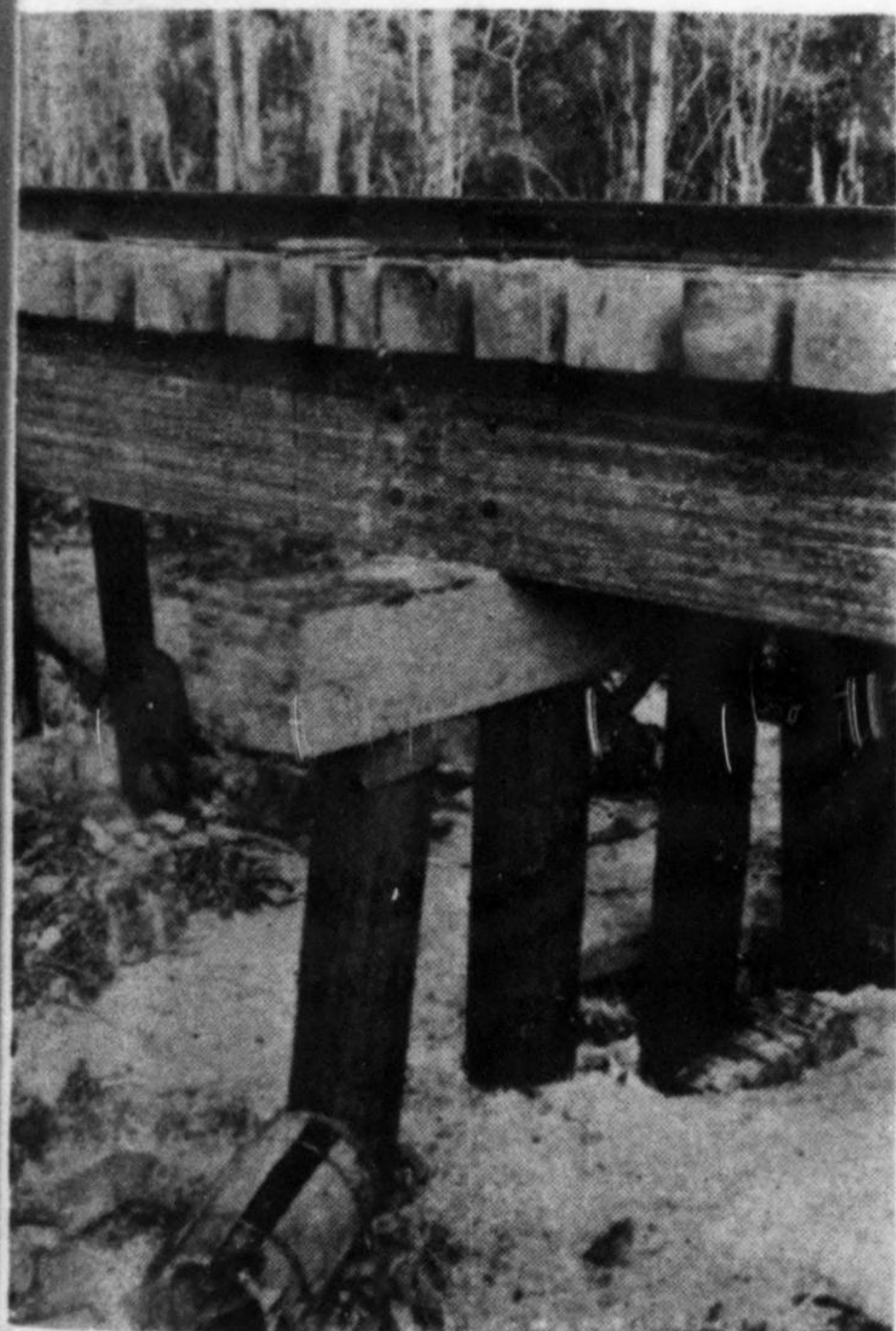
Caps and stringers of this bridge are 1-in. boards glued together. Stringers are 30 ft. long and are spliced over alternate bents of piles, spaced 15 ft. c. to c. A guard-timber spaces and holds the ends of the ties. The structure will support the largest locomotives used on Florida railroads
