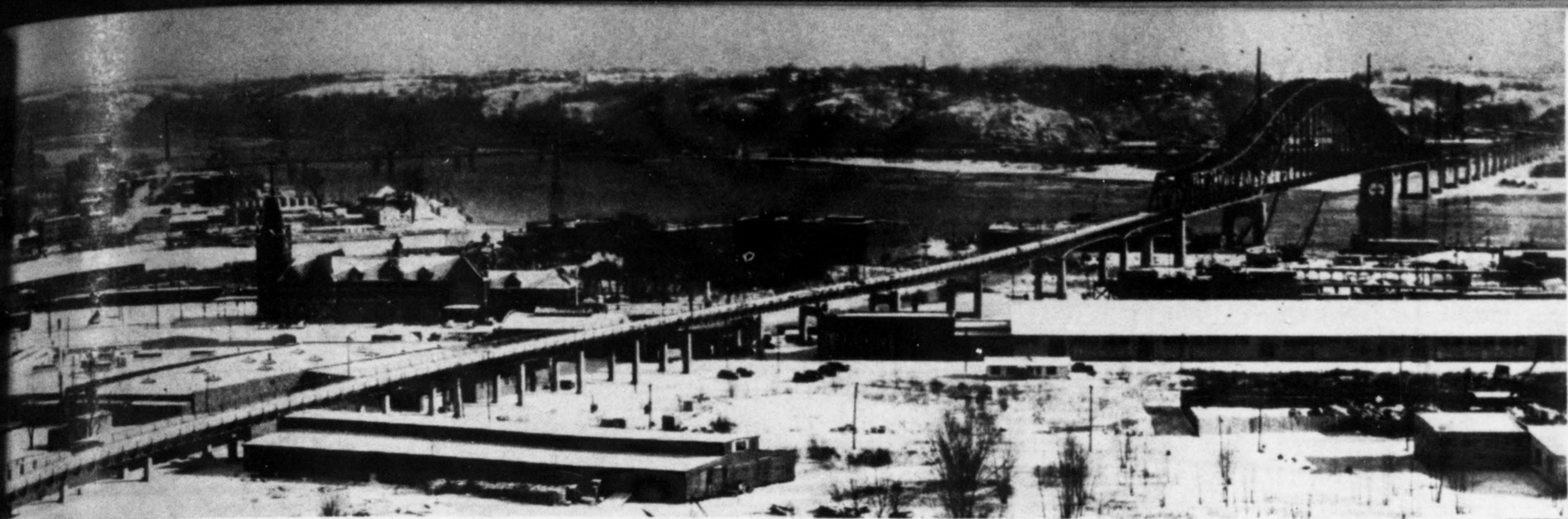
Fig. 2. Flanked by girder approaches, main crossing is a 3-span truss with central span a tied arch. View is from Iowa side.
