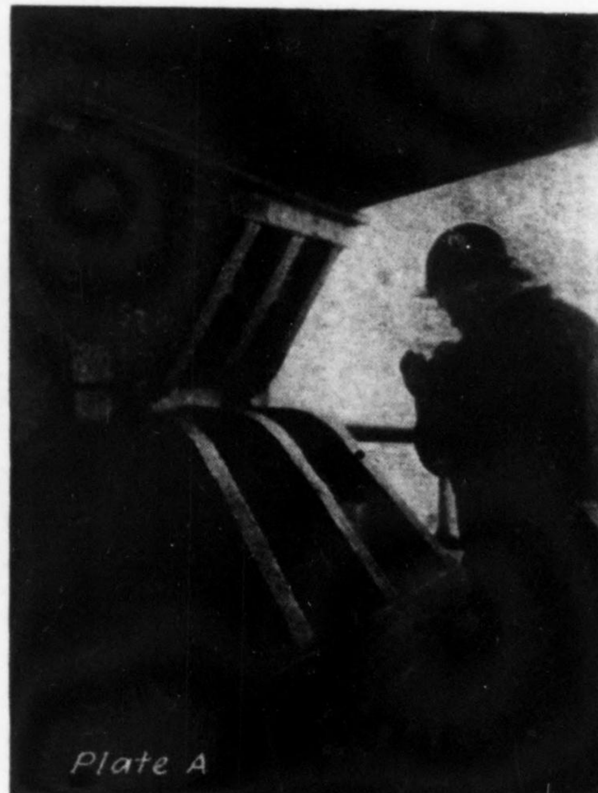
Fig. 5. Below each truss at Piers 18 and 19 shoes of the type above were used. When this picture was taken at Pier 19 that shoe had been frozen by welding to the top of the shoe Plate A, which is bolted to the bearing plate. Later the shoe was made free by cutting away Plate A.
