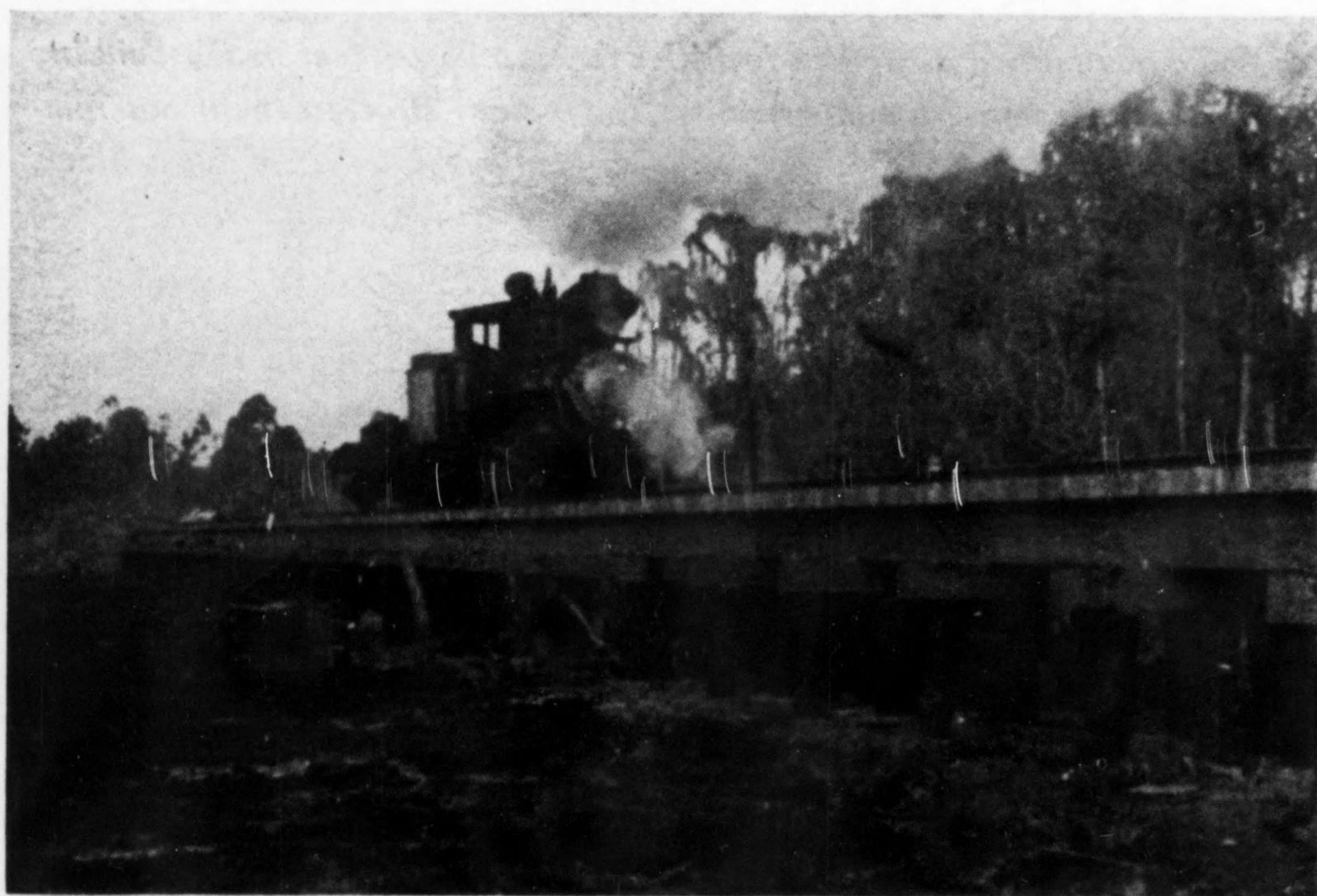
Caps and stringers of this bridge are 1-in. boards glued together. Stringers are 30 ft. long and are spliced over alternate bents of piles, spaced 15 ft. c. to c. A guard-timber spaces and holds the ends of the ties. The structure will support the largest locomotives used on Florida railroads
