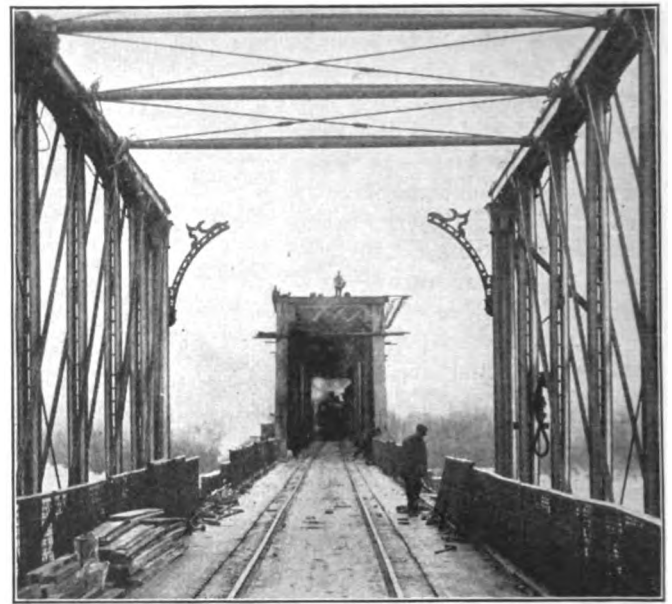
FIG. 5. DISMANTLING ONE OF THE SPANS
