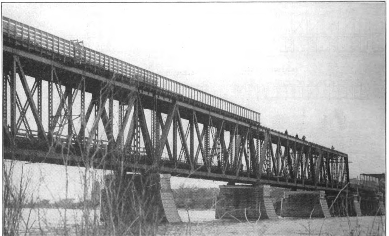
FIG. 6. NEW DOUBLE-DECK SPANS OF THE KEOKUK BRIDGE
