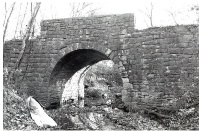
Chicken Creek Bridge. W elevation, E view. October, 1989. KSHS.
