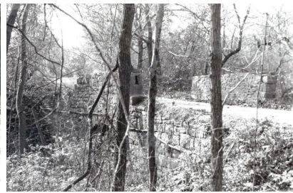
Chicken Creek Bridge. E elevation, SW view. October, 1989. KSHS.
