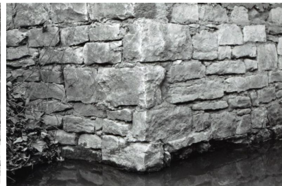
Chicken Creek Bridge. W elevation, NE view. October, 1989. KSHS.
