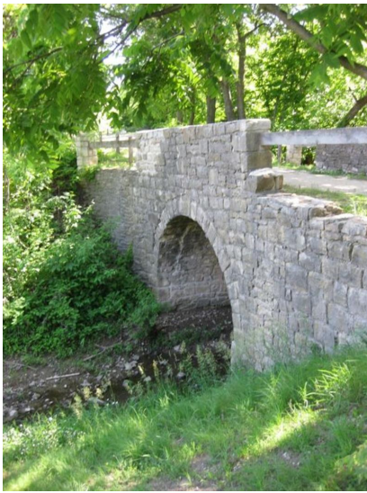
Chicken Creek Bridge. W elevation, NE view. Photo by Andrew Raker.
