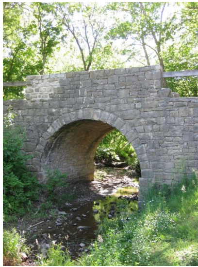
Chicken Creek Bridge. W elevation, E view. Photo by Andrew Raker.
