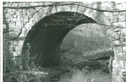
Chicken Creek Bridge. E elevation, SE view. October, 1989. KSHS.
