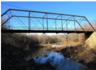
Elk Falls Pratt Truss Bridge. 12/25/2014. Metcalf, Mark.
