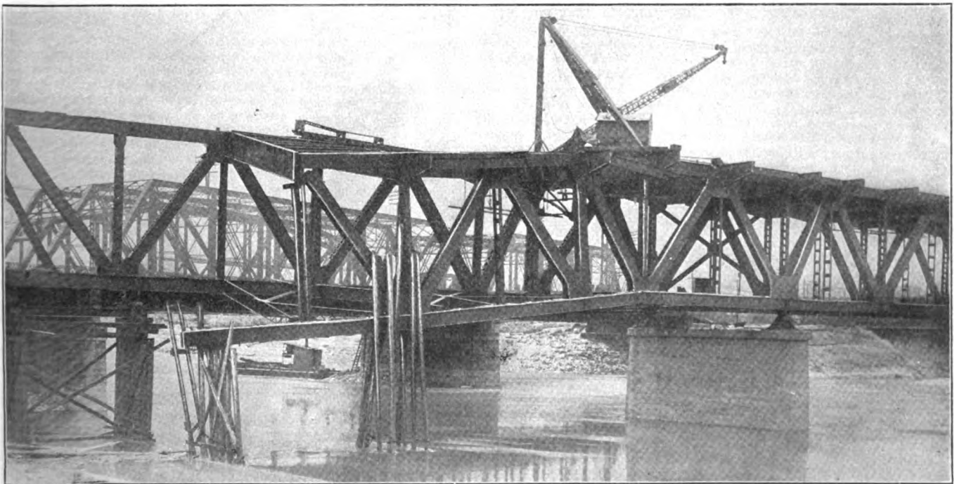
FIG. 2. LOOKING NORTHERLY TOWARD KANSAS AVE. BRIDGE AT KANSAS CITY
