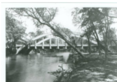
National Avenue Bridge. N National Ave at Marmaton River. Historic Image. 1930s.
