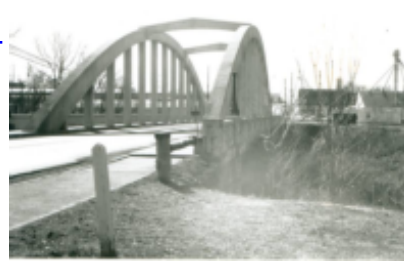
National Avenue Bridge. N National Ave at Marmaton River. JLBanwart, Jr. 2/19/90.
