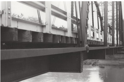
Republican River Pegram Truss Bridge. Bottom Chord Connections. Cloud County. 10/27/1986.
