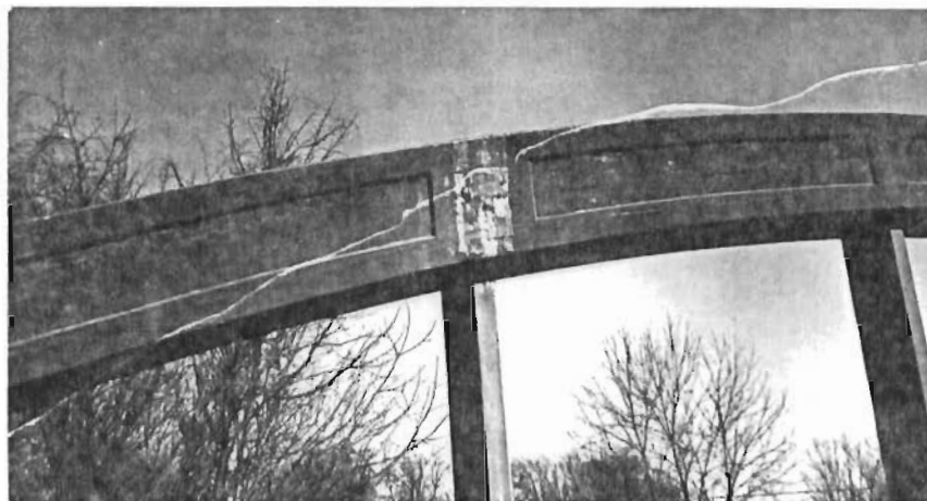
Mine Creek Bridge West arch looking west. Evidence of overhead thru strut removal.
