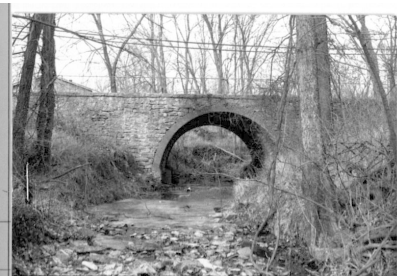
Baldwin-Media Bridge. Winter 1988. Nimz.
