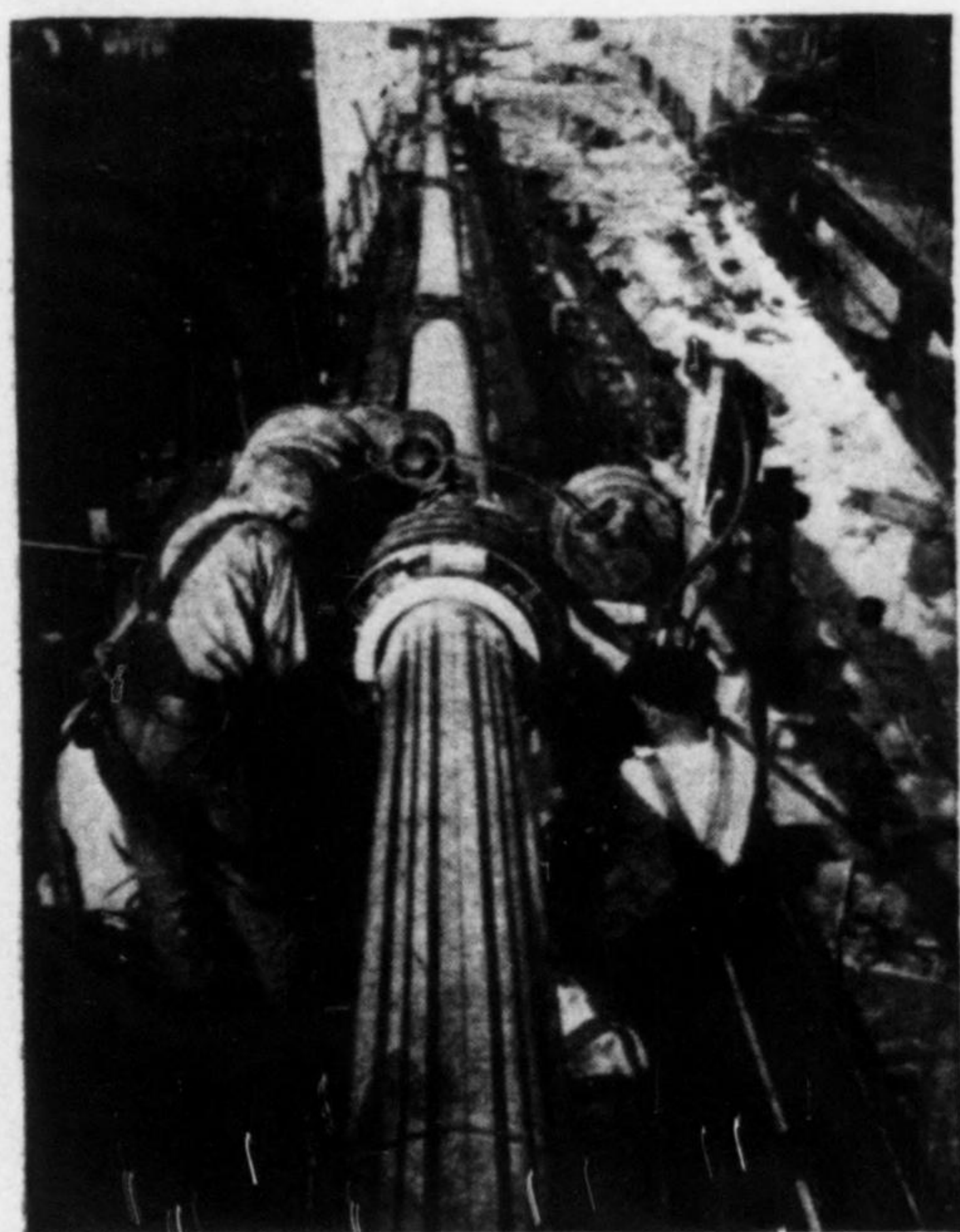
Fig. 9—Wrapping the Maysville strand cable which was brought to a circular section by the use of aluminum fillers.
