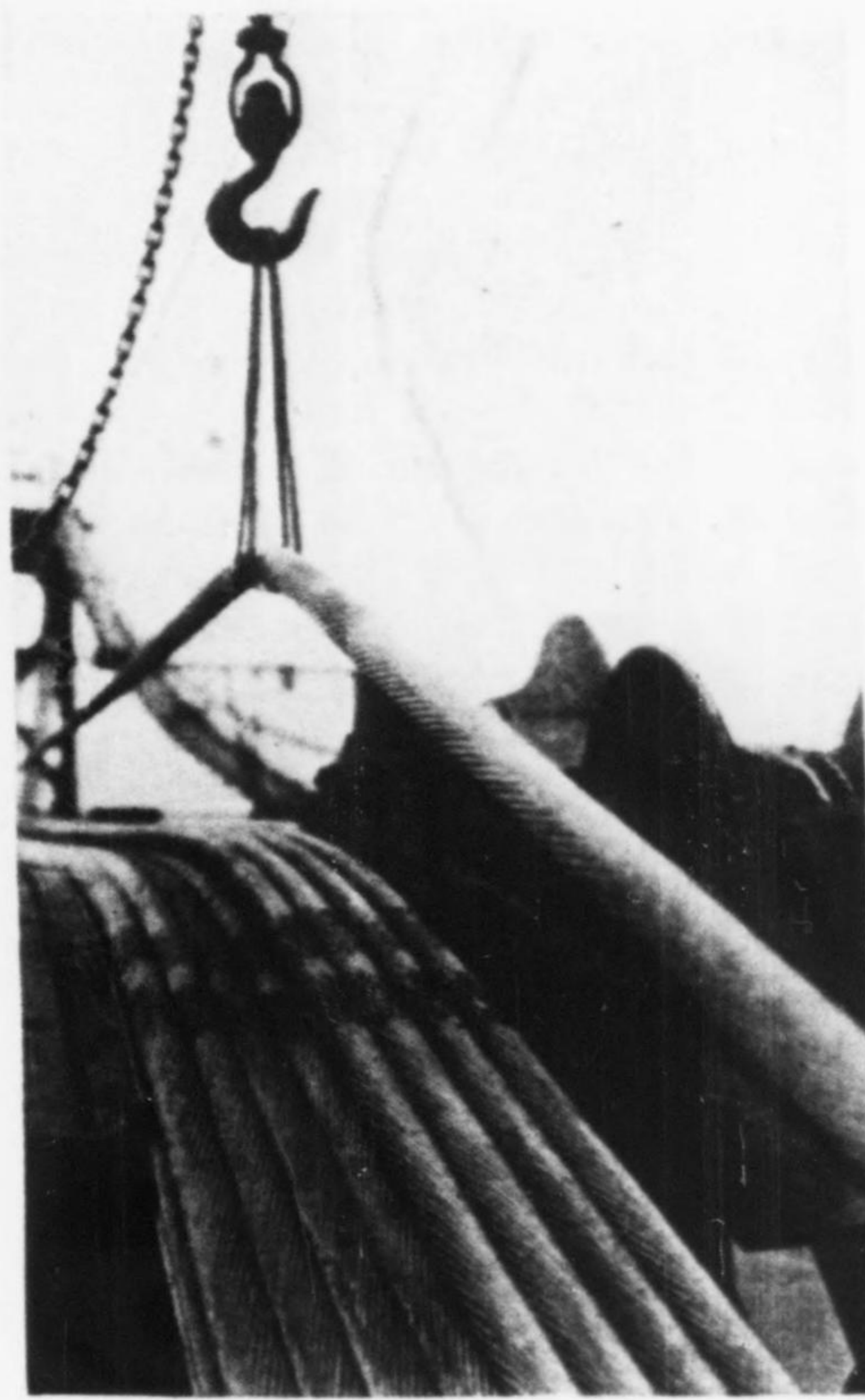
Fig. 8—In constructing the Maysville bridge cable the tramway rope to which strands were connected through a plate and pennant-line (center) was carried at the tower top by a line of deflector sheaves (left). Strands which were supported at the tower tops on four rollers while being hauled across the river were lifted into the saddle by a chain hoist (left and right). In right-hand view note right- and left-lay strands in adjacent layers.
