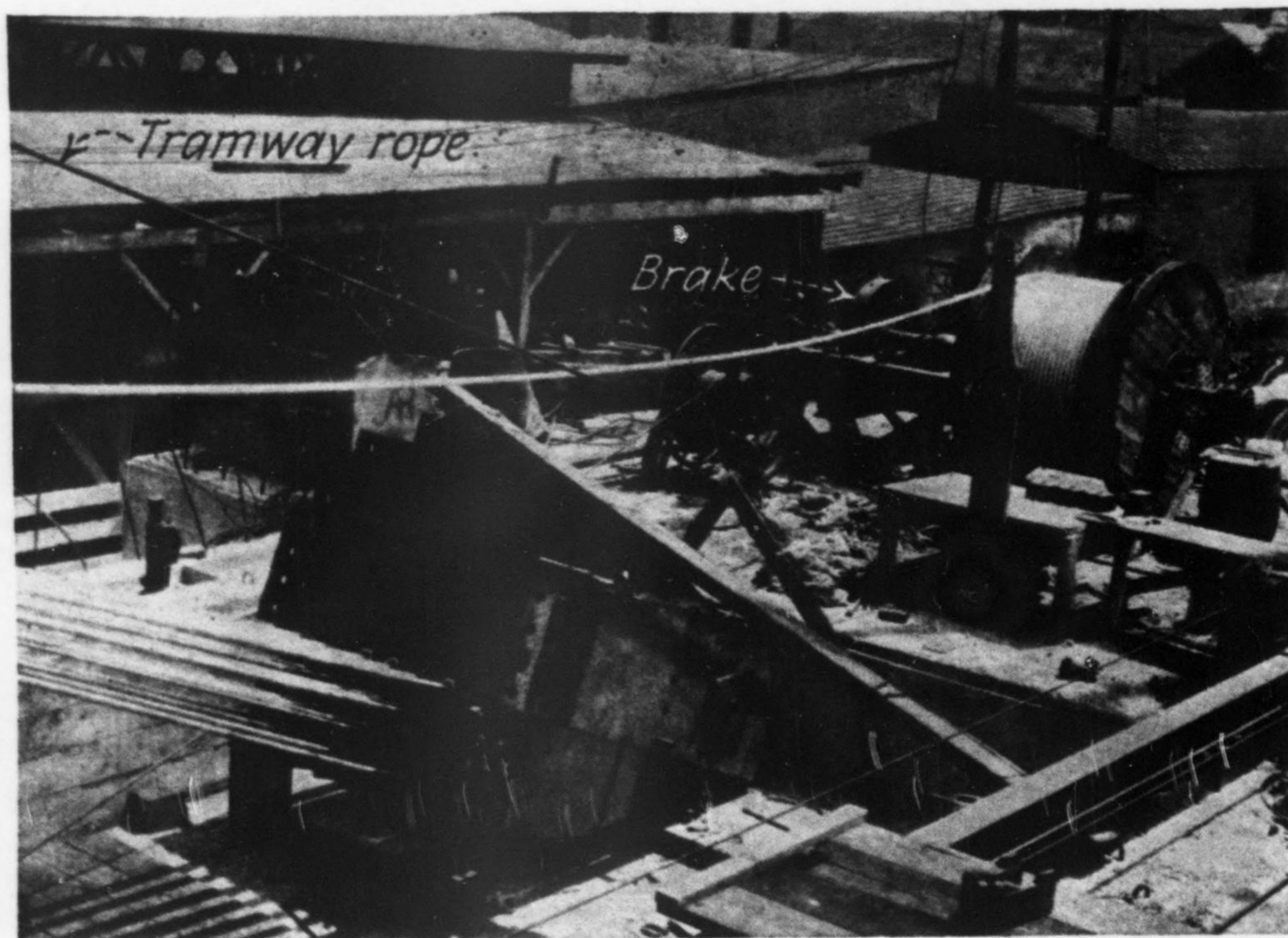
Fig. 7—Cable strands wound on special reels in the field were pulled across the river by an endless tramway rope. Note the compact anchorage requiring a minimum splay of the strands.
