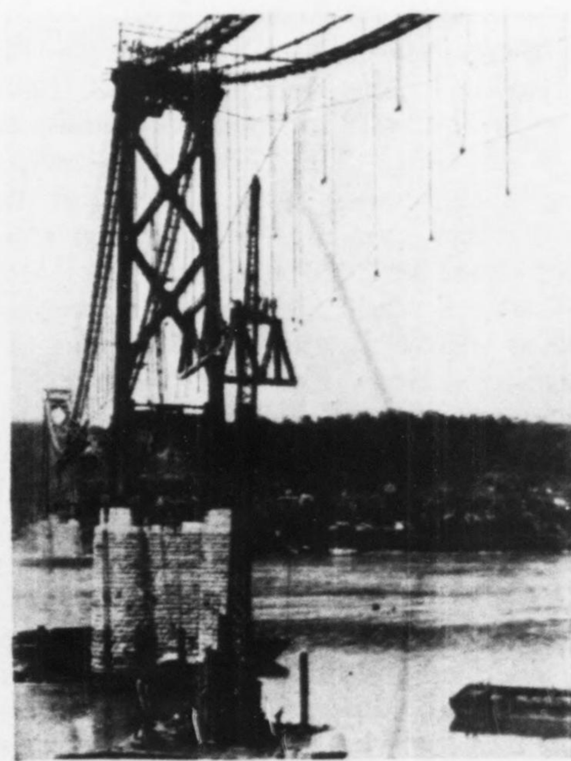
Fig. 10.—Stiffening trusses and floor steel were lifted into place with 130-ft. boom of crane mounted on float.
