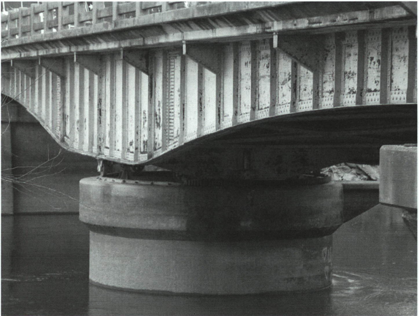
Photo 2: Close-up of center pier and central pivot (photo from TexasFreeway.com)
