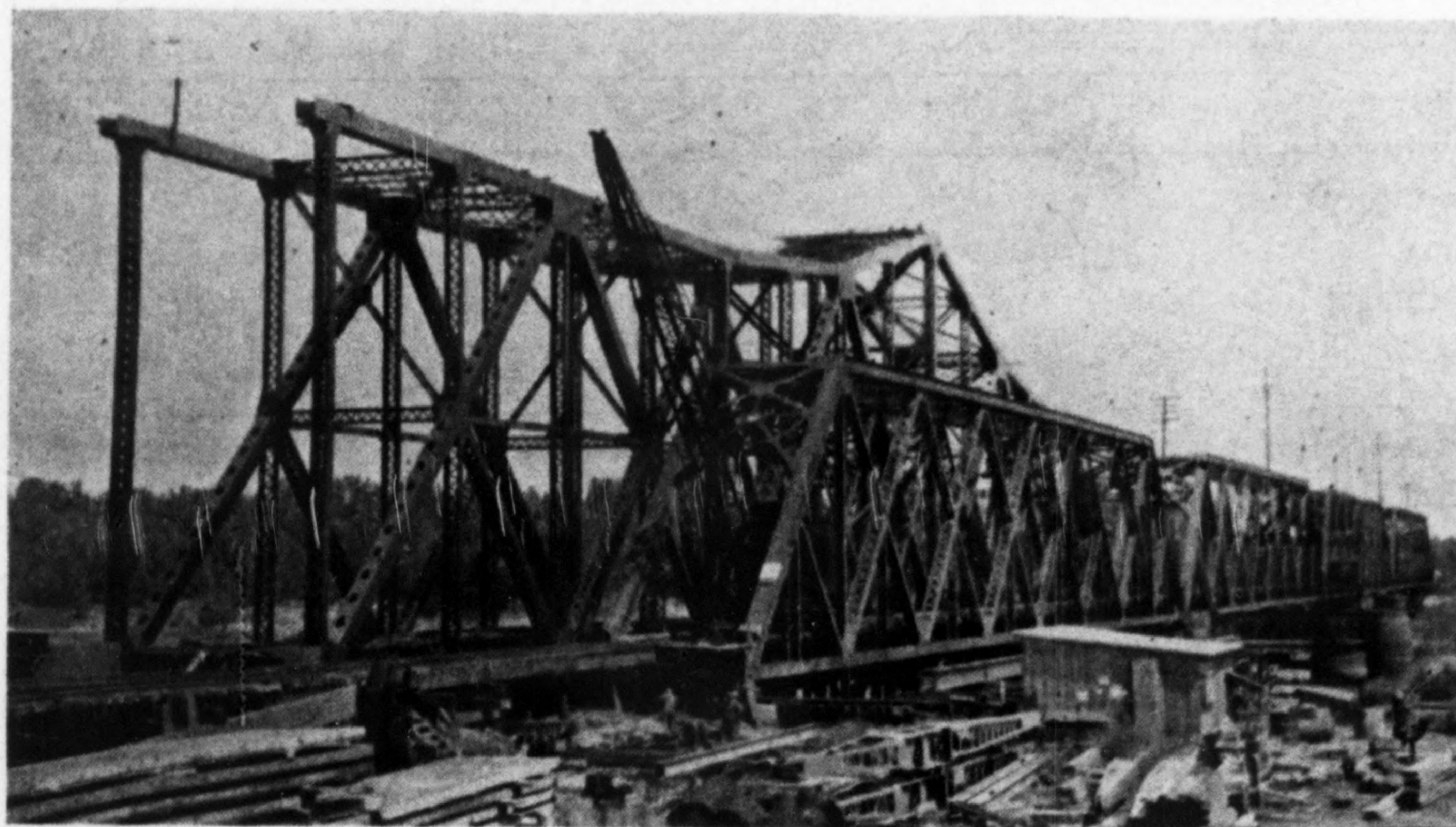
Fig. 4. Ready to roll out the 300 ft. truss span and roll in the new steelwork, which is part of a long span cantilever.
