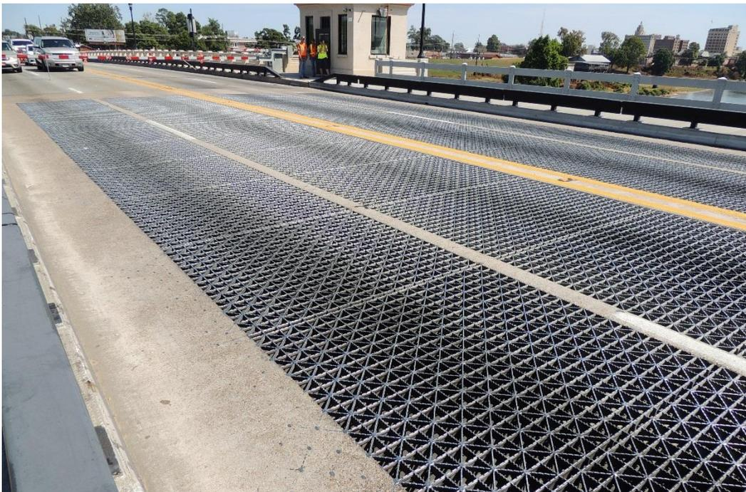
*Condition Photo 16: Steel open grid deck on the bascule span.*
