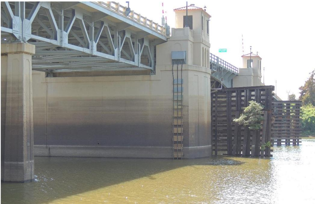
*Condition Photo 28: Pier 5 of the bascule span and vegetation growth in the east timber fender system.*
