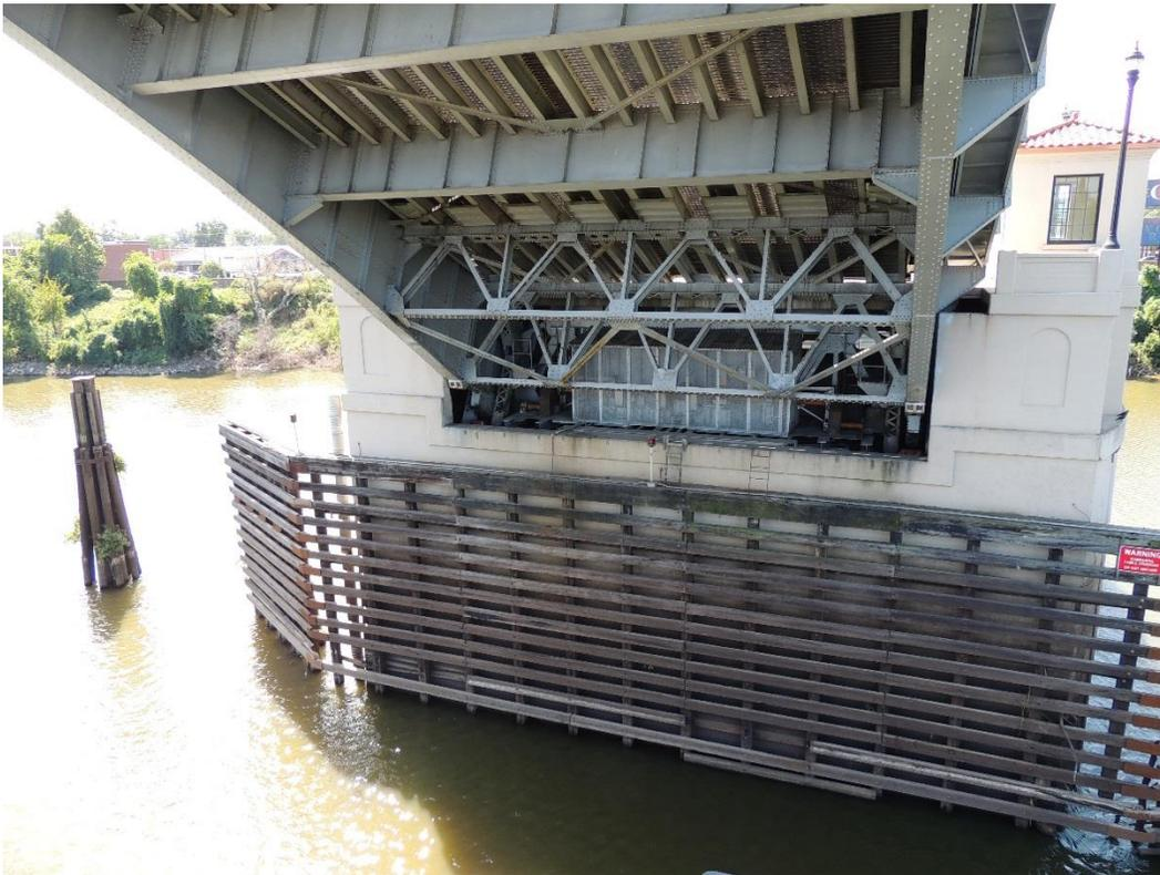
*Condition Photo 30: The west timber fender system, missing members and damaged and the lowering of the bascule span, looking west.*
