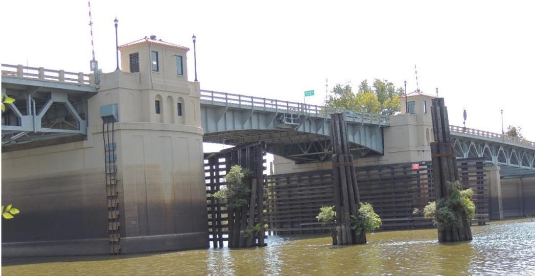
*Character-defining Feature Photo 1: The movable bascule span in the center of the bridge.*
