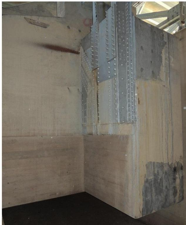
*Condition Photo 8: The counterweight for the bascule span lowering into the pier.*
