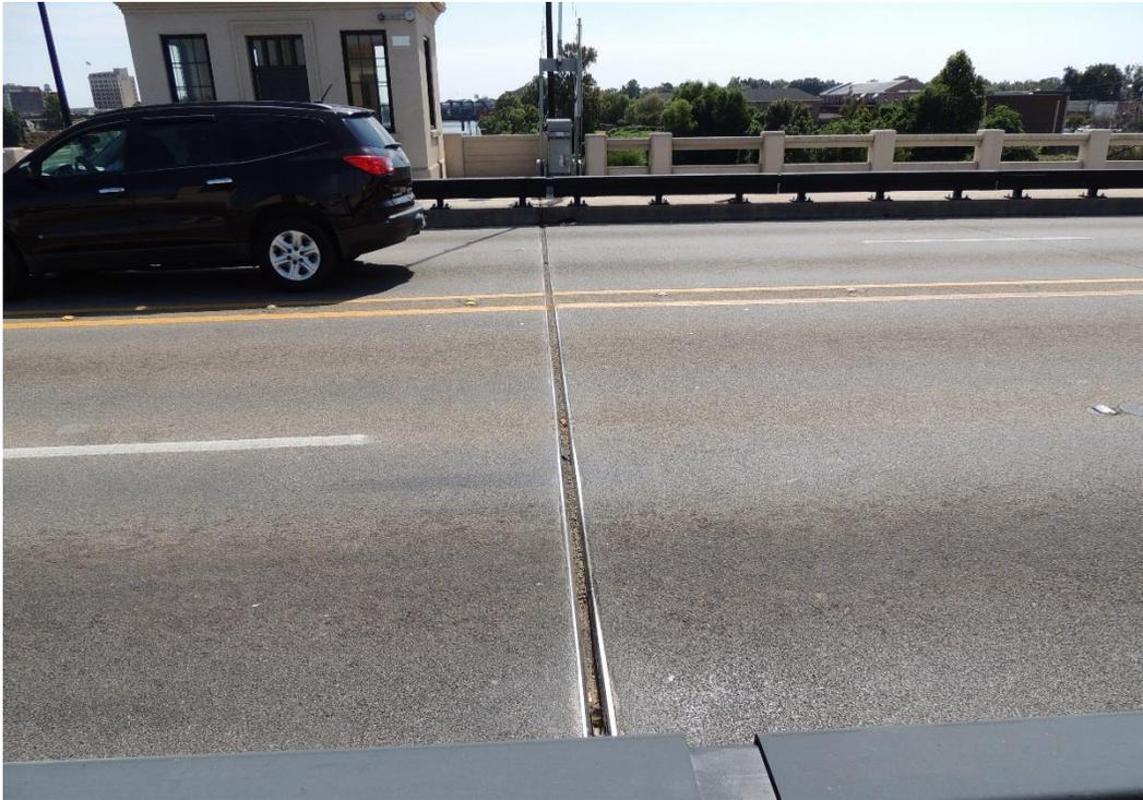
*Condition Photo 13: Pier 4, compression joint full of dirt and debris, typical condition.*
