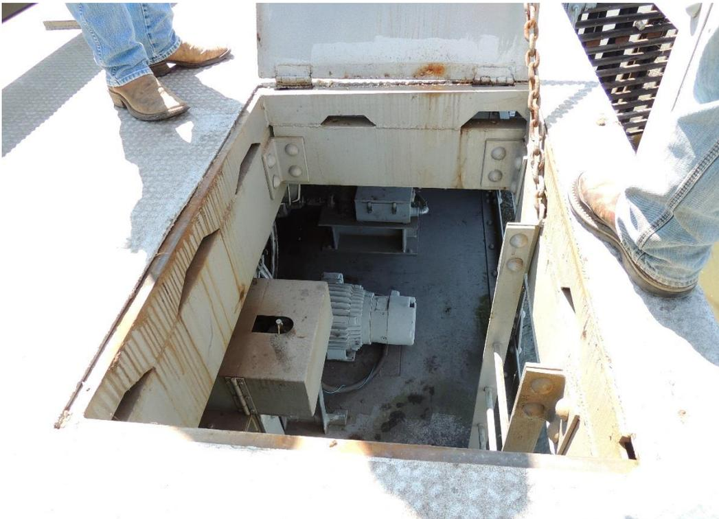
*Condition Photo 18: The gearing and equipment for the locking system for the bascule spans housed under the sidewalk.*
