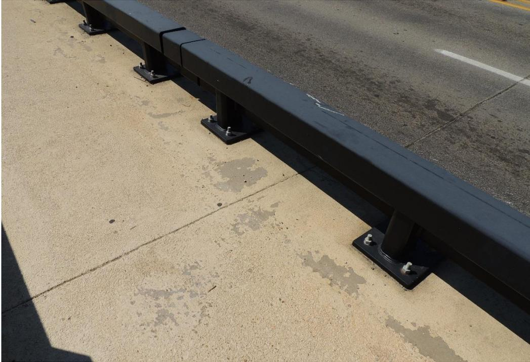
*Condition Photo 17: Vehicular scratches/damage to the metal curb rails on the sidewalk.*
