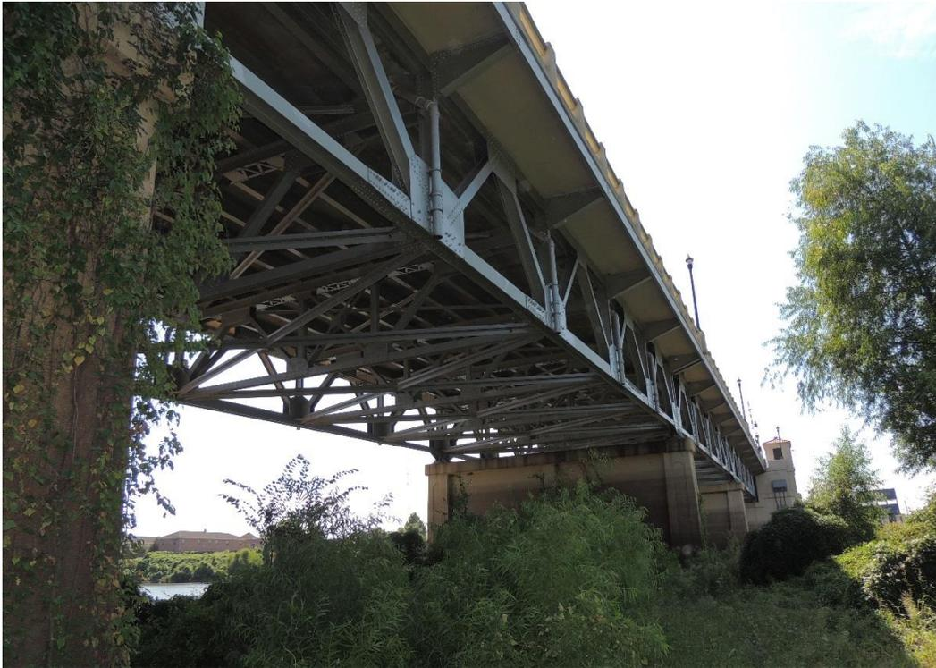
*Condition Photo 25: The underside of the steel truss superstructure approach spans 8 through 10.*
