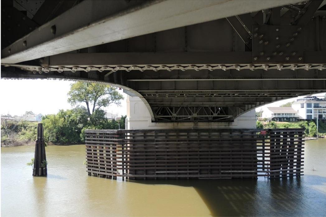
*Condition Photo 29: Typical overview of the west timber fender system.*
