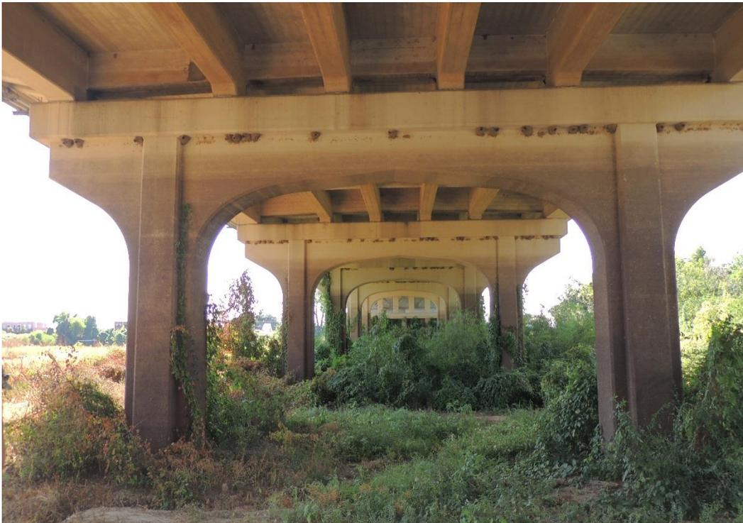
*Condition Photo 24: Vegetation, water staining, and dirt daubers on the substructure units, typical.*
