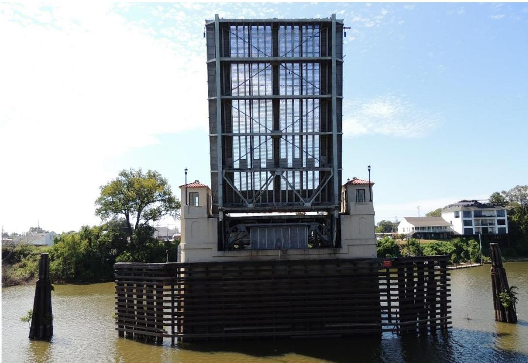
*Character-defining Feature Photo 2: The bascule main span in open position.*
