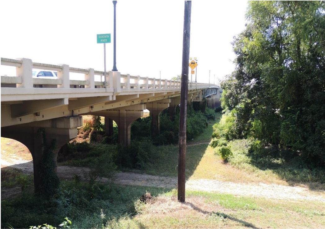
*Condition Photo 23: Approach spans 11 through 18, staining on bents, looking west, typical.*
