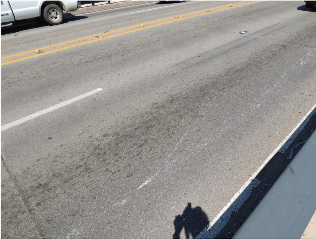
*Condition Photo 15: The concrete deck driving surface, typical condition.*
