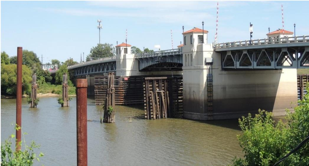
*Historic Fabric Photo 1: Overview of the Lea Joyner Bridge from the northwest bank of the Ouachita River. The bridge's historic fabric includes the two I-beam counterweight spans flanking the bascule span, six steel deck girder spans, and nine concrete approach spans.*
