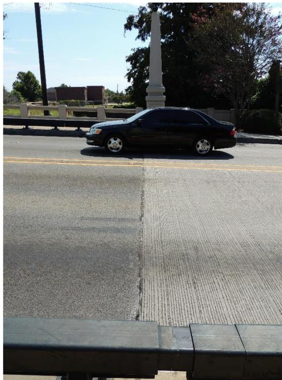
*Condition Photo 12: The relief joint between the approach span 1 and the west approach slab.*
