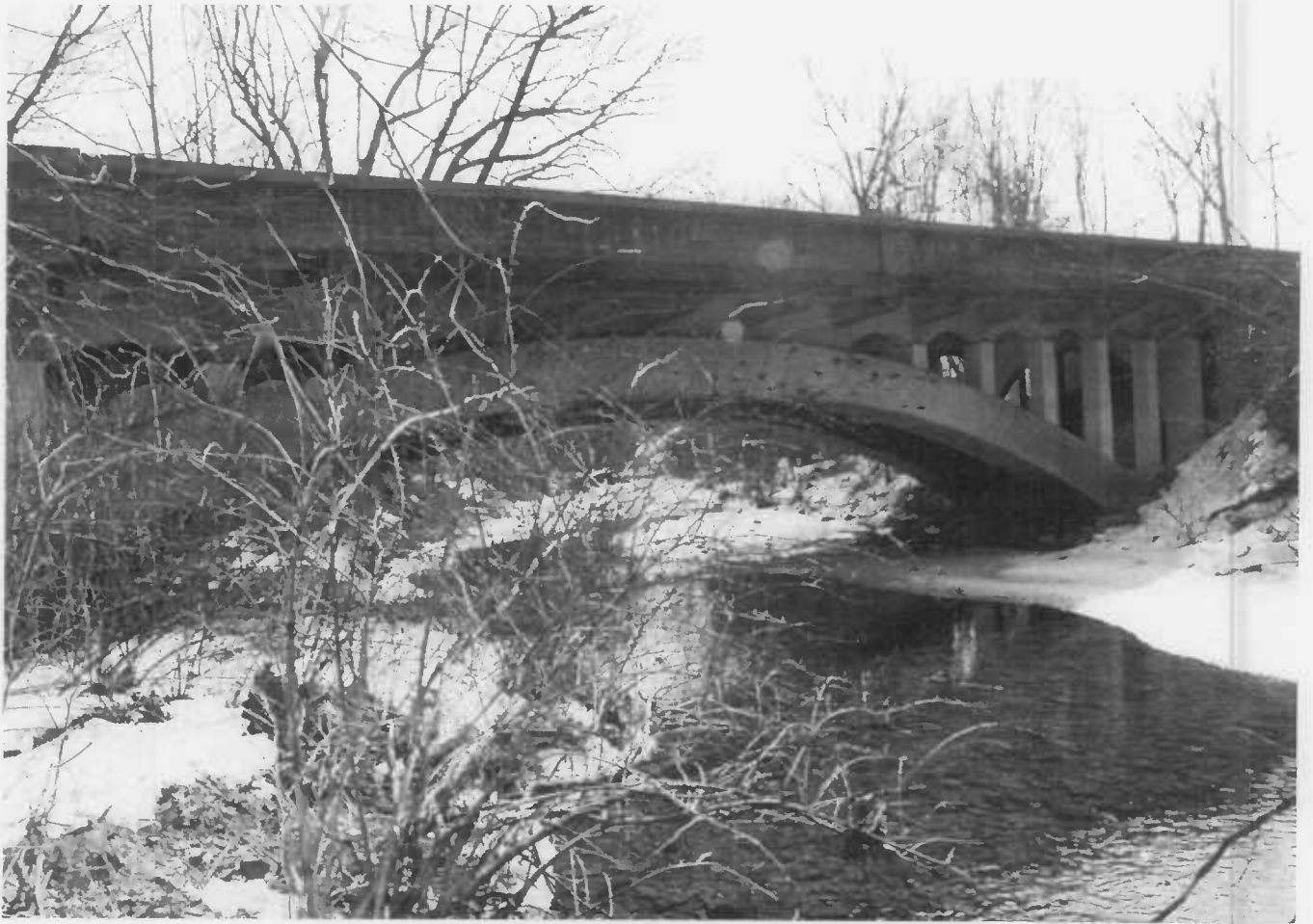
View of SHA Bridge # 1036 (AI-I-83).
